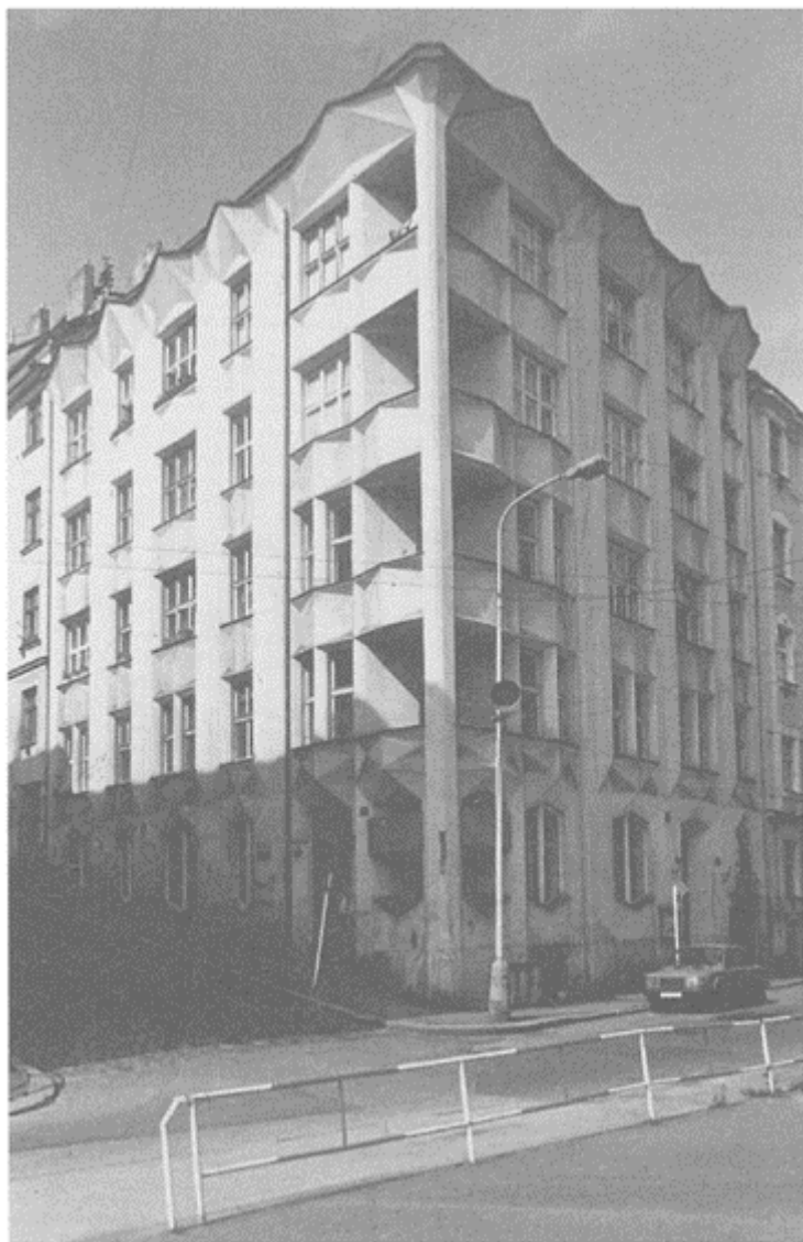
Figure 10.6 Apartment building: Neklanova Street, Vyšehrad, Prague.
