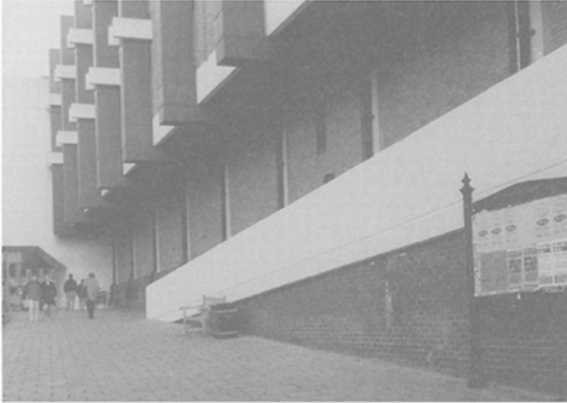
Figure 4.5 The blank exterior of the Westgate Mall.
