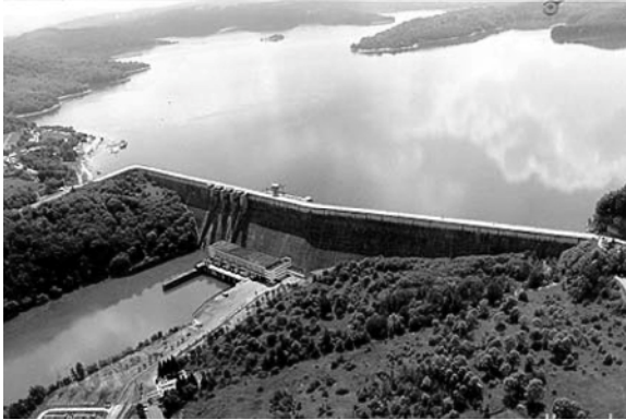
Figure 9.7. Solina power plant [9]
