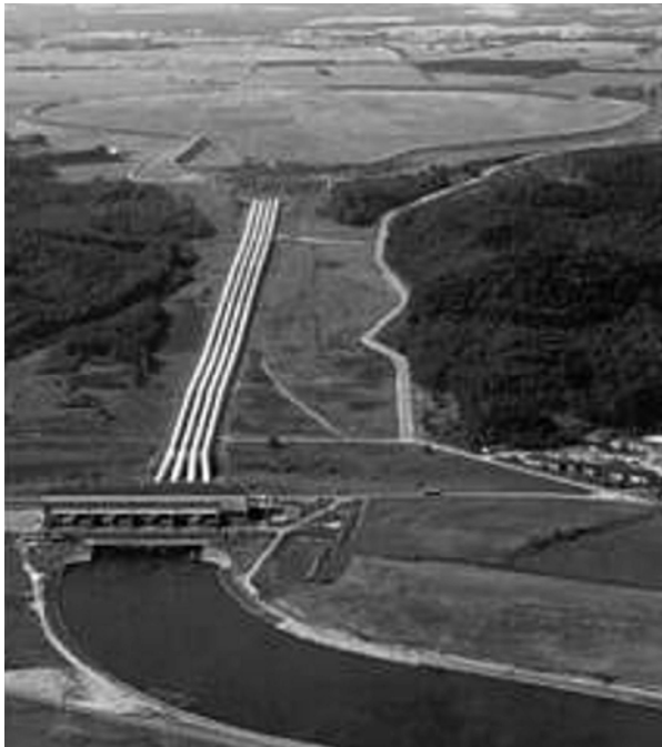
Figure 9.6. View of the Żarnowiec power plant [8]
