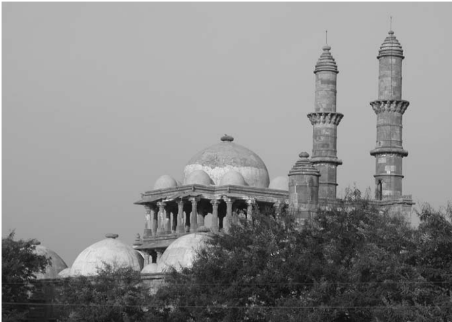
Fig. 5.9 Champaner, Jami Masjid's dome and second-story terrace (photo: Sinah/Ruggles)
