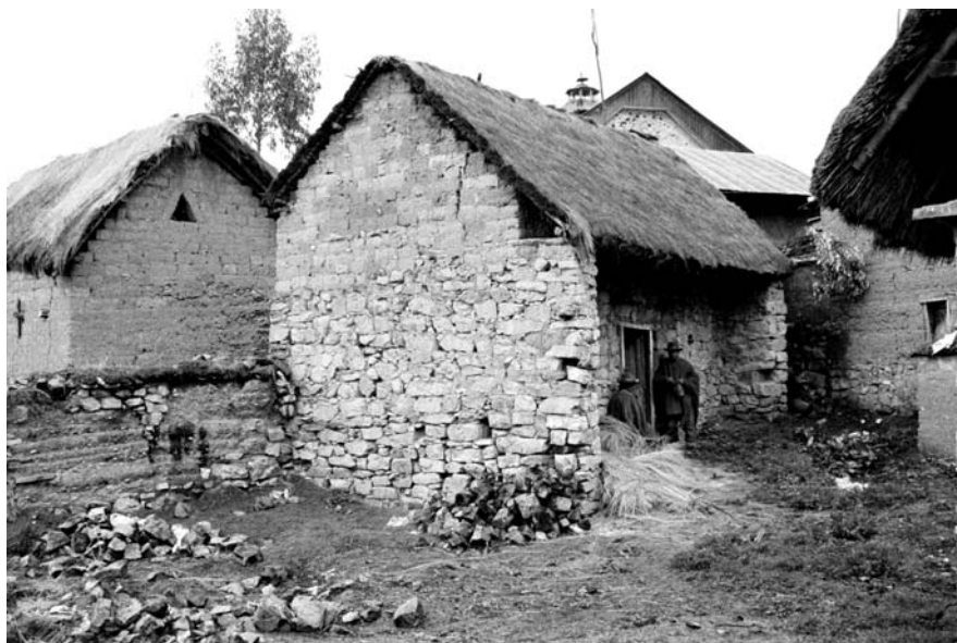
Fig. 6.2 The precinct's Kaha Wayi or "khipu house" before conservation
