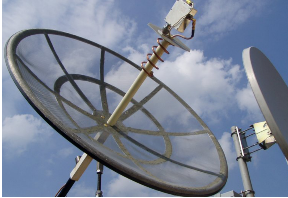
Figure 3.19. Perforated satellite dish
