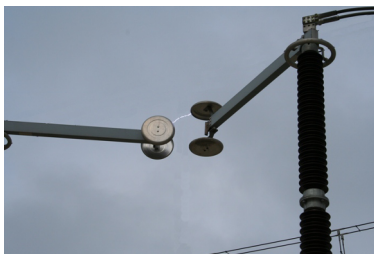
Figure 1.3. Spark gap
