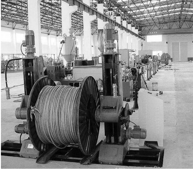
FIGURE 5.11 Conductor paying-off from a drum.
