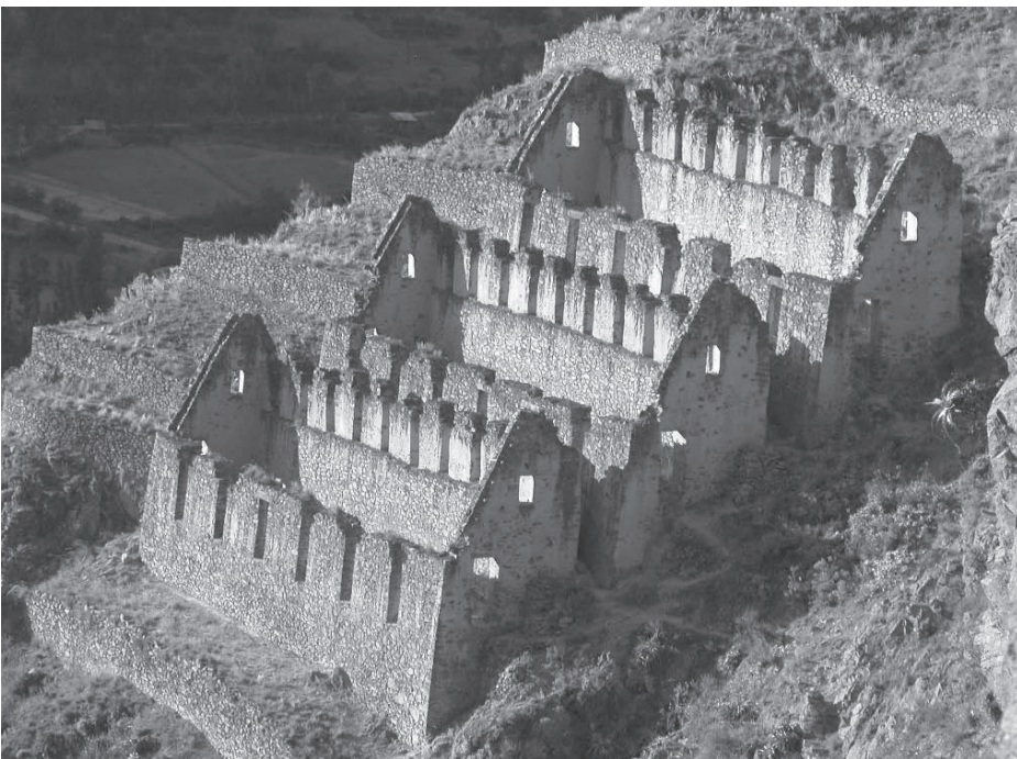
Figure 40.5. A qollqa complex at Ollantaytambo in the imperial heartland. (photo: Catherine Covey).
