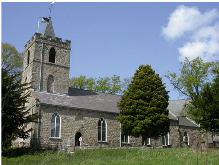
Fig. 10.9 At Blaenavon the ironmasters founded the Anglican St. Peter's Church in 1804 at the heart of the new workers' settlement, complete with cast-iron baptismal font, iron window tracery, sills, and iron heating-flues and surrounded by the cast-iron tombs of the ironmasters and their managers (Crown Copyright RCAHMW)
