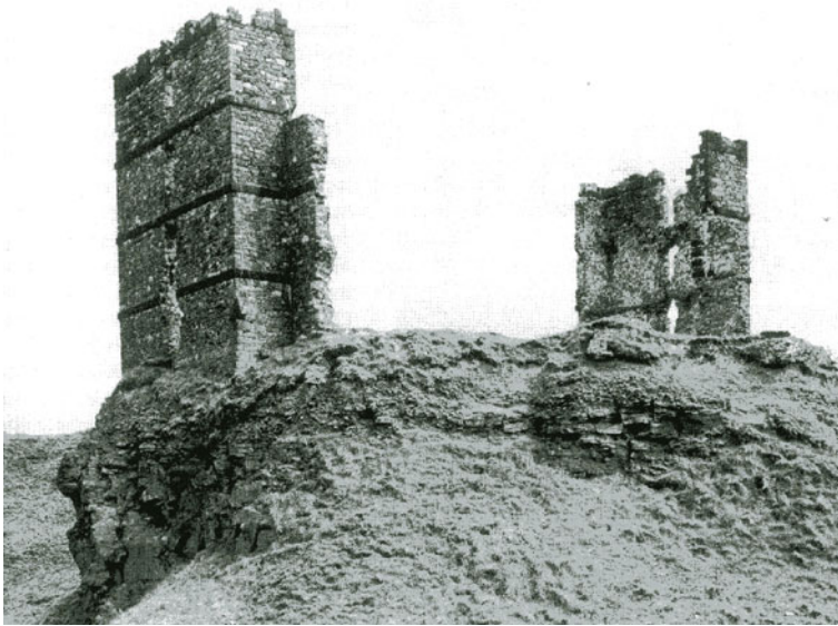
Fig. 10.8 Two of the corner turrets remain from the 1773 hilltop Morris Castle at Swansea, which once housed 24 colliers and their families. It also formed a gleaming white eye-catcher for the nearby Palladian mansion of the Morris family, the coppermasters, who ornamented it with horizontal bands and battlements of glistening black cast copper-slag blocks from their smelting-works (Crown Copyright RCAHMW)
