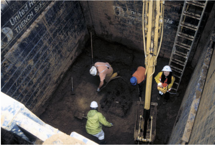
Fig. 3.2 Archaeology in the early twenty-first century (San Francisco, California). Archaeologists target their excavations with surgical precision; use heavy equipment, air monitors, elaborate health and safety plans; cope with looters, unreliable security firms, and the displaced homeless; they must have HAZMAT training, wear hardhats, safety vests, and protective clothing (Photo courtesy Anthropological Studies Center, Sonoma State University)
