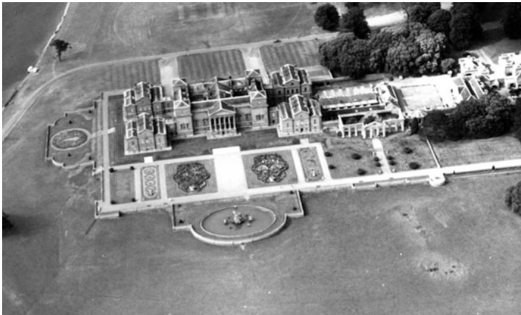
Fig. 2.3 Holkham Hall, Norfolk. When completed in the middle of the eighteenth century, the hall was set within an open, “naturalistic” landscape. In the mid-nineteenth century, in keeping with the prevailing fashion, it was provided with a more formal and architectural setting—geometric gardens and substantial terraces—designed by William Andrews Nesfield
