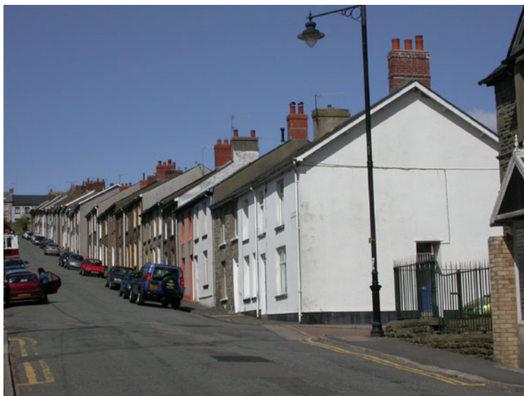
Fig. 10.6 The present township of Blaenavon was built in three components, the first a partly planned company township, the second a partly self-built and speculative worker's town, and the third another planned grid (1864–1866), pictured here constructed as the iron-making company diversified into coal sales (Crown Copyright RCAHMW)
