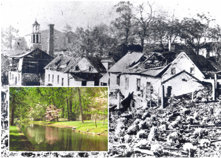
Fig. 1.3 A serene Brandywine River meanders through the former du Pont gunpowder works at Hagley Museum, inset over an image of the aftermath of a devastating gunpowder explosion in the upper yard of the powder works, 1890 (Photo courtesy of Hagley Museum and Library)
