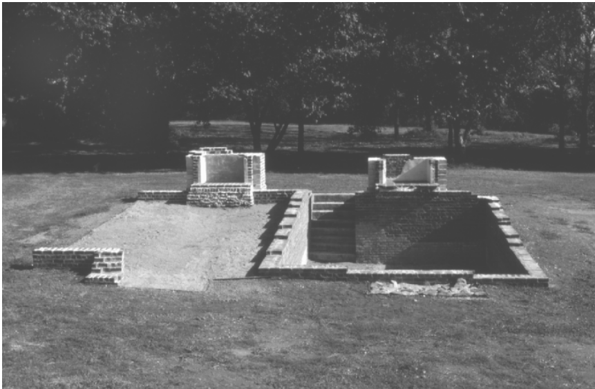
FIGURE 2.1. The stabilized and partially rebuilt brick foundations, chimneys, and cellar of the ca. 1740 Tolle-Tabbs house. (Courtesy of Historic St. Mary's City)
