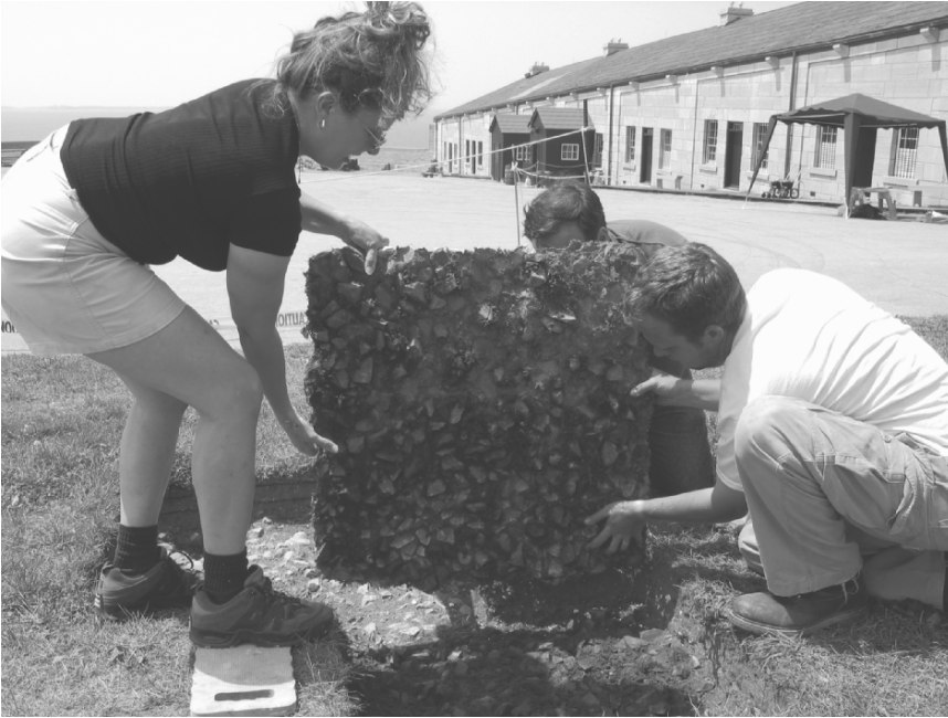
FIGURE 22.2. Lifting the latex mould of the macadamized parade surface at Fort Henry in preparation for a resin cast of the landscape feature. (Photo by J. Last. Parks Canada, Ontario Service Centre (Cornwall), photo no. 131H0107E.)
