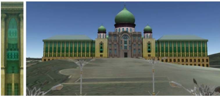
Fig. 17 Using higher exposure settings to represent raised geometry for Putrajaya Prime Minister Department
