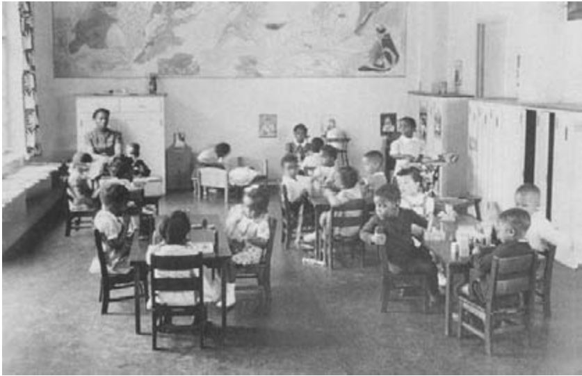
FIG. 6.5 A nursery school at Harlem River Houses. This photograph shows a class from 1938. As at the Mackley Houses, the nursery school was one of the most successful aspects of the development, functioning to integrate adults into the community as well as providing a service for children.
