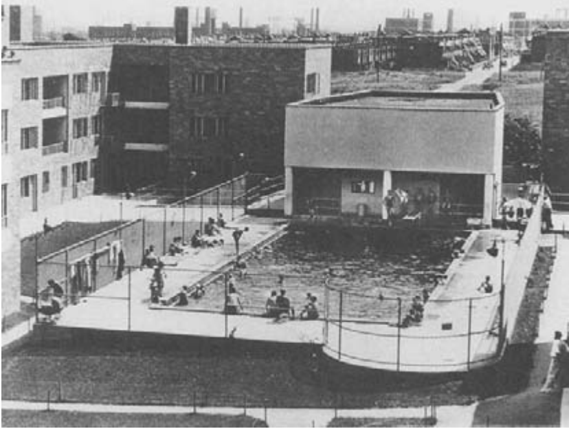
FIG. 5.5 The pool and community hall at the Carl Mackley Houses. In the background, one can see the dense rowhouse pattern of development that was filling up this working-class section of Philadelphia. (The empty areas in the photograph have now been filled in with the same kind of housing.) The community facilities, while built on a less lavish budget than those in Moorestown (shown in figure 2.6), were well regarded and heavily used by residents. Reproduced courtesy of the Historical Society of Pennsylvania.
