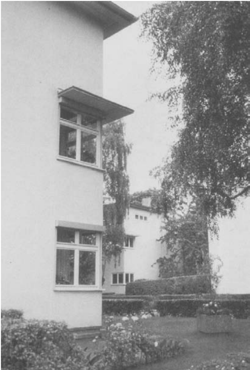
FIG. 3.3 Small apartment houses and grounds built in Frankfurt, Germany, in the 1920s. This photograph, taken in 1990, shows how the precise geometric shapes and plain (often white) exterior walls characteristic of modernistic rationalism complement the lush gardening for which the Germans are famous. This strand of architectural modernism eventually won out over competing tendencies throughout the world and became known as the "International Style," in good part because its simple rectangular forms lent themselves to economies of production. Rationalism's proponents, however, prized it not merely or even chiefly for its utilitarian qualities, but rather for the abstract beauty of its forms and its connection to utopian social ideals.
