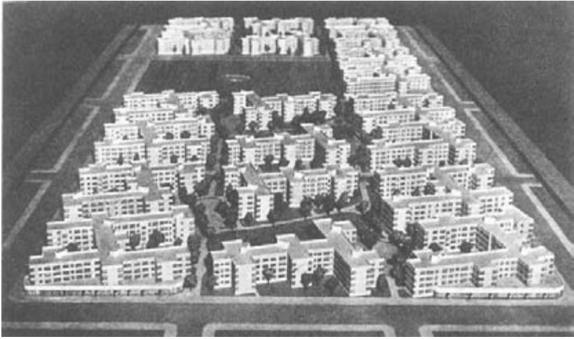
FIG. 6.4 Architect's model of the Williamsburg Houses in Brooklyn, designed by William Lescaze. This was Harlem River's sister project, intended for white residents. The off-grid parallel design is superficially reminiscent of Zeilenbau style but did not provide its practical advantages. The prevailing winds in this area turned the courts into wind tunnels, and many of the rooms were not properly oriented for receiving good sunlight. The Carl Mackley Houses, though they had a more traditional appearance and fit into their environment more comfortably, did provide many of the advantages of Zeilenbau planning. The Harlem River Houses looked like commercial New York apartment buildings of the era, but they were designed on superblocks containing extensive landscaped grounds (a core modern housing idea). AP/Wide World Photos.
