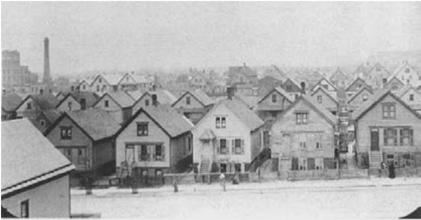
FIG. 1.1 This Chicago neighborhood of small wooden homes was actually more typical of inexpensive urban housing in the late-nineteenth-century American cities than the famous tenement houses of New York City. Initially, such structures were often little more than drafty shells, with only stoves for heat and no running water or indoor toilets. While they appear to be single-family dwellings, they were routinely divided between two or more families. Their deficiencies as individual units could be significantly rectified over time, however, as owners invested money and their own labor in upgrades of various kinds. A more problematic outcome of the housing delivery system of this era was the monotony and density of the larger neighborhood environment, with few landscaped open spaces available for visual relief or recreation. Photograph reproduced courtesy of the Chicago Historical Society.
