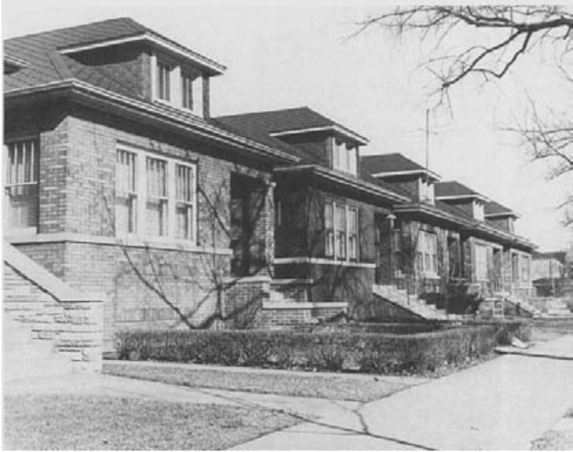
FIG. 1.4 Streetscape of Chicago bungalows constructed in the 1920s. Built of brick and provided with indoor plumbing, electricity, and central heating, these homes were significantly more comfortable than the crude wooden residences of previous decades. Nevertheless, methods of subdividing continued to result in long narrow lots. Thus, bungalows were quite long and usually set close to the property lines on their sides, an arrangement that compromised possibilities for interior sunlight as well as pleasant views from windows. Furthermore, although these houses were some of the least expensive built in the 1920s, they still cost much more than the entry-level homes of previous decades and were not easily affordable for people of modest incomes. Photograph: Bungalows on 9100 block of South Colfax Avenue, Chicago, Illinois, 1962; photographed by Ralph E. Tower. Reproduced courtesy of the Chicago Historical Society.
