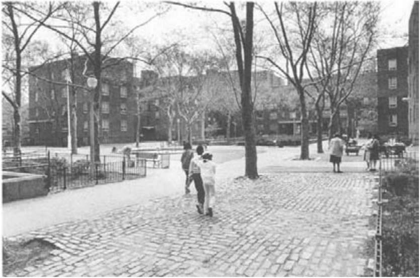
FIG. 6.1 The Harlem River Houses in New York City. This complex, completed in 1937, was built directly by the PWA to serve African-American New Yorkers. The architectural team was headed by Archibald Manning Brown and included Will Rice Amon, Richard W. Buckley, Frank J. Forster, Charles F. Fuller, Horace Ginsbern, and John Lewis Wilson. This 1987 photograph shows the view looking north along the central courtyard. Vic Delucia / NYT Pictures.
