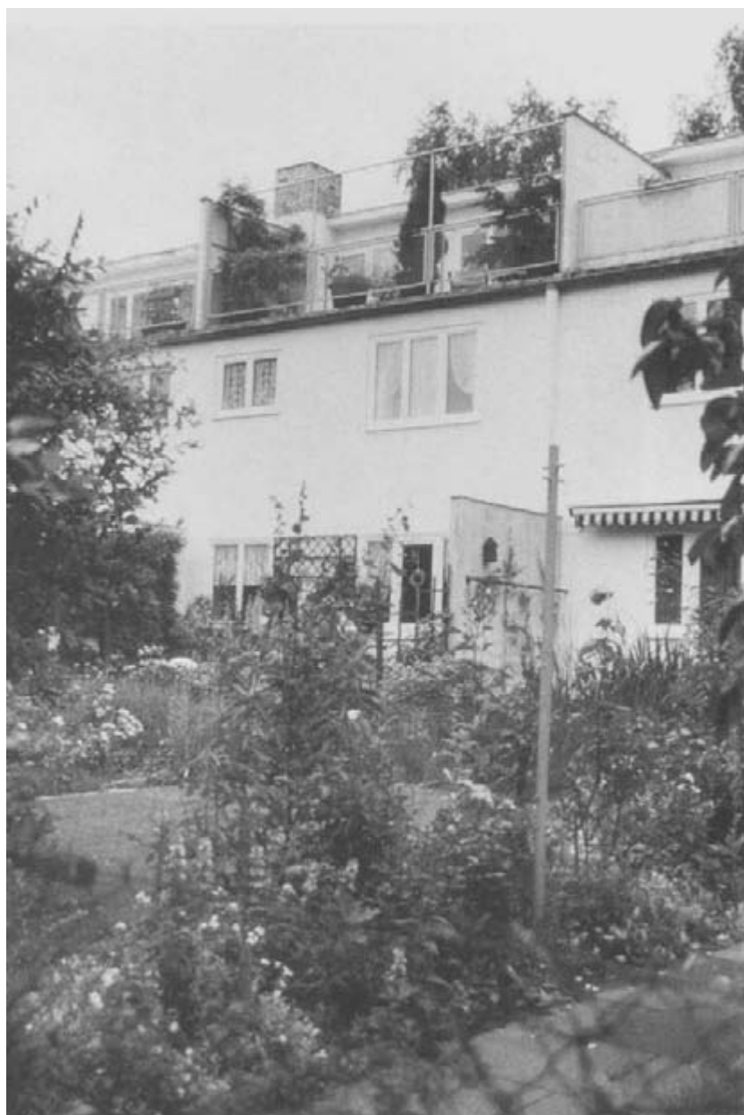
FIG. 3.5 This photograph, taken in 1990, shows the garden side of two-unit rowhousing at Praunheim, a settlement adjacent to Römerstadt. The first two floors form one dwelling, while the apartment at the top was designed as a rental area for owners living below. As the apartments lacked direct access to the garden area, they were provided with open terraces at the rear. At Praunheim, May began using large precast concrete blocks to construct building shells, much like the ones Grosvenor Atterbury had used at Forest Hills Gardens. Eventually, May built just under 900 dwellings using this process.
