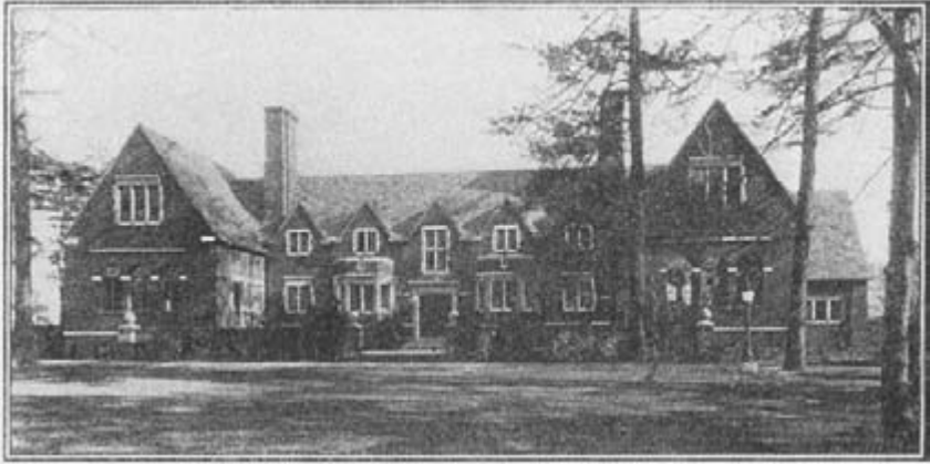
FIG. 2.6 The neighborhood center in Moorestown, New Jersey, built in the 1920s. Much like the facility envisaged for Union Park Gardens, it included a swimming pool, a gymnasium with stage, a children's health clinic, and meeting rooms to be used by local organizations. This commodious and well-appointed building provides evidence that affluent families were interested in having much the same kind of neighborhood amenities that housing reformers of the era desired to provide to those of more modest resources. In the 1990s, this building is still in use and in excellent condition.
