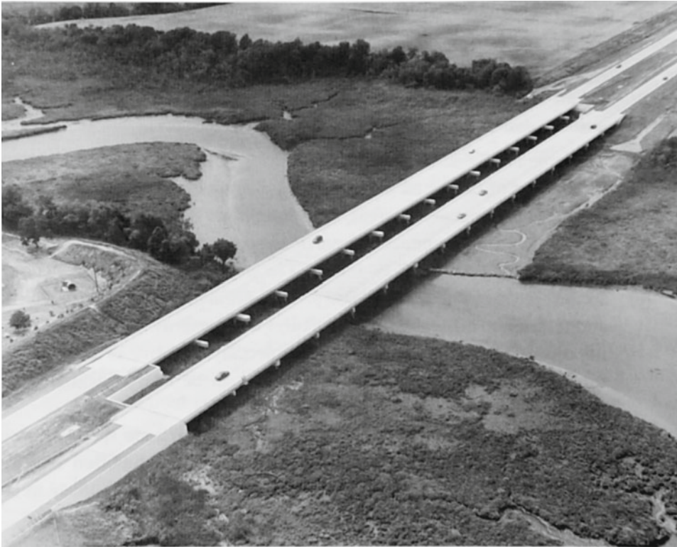
Figure 4-8 Tidal wetland and river spanned by multilane highway bridge that facilitates wildlife and floodwater passage (Forman, 2008, Reproduced with permission of Cambridge University Press, Redrawn by Yuan Ren, 2014).
