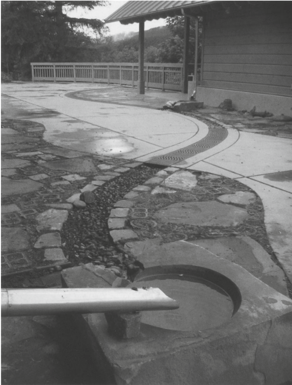
Figure 6-15 Downspouts serve as an artistic element in the courtyard (Miller, 2005, Reprinted with permission of University of Washington Press).
