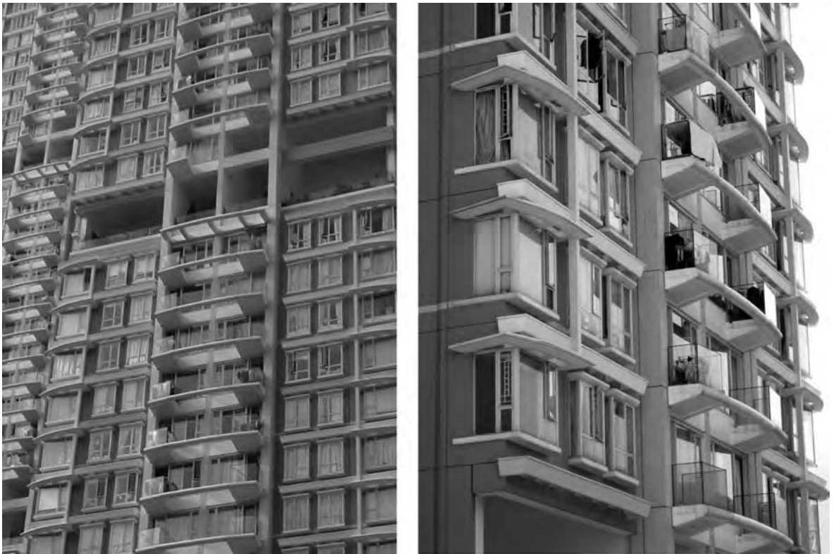
Figure 14.9 Prefabrication construction adopted at The Orchards in 2003
