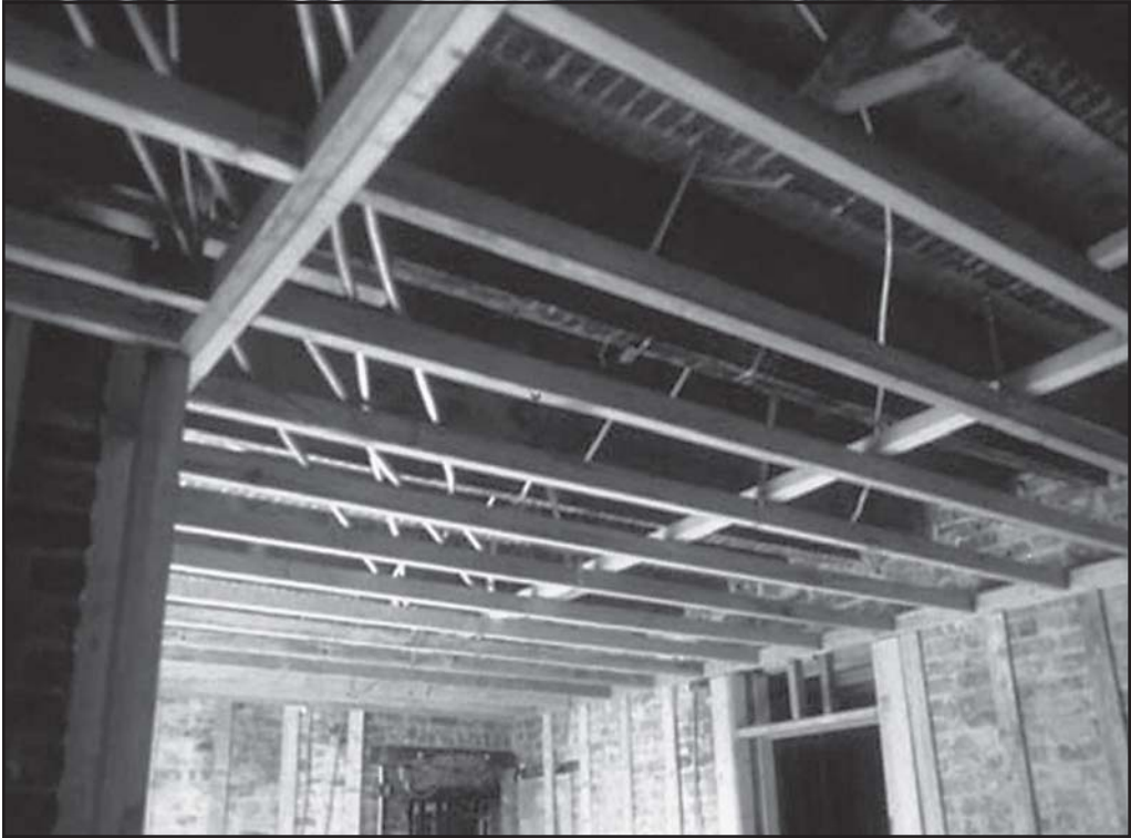
Fig. 12–3. Suspended ceiling are found in renovated buildings on all floors.
