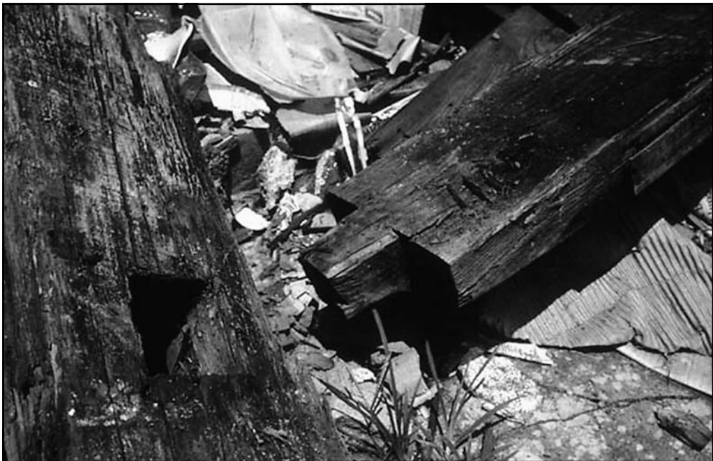
Fig. 15-7. A wood mortise and tenon connection
