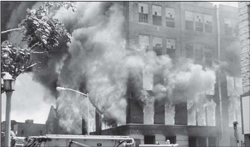
Fig. 3-5. Large fire in a Type IV heavy timber construction that creates a radiated heat fire spread problem for surrounding structures.
