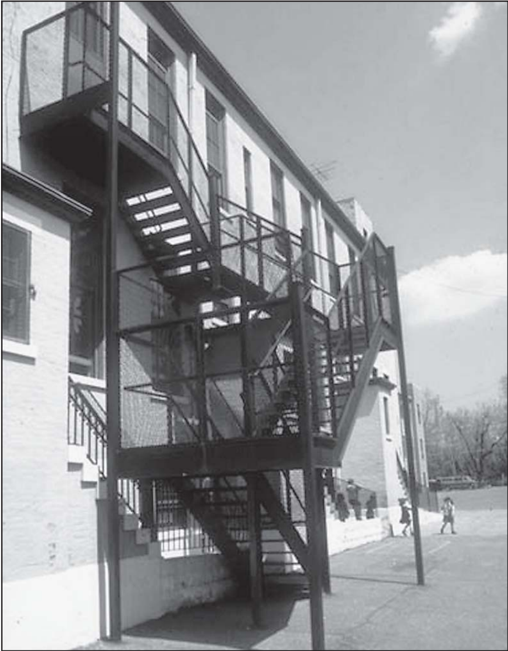
Fig. 14–1. An exterior fire escape screened-in balcony is the safest type of fire escape exit.
