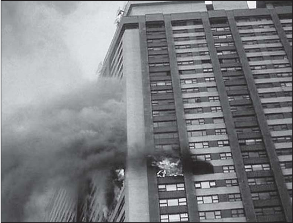
Fig. 3–6. Type I reinforced concrete structure suffers concrete spalling during a fire.
