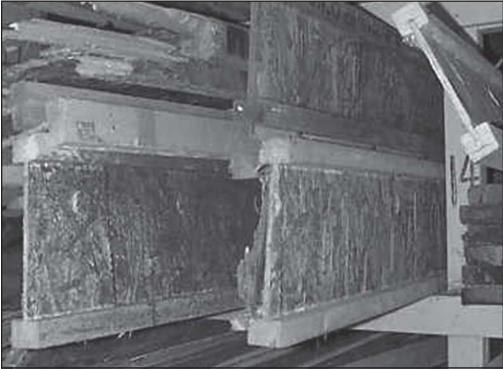
Fig 23–2. Lightweight wood I-beams have a wood web member and a 2×2 inch top and bottom flange.
