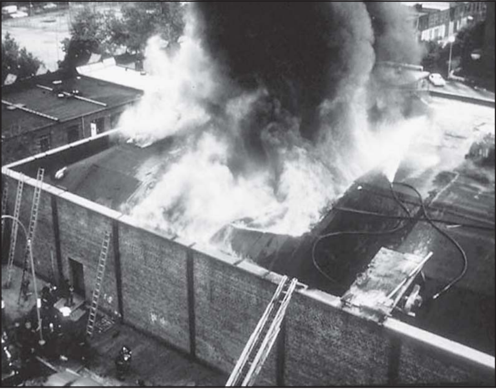
Fig 8–1. The truss roof collapse at the Waldbaum's supermarket in Brooklyn, NY, in 1978
