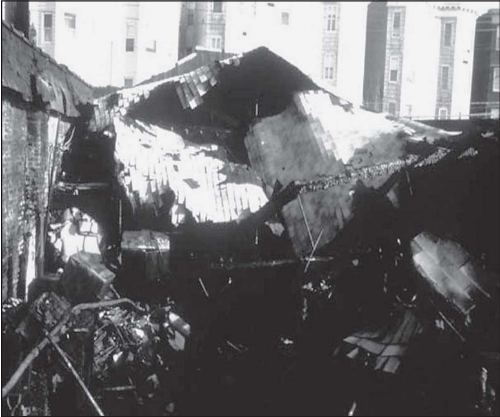
Fig. 7-4. Lieutenant Harry Korwatch of the Yonkers, NY, FD was killed when the roof deck collapsed.
