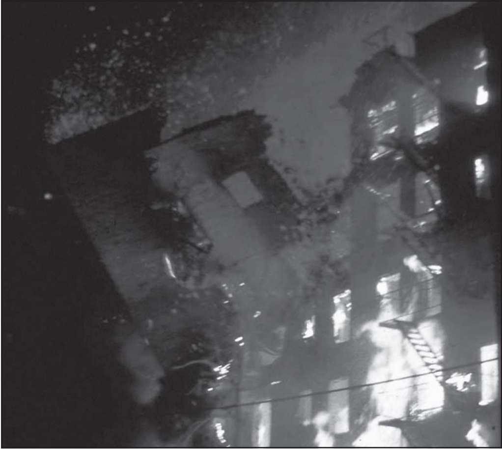
Fig. 1–2. The age of a building increases its collapse danger.
