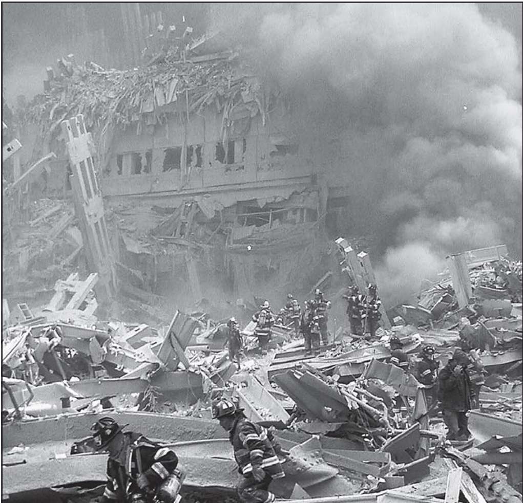
Fig. 20-1. The World Trade Center following its collapse
