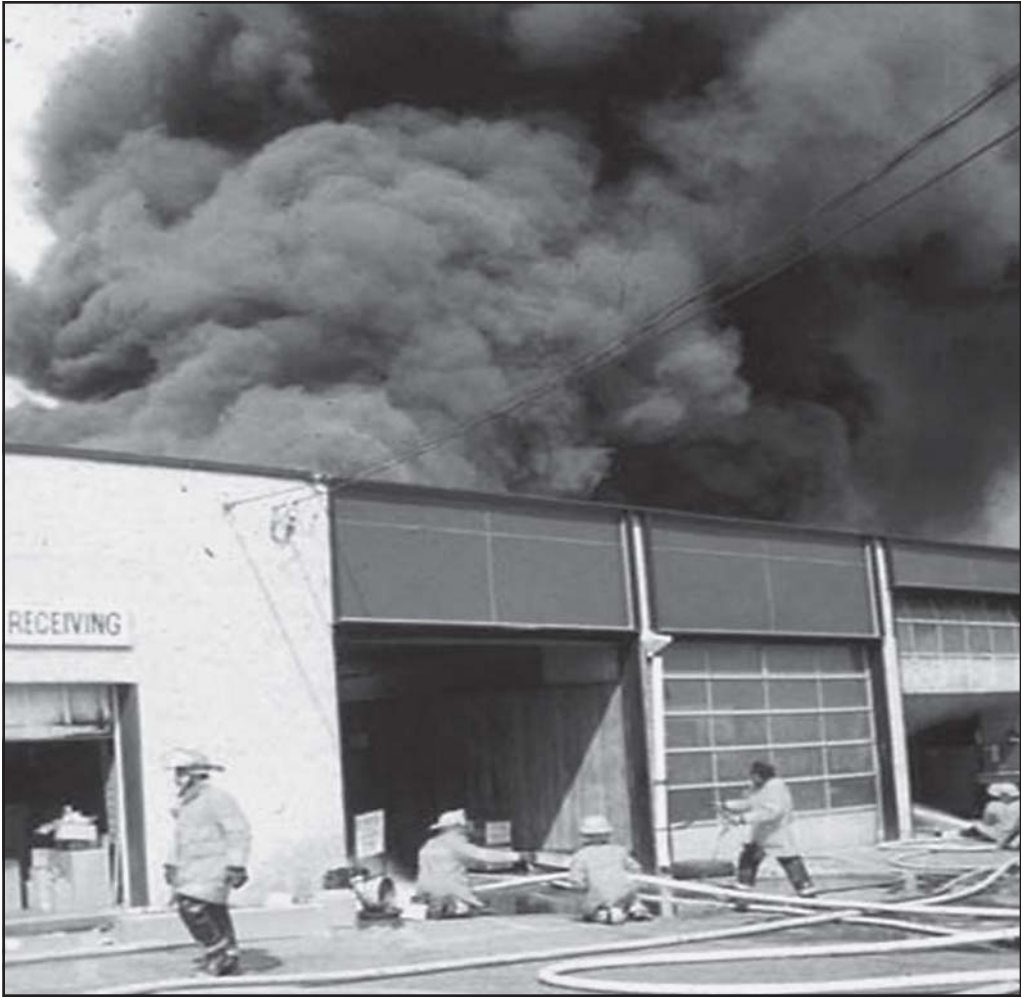
Fig. 8–3. Five firefighters from the Hackensack, NJ, FD were killed in this bowstring truss roof collapse.
