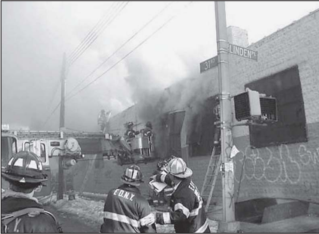
Fig. 10–1. A lightweight Type II constructed building with an open-web bar joist roof presents a collapse danger to firefighters. As a precaution, the use of horizontal ventilation is recommended.
