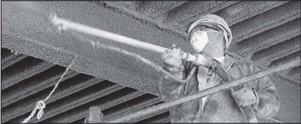
Fig. 10–3. Spray-on fire retarding material to protect steel
