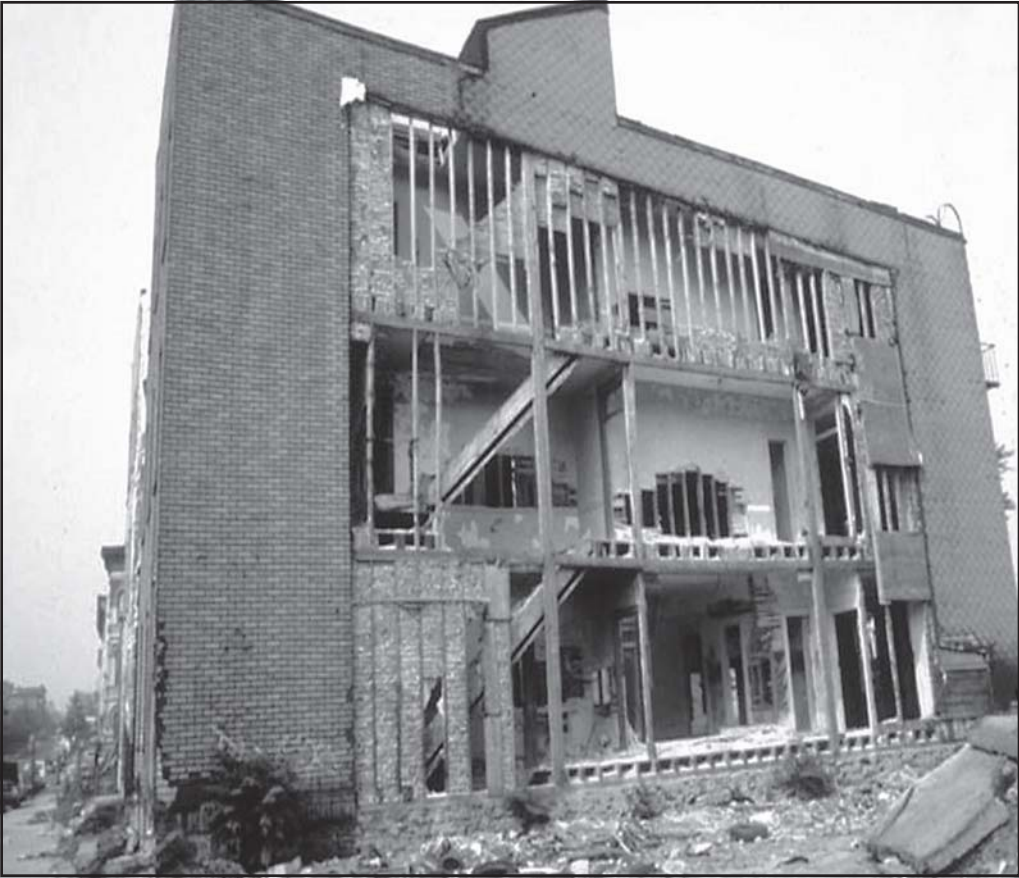
Fig. 15–5. Braced-frame construction
