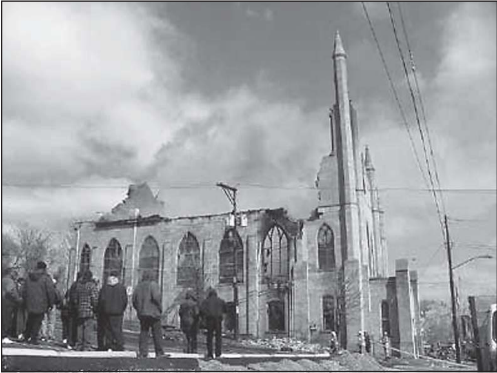
Fig. 8–12. The scene after the steeple and roof collapsed in Pittsburgh, PA
