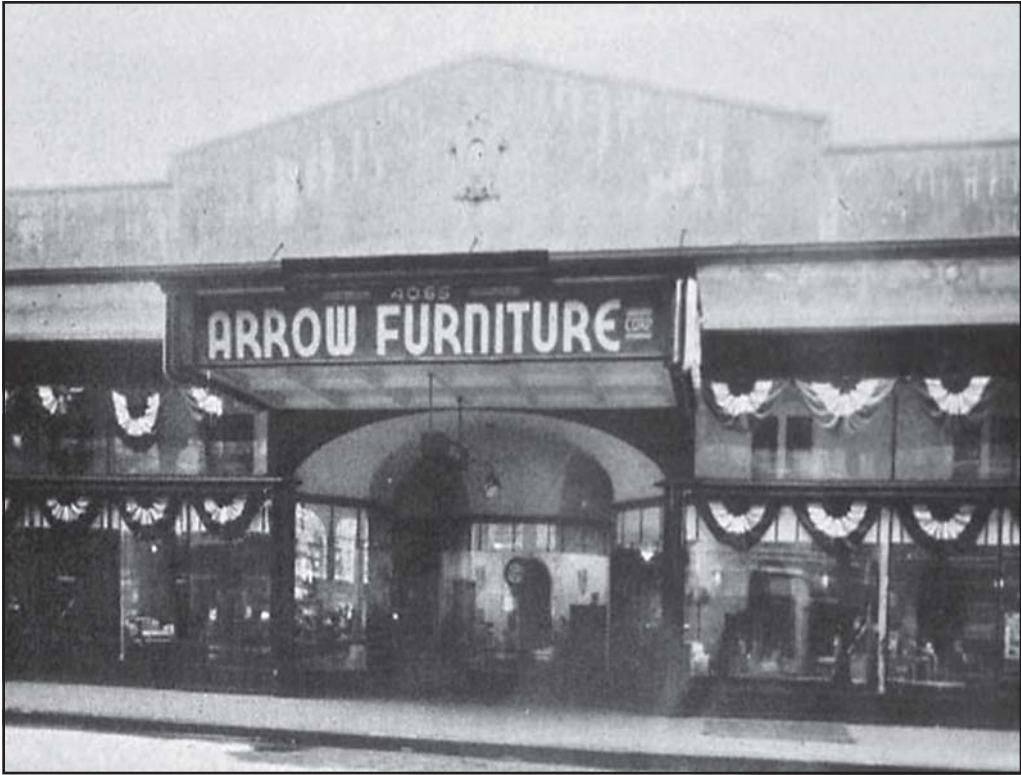
Fig. 5-5. This marquee and parapet wall collapsed and killed six FDNY firefighters.
