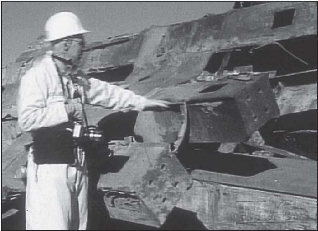
Fig. 20–6. The World Trade Center had tubular bearing walls; some only one-half-inch thick on the upper floors.
