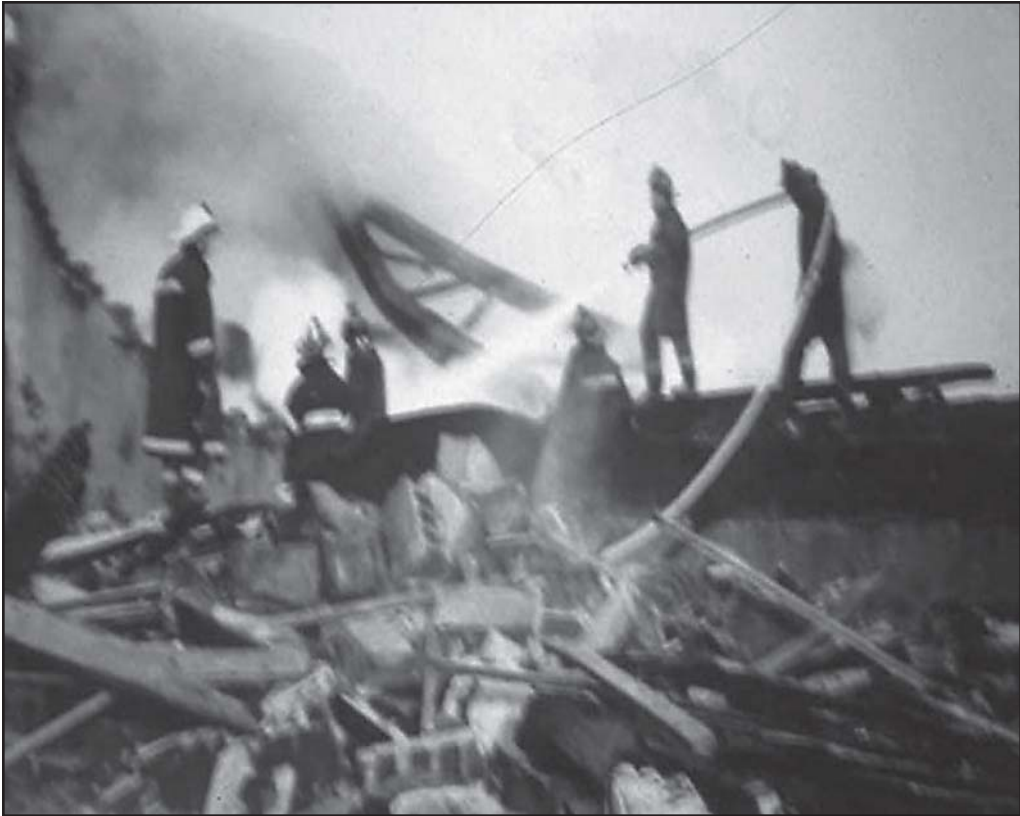
Fig. 8–2. This truss roof collapse in Cliffside Park, NJ, killed five firefighters from Ridgefield, NJ, who responded on mutual aid.
