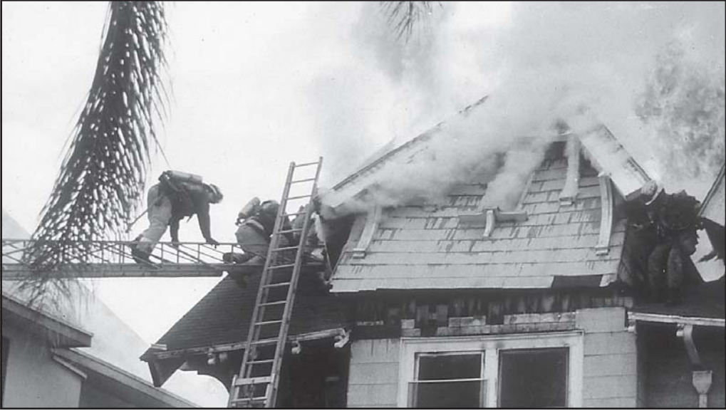
Fig. 7-1. A ridge rafter peaked roof collapse
