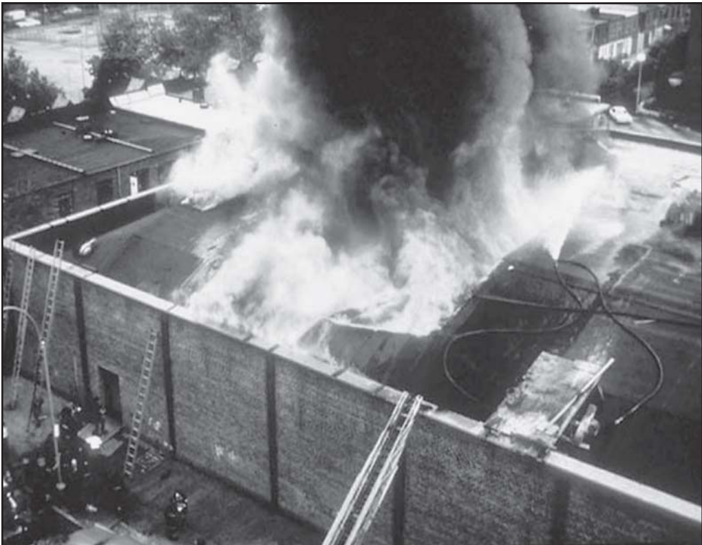
Fig. 22–1. Waldbaum's Supermarket timber truss roof collapse killed six FDNY firefighters in 1978.
