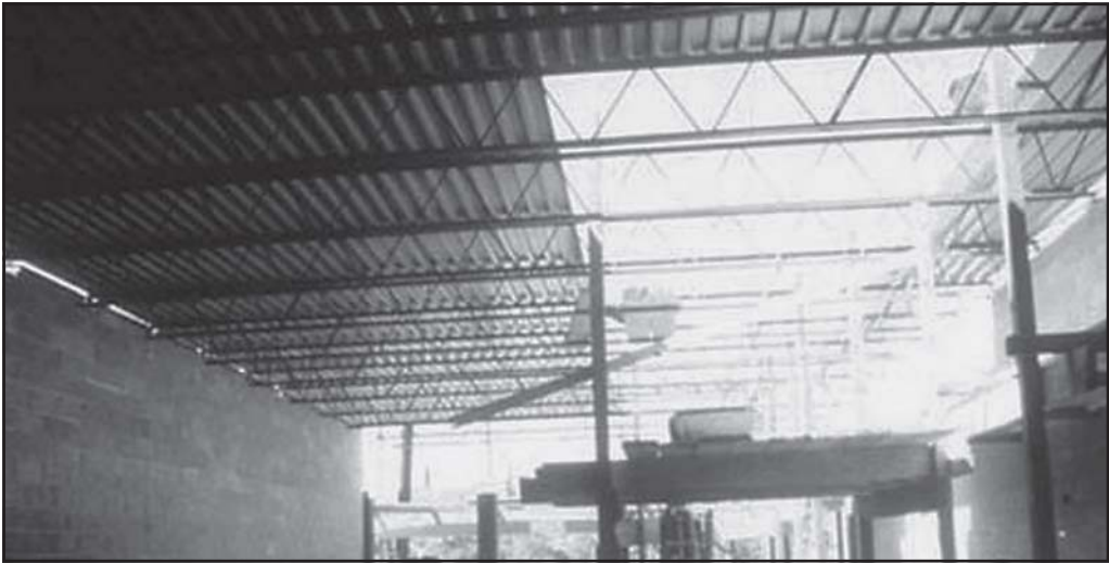
Fig. 10–4. Lightweight steel bar joist roof construction
