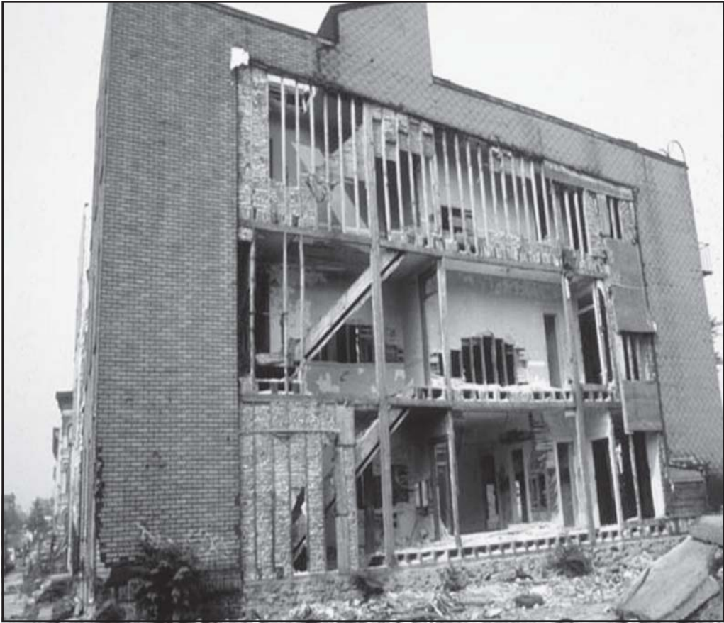
Fig. 2–3. Brace-framed construction has posts and girts fastened by mortise-and-tenon joints.
