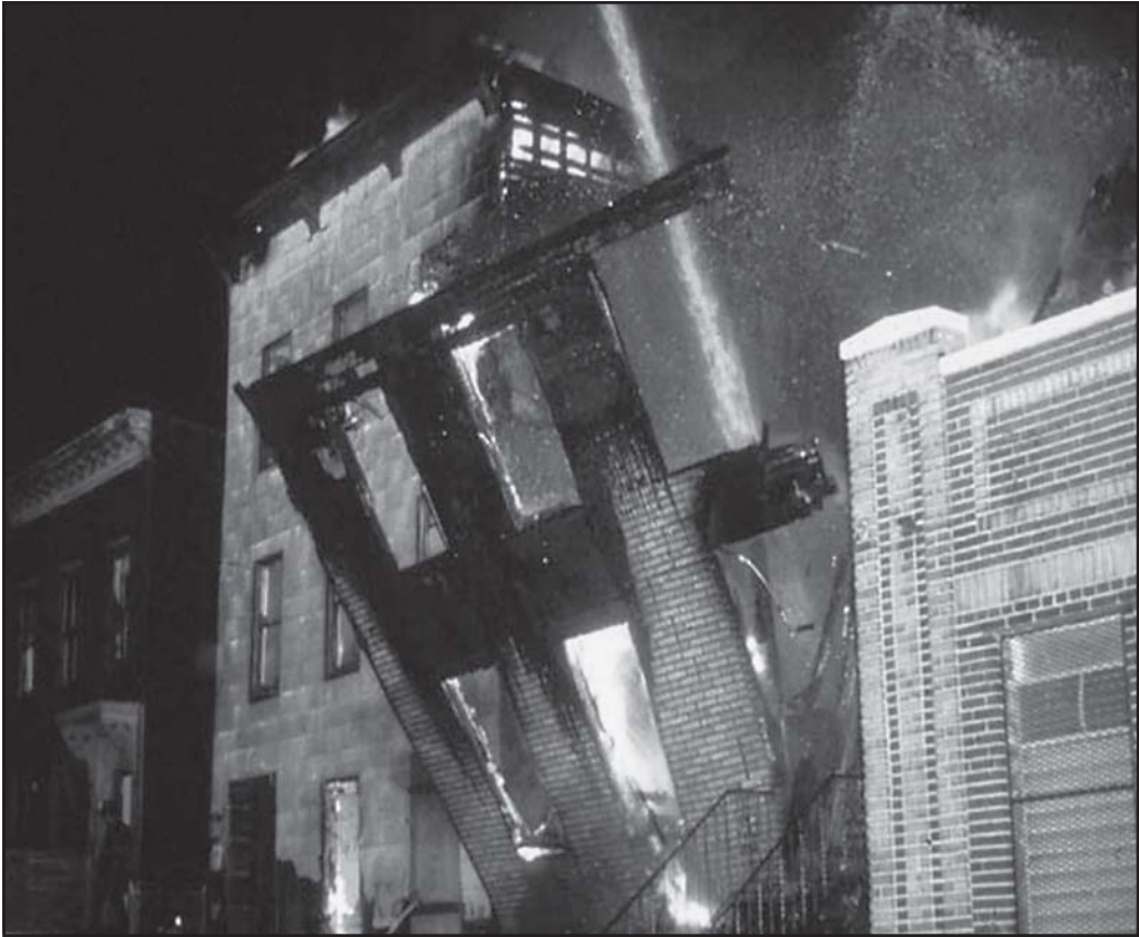
Fig. 15–2. A 90-degree wall collapse
