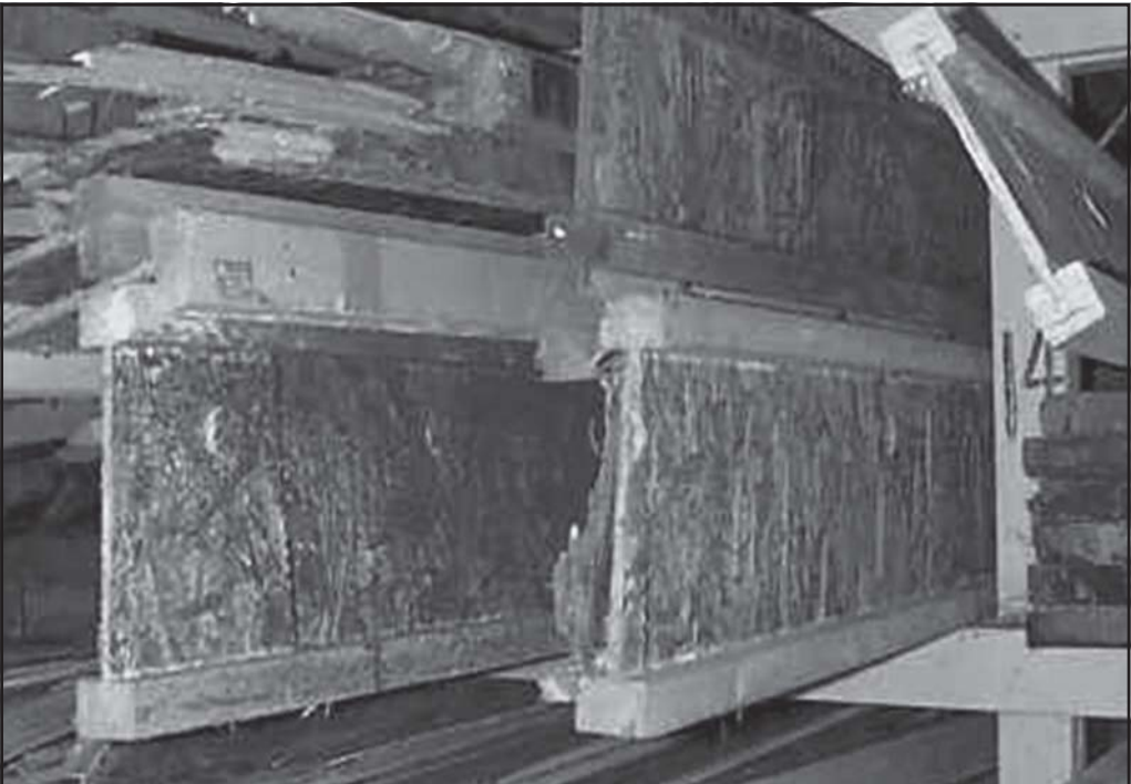
Fig. 2–14. Wood I-beams have a web section connected with top and bottom wood flanges.
