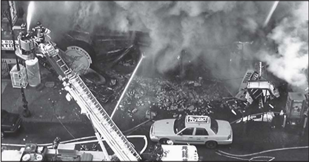
Fig. 5–4. This parapet wall supported by steel lintel collapsed suddenly during a fire.
