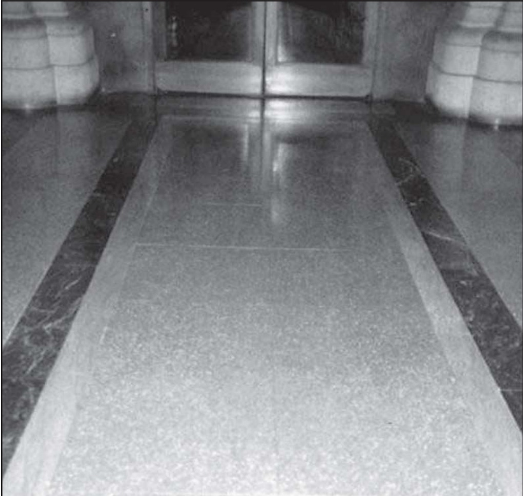
Fig. 2-19. Terrazzo floors have polished marble chips in cement.
