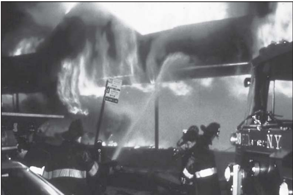
Fig. 5-1. A parapet wall supported by a steel lintel with flame flowing out the opening below the steel lintel is distorting the steel support.
