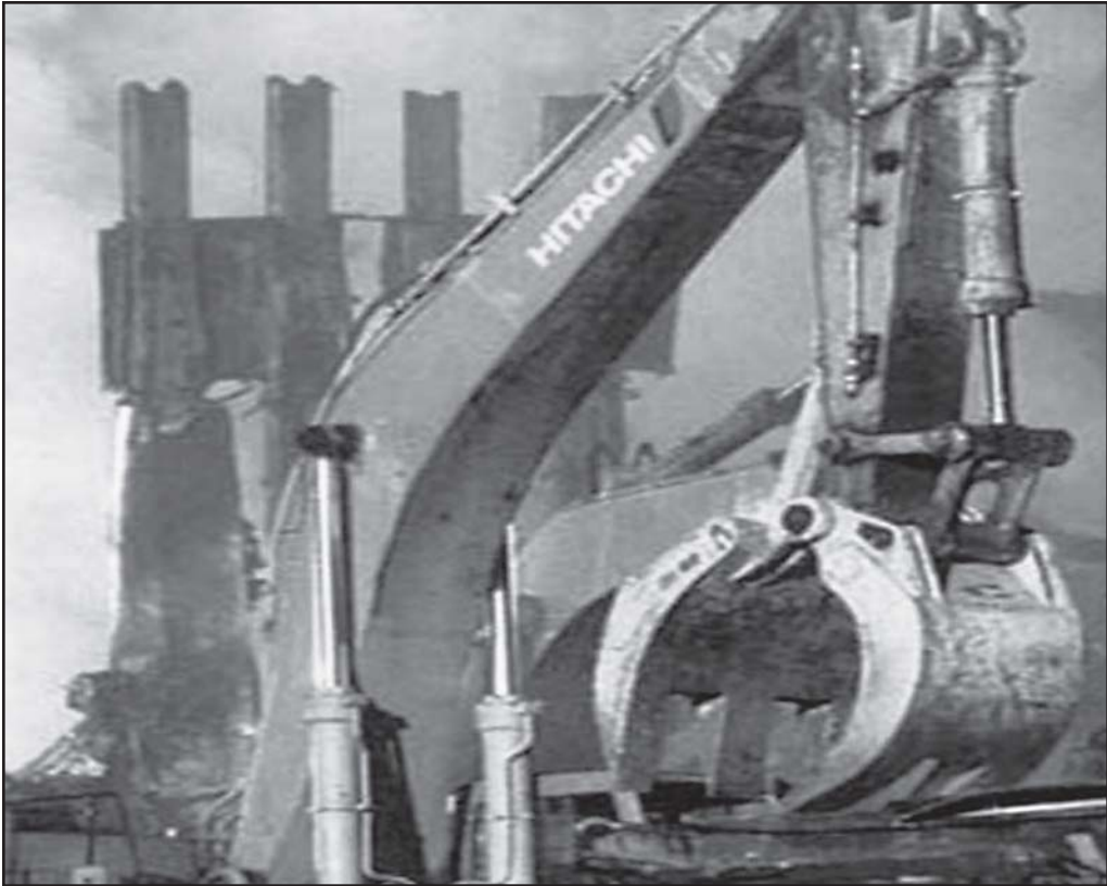
Fig. 18–12. General debris removal in progress
