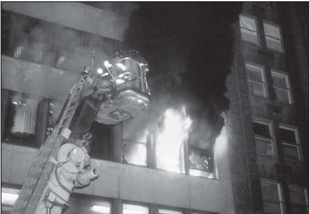
Fig. 3-1. Type 1 fire-resistive construction may allow fire spread by auto exposure from window to window.
