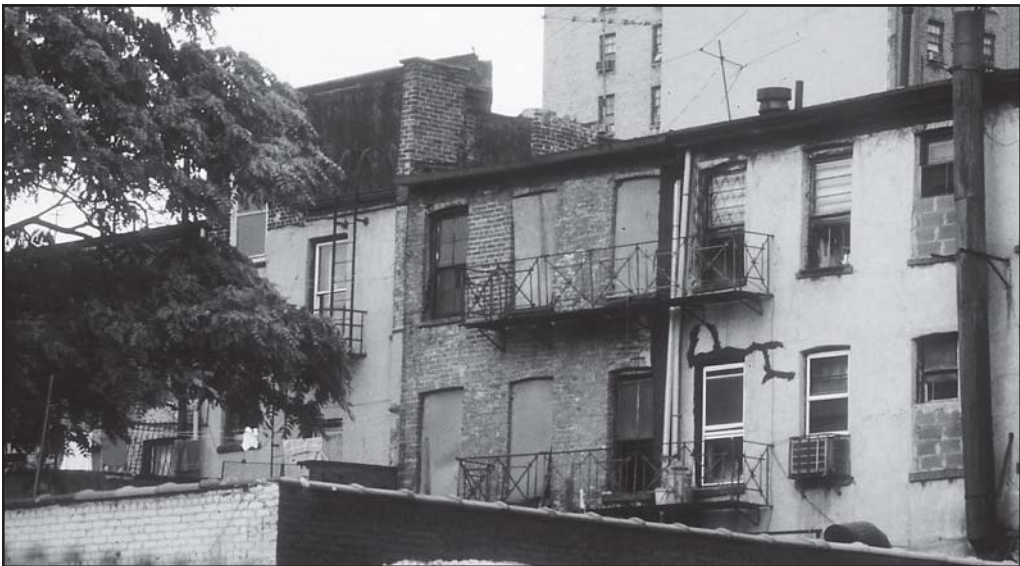
Fig. 14–2. A party balcony fire escape is often overloaded with occupants fleeing a fire.
