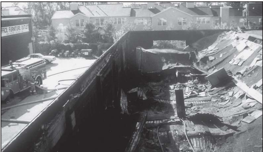
Fig. 10–5. Unprotected lightweight open-web steel bar joist can collapse within 5 to 10 minutes of exposure to fire.
