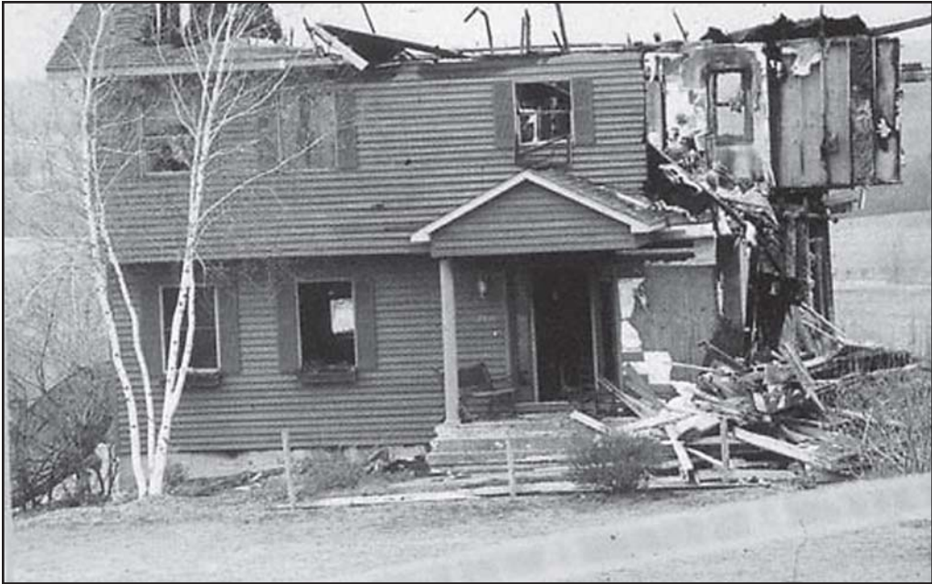
Fig. 11–4. Firefighters Tim Lynch and John Ginocchetti died when the floor collapsed in this private dwelling.
