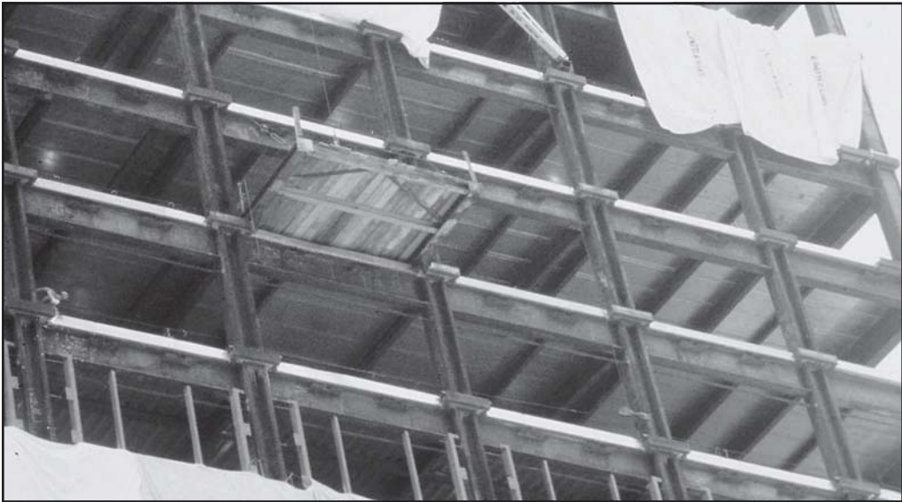
Fig. 16–4. Scaffolding can extend beyond the edge of a building under construction.
