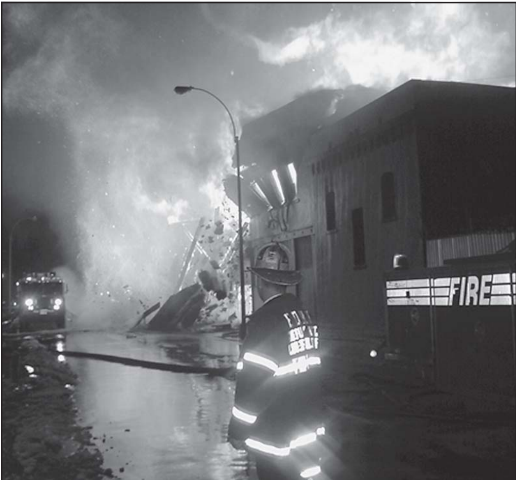
Fig. 4–2. A masonry wall falling at a 90-degree angle
