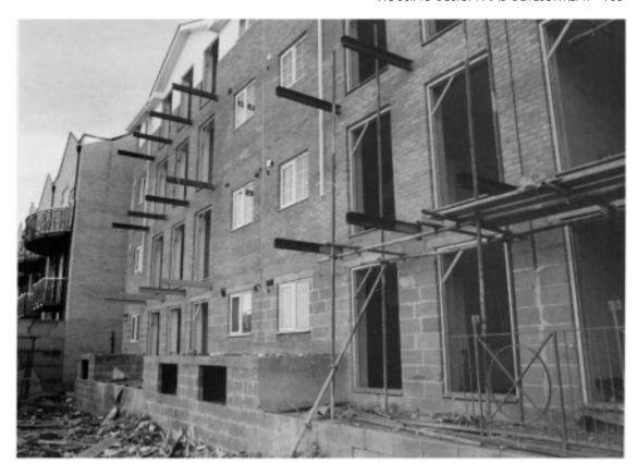
Plate 6.2 King's Bridge Court, front elevation during construction The protruding steel beams will support balconies similar to those that can be seen in the background. The blockwork is to be rendered, as on the rear elevation
