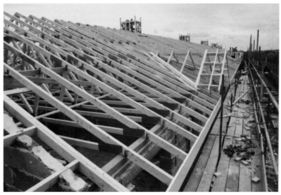
Plate 6.4 King's Bridge Court, pitched roof during construction
