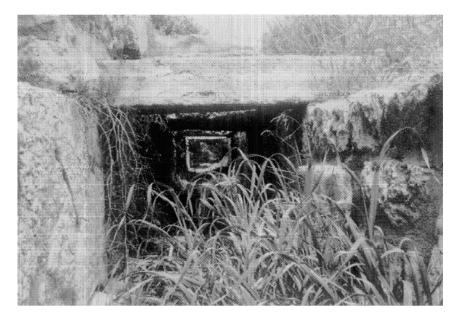
**Figure 17.11.** Great drain, Athenian Agora, no later than the sixth century B.C. This drain is 1 to 1.25 meter wide and up to 2 meters deep.
