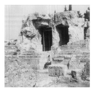
**Figure 11.3.** Glauke Fountainhouse, Corinth. Sculpted from a huge block of stone that remained after the Temple of Apollo was constructed in archaic times, this fountainhouse seems never to have been a spring, but rather to have been supplied by pipes bringing water from uphill. The arched openings cut in the rock are approximately 4 meters tall.
