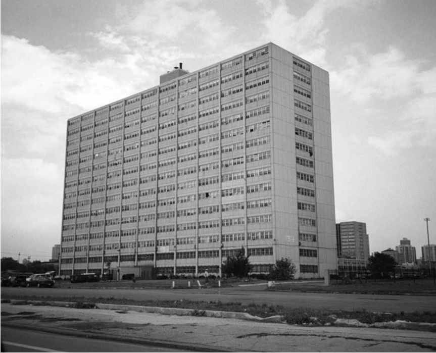
Figure 5. Photograph of 1230 North Burling Street, Chicago, IL, 2000
