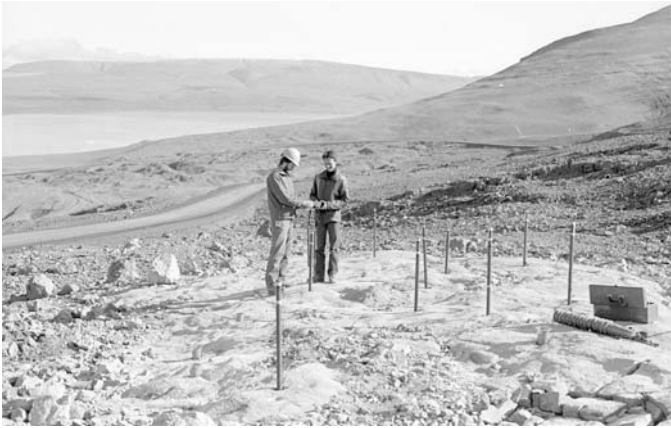
Figure 21.4 Installation of the 12 anchors.
