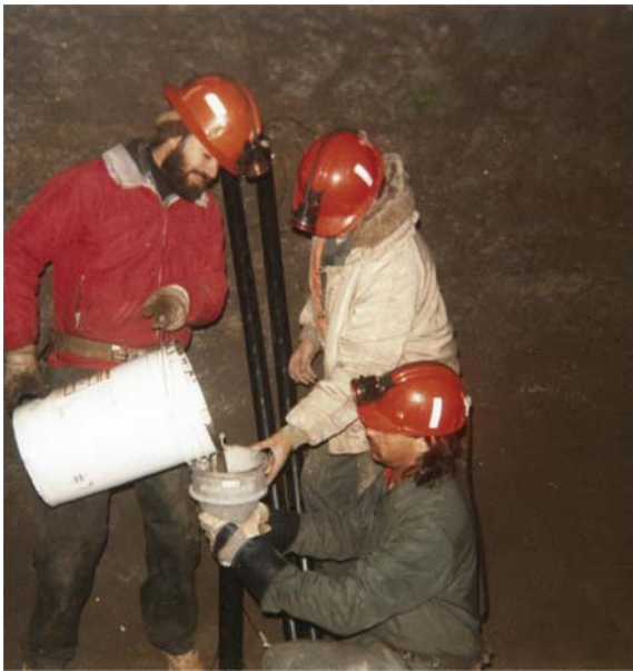
Figure 21.3 Grouting the anchors in the mine gallery.
