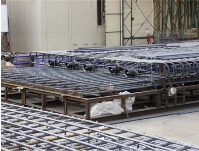
Figure 27.16 The reinforcing system of the conventional slabs.
