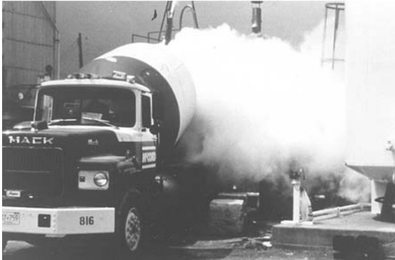
Figure 18.1 Cooling concrete with liquid nitrogen. Courtesy of John A. Bickley.
