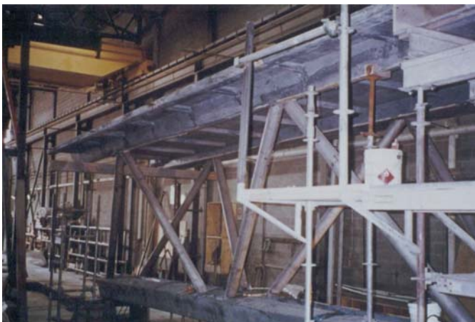
Figure 27.7 Construction of a prefabricated element in the pre-cast plant.
