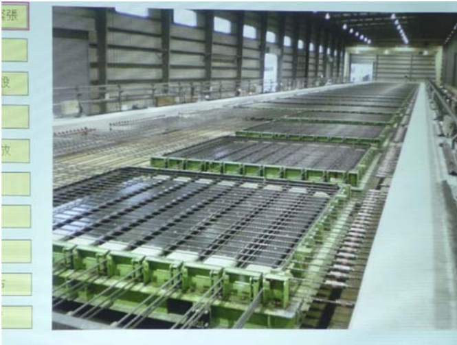
Figure 27.19 Installation of the pre-tensioned reinforcing system.
