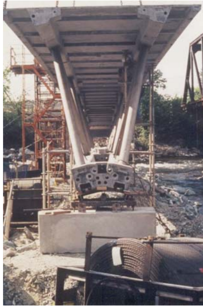
Figure 27.10 Assembling the northern part of the bridge.
