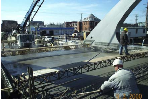
Figure 5.2 Fogging to prevent plastic shrinkage. Courtesy of Richard Morin.
