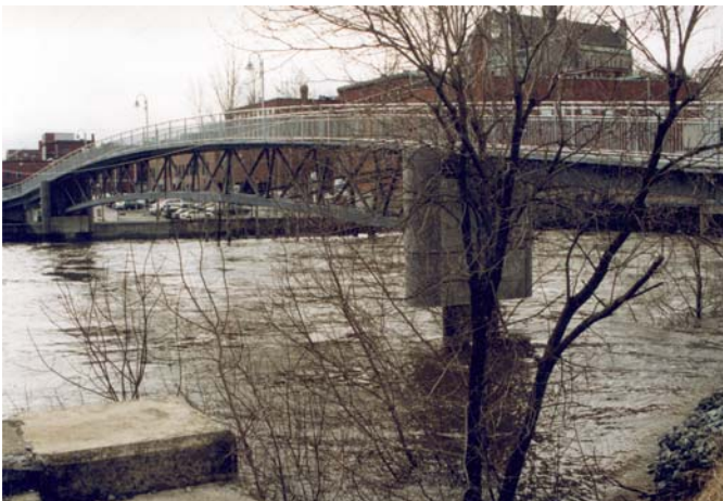
Figure 27.13 The completed Passerelle.
