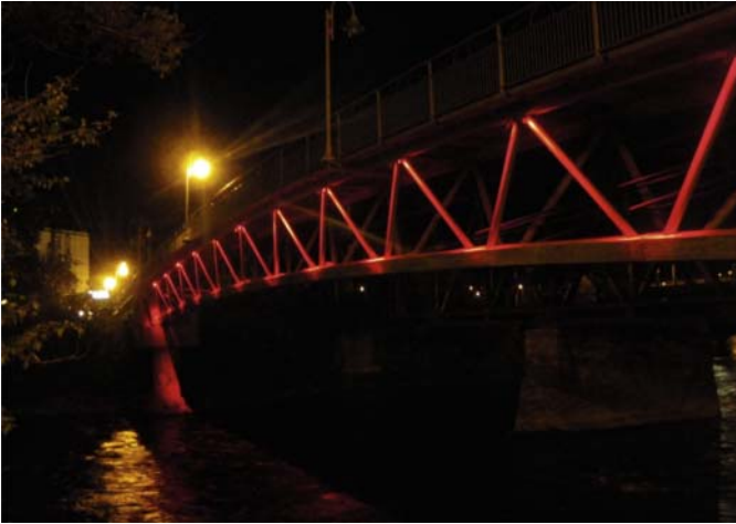
Figure 27.14 The Passerelle at night.
