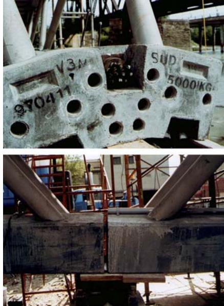
Figure 27.11 Assembling two prefabricated elements (dry joint).
