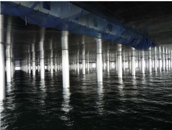
Figure 27.15 The additional landing strip built at Haneda Airport in the Bay of Tokyo.
