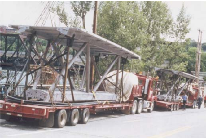
Figure 27.9 Transportation of the prefabricated elements.
