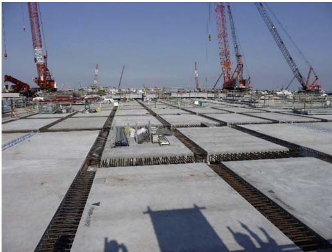
Figure 27.17 Installed slabs made of conventional concrete.
