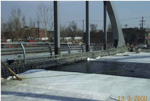
Figure 5.3 Application of saturated geotextiles 24 h after casting. Courtesy of Richard Morin.
