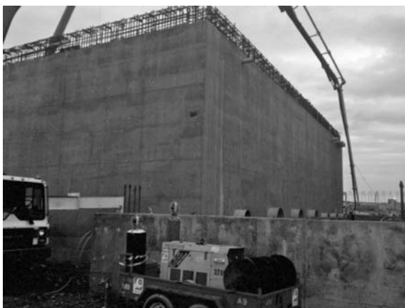
Figure 20.15 Construction of Fermont tank in Quebec using SCC1.
