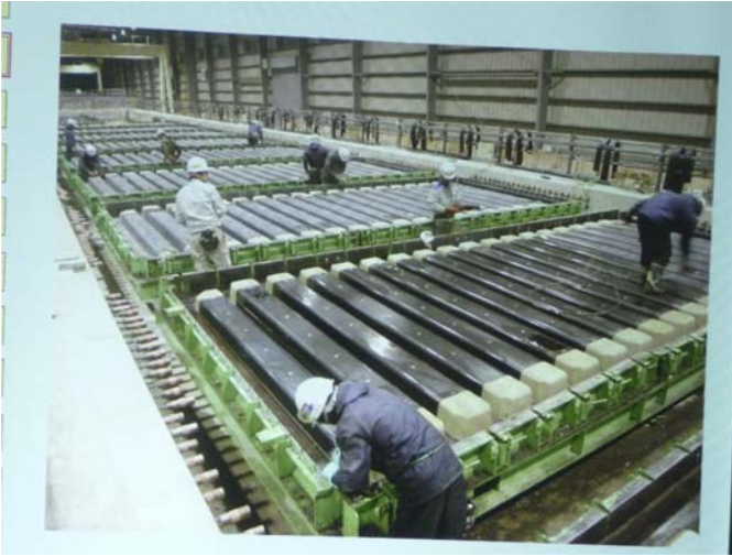
Figure 27.18 The moulds used to build the UHSC slabs.
