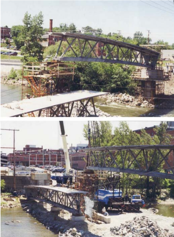
Figure 27.12 Assembling the two halves of the bridge.
