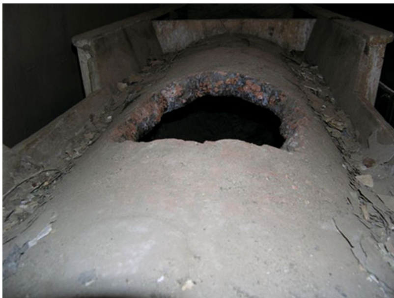
Fig. 2.5 Prop used for Andy's escape into the Shawshank sewer system, on permanent display at OSR. Note the thickness of its concrete opening
