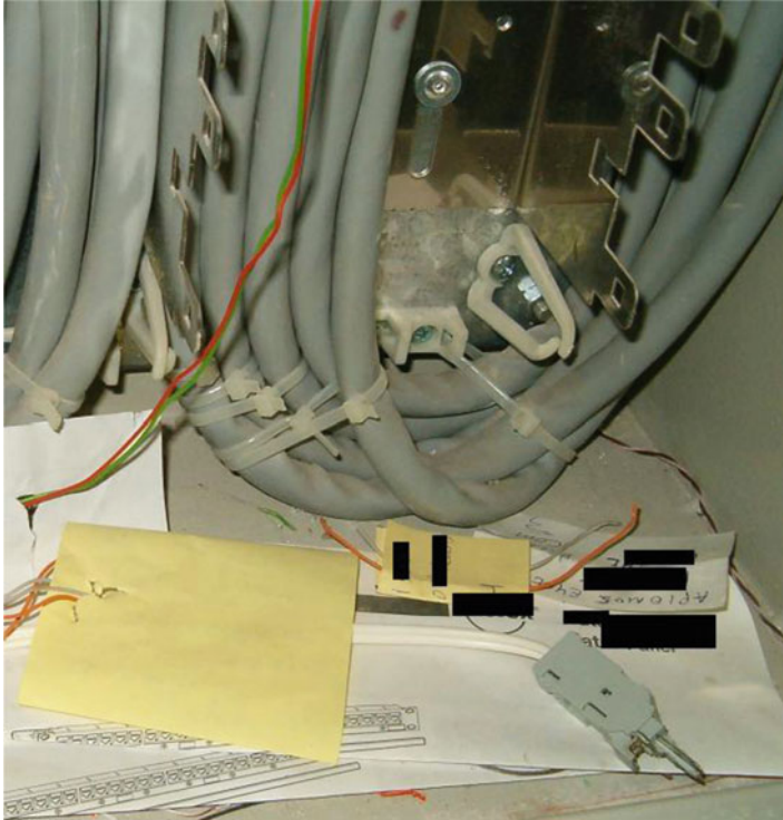
Fig. 2.2 Sensitive information left over in the distribution frame plus the tool to intercept calls
