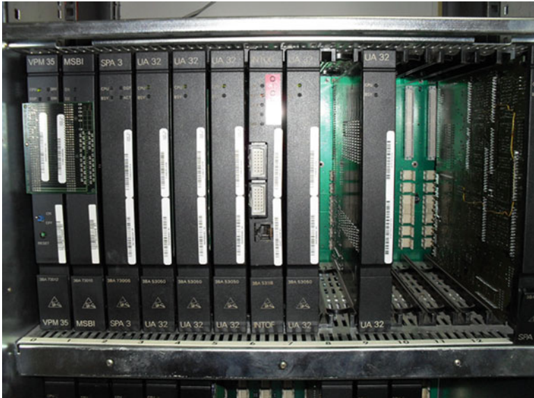
Fig. 2.5 Close-up of boards
