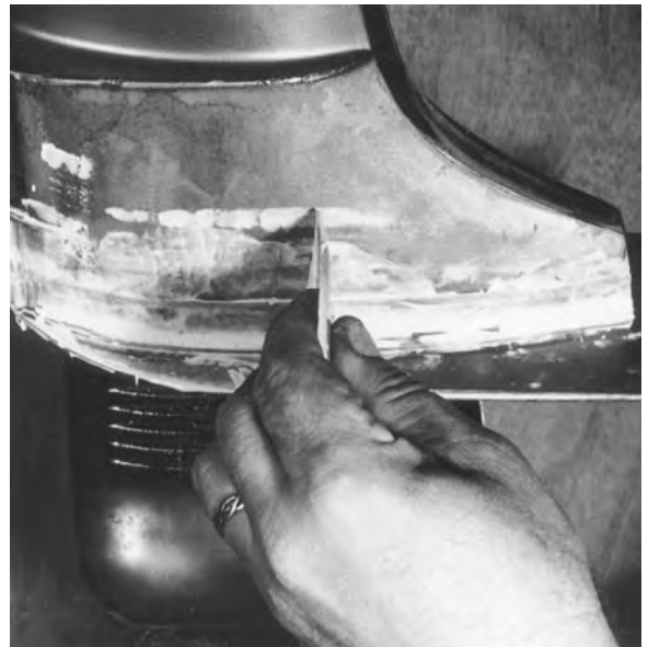
Figure 10-5. Filling corrosion pockets with epoxy putty.
