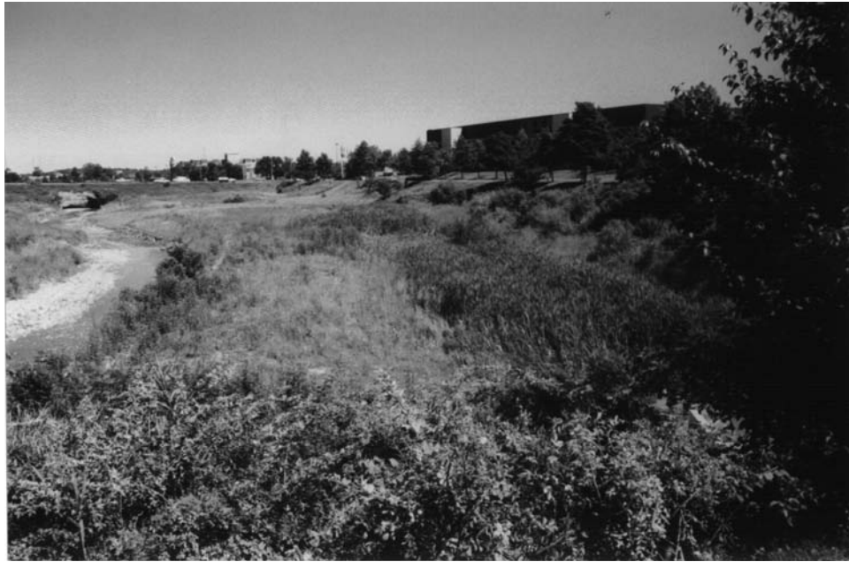
Stream restoration and stormwater retrofit project along White Marsh Run, one of Baltimore County's planned growth centers. This project provides for stable streams, enhanced habitat, and treatment of runoff from a regional shopping mall. Photograph courtesy of Baltimore County, Maryland.
