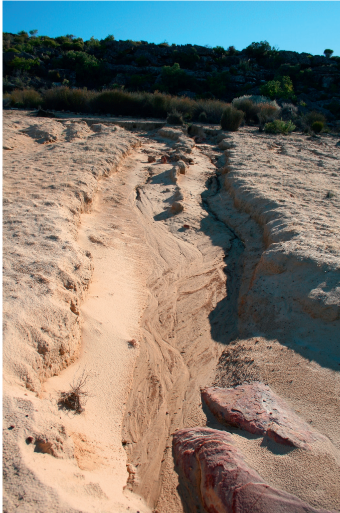
Erosion damage following the January 2000 Dobbelaarskop cloudburst.
