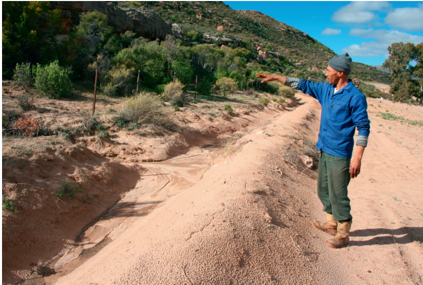
Hartweg Oktober demonstrates how a contour bund is controlling runoff from a rocky mountainside and enhancing the infiltration of water.
