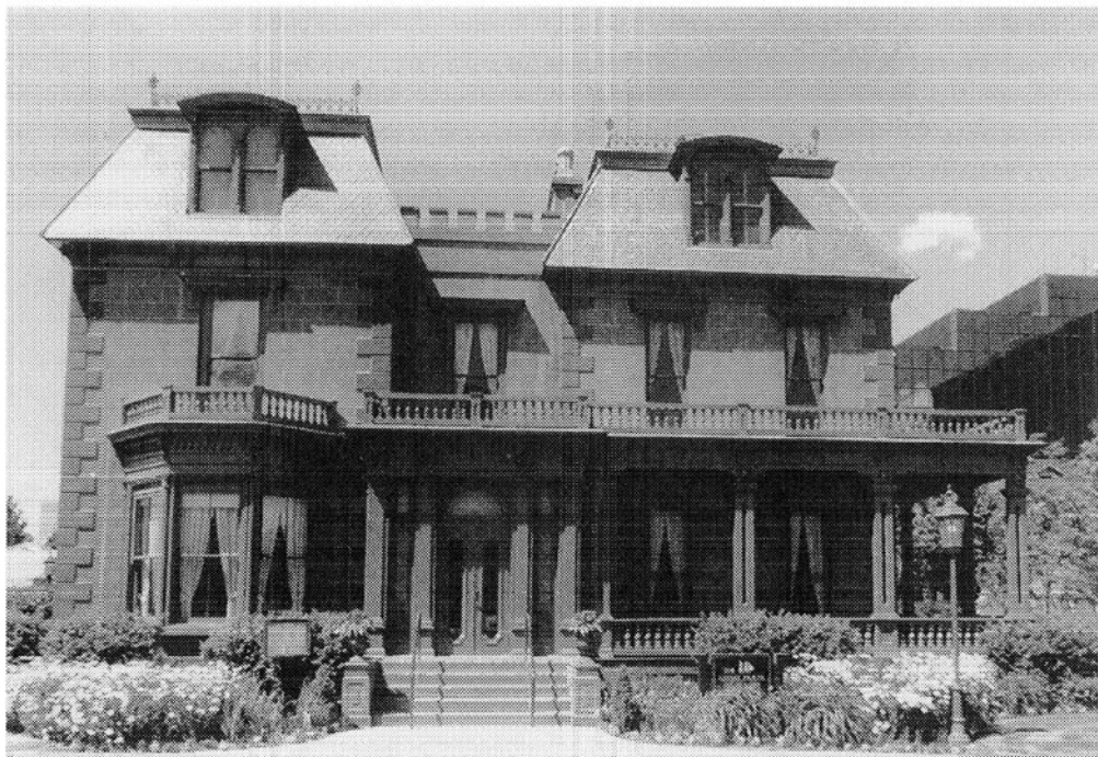
112. A view from the south of the Devereaux House (1856–57/1868/1877) in Salt Lake City. The adobe walls were stuccoed and scored to give the impression of ashlar construction. ( Author )
