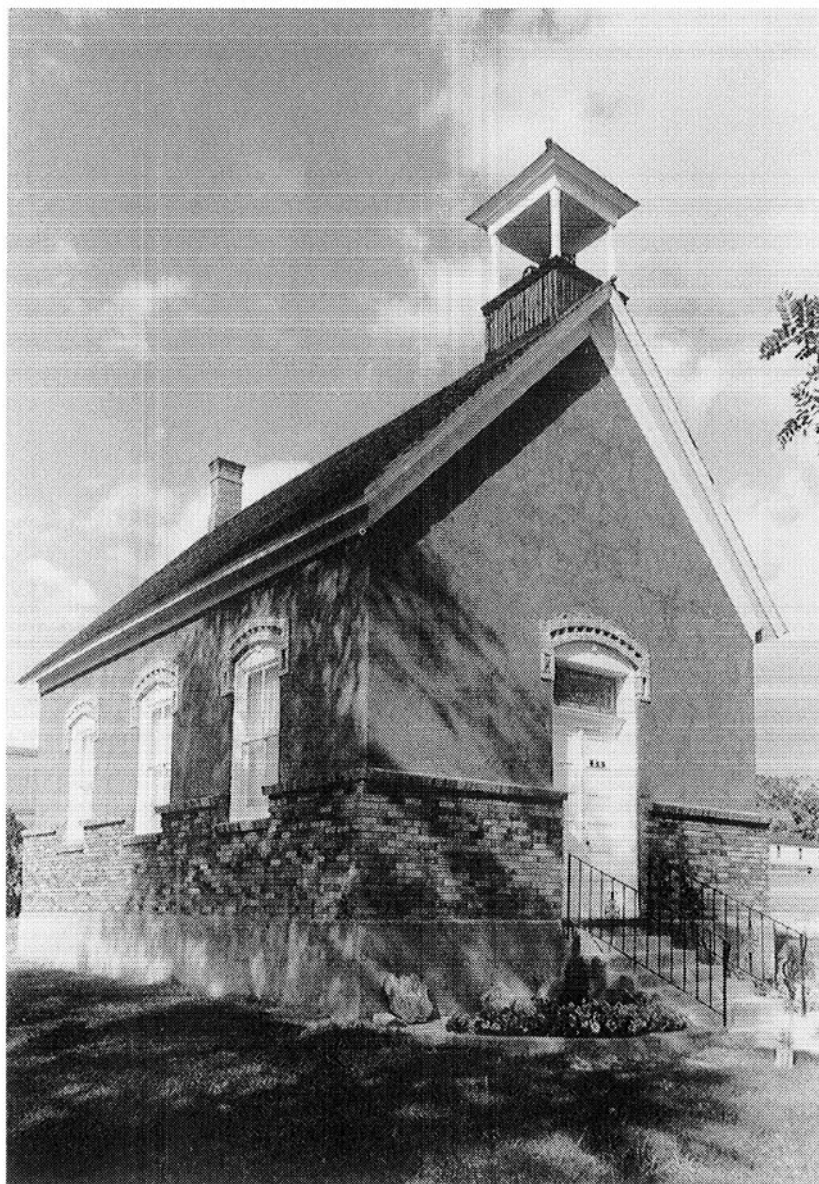
74. The Thurber (Bicknell) Relief Society Hall (1897–99) seen from the southwest. Decorative brick Victorian door and window hoods adorn the building. (Author)
