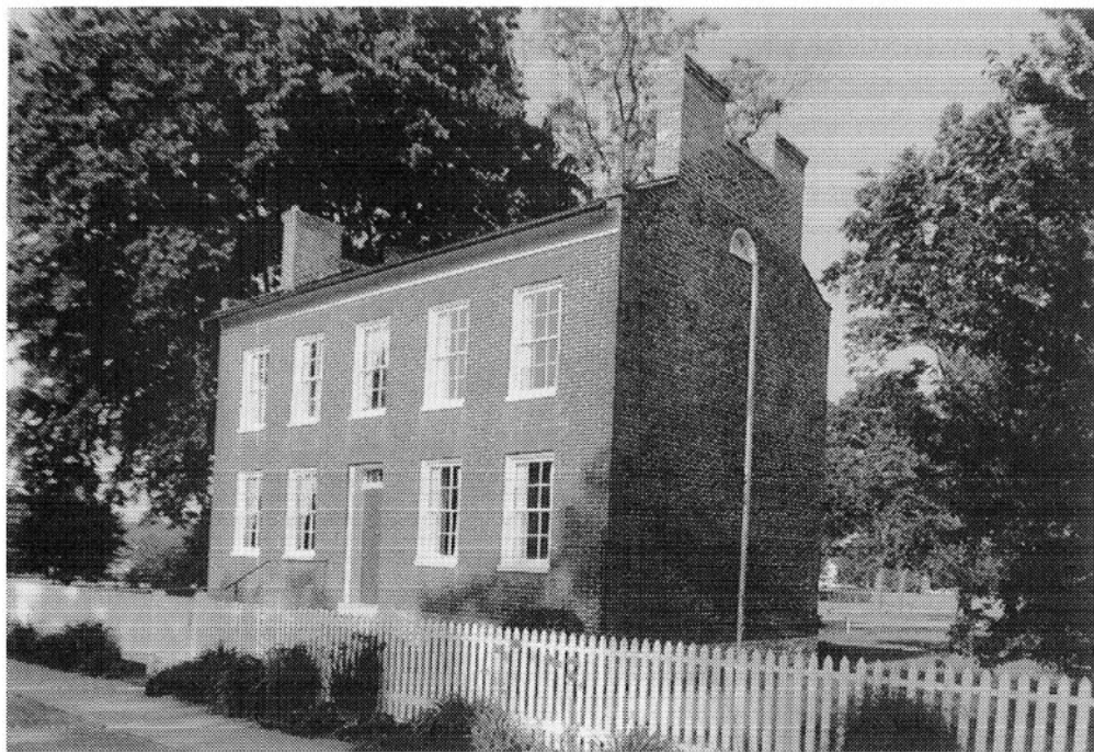
87. The Wilford Woodruff house (1843–45) seen from the northeast. It is one of the more refined dwellings constructed in Nauvoo. ( Author )
