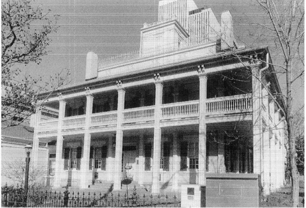
109. Brigham Young's Beehive House (1852–54) in Salt Lake City. The balcony (gallery) was probably added about the same time as the veranda and balcony on the nearby Tithing Office (Deseret Store). The view is from the southeast. ( Author )
