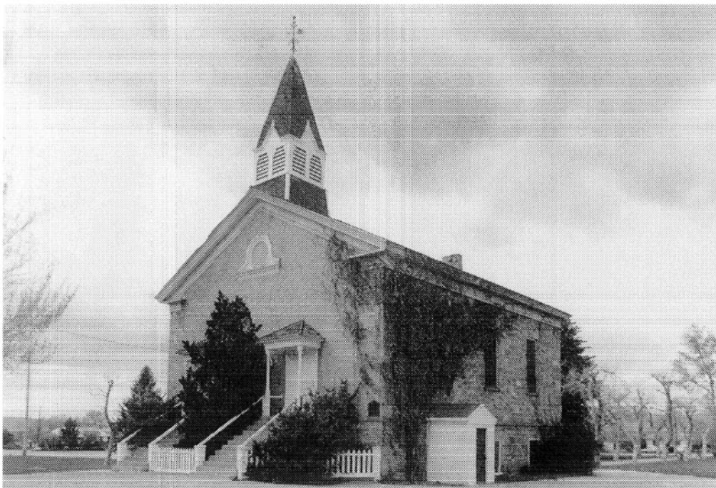
58. The Parowan Rock Meetinghouse (1861–70/1880s) seen from the southeast. Notice the difference between the stone sidewalls and the stuccoed front. (Author)
