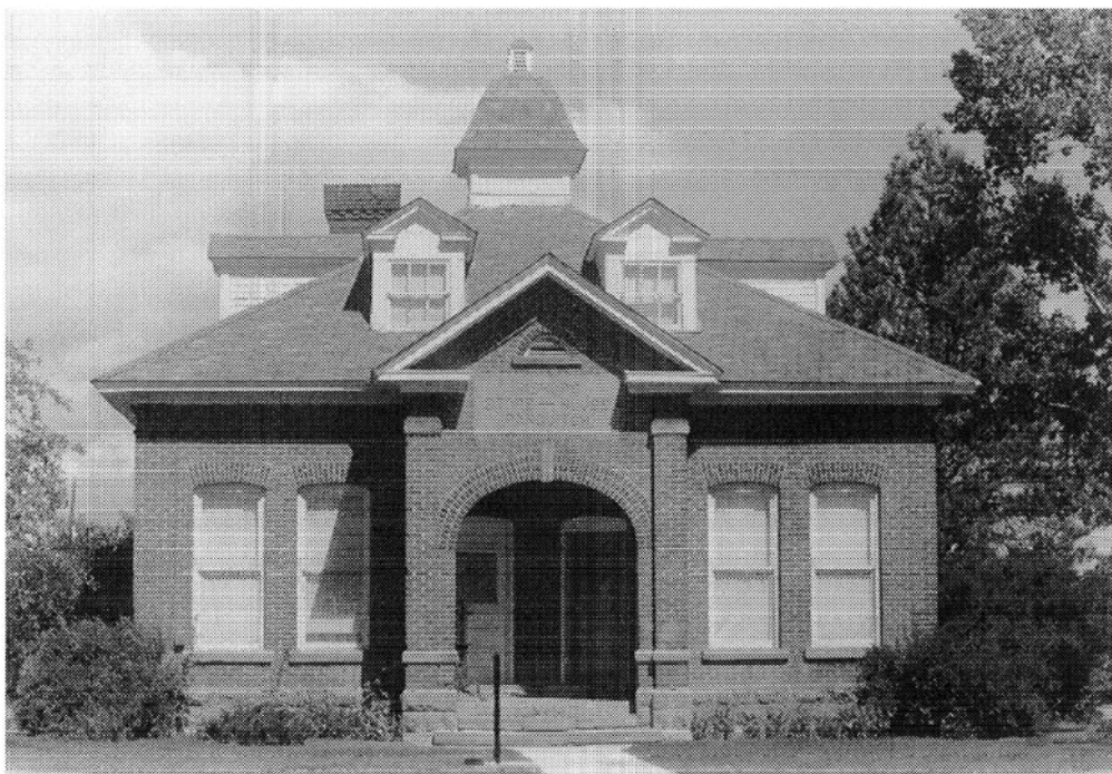
80. The Tithing Office or Bishop's Storehouse in Panguitch, Utah (1903). It is representative of the new type of tithing offices built at the turn of the century. The view is from the south. ( Author )
