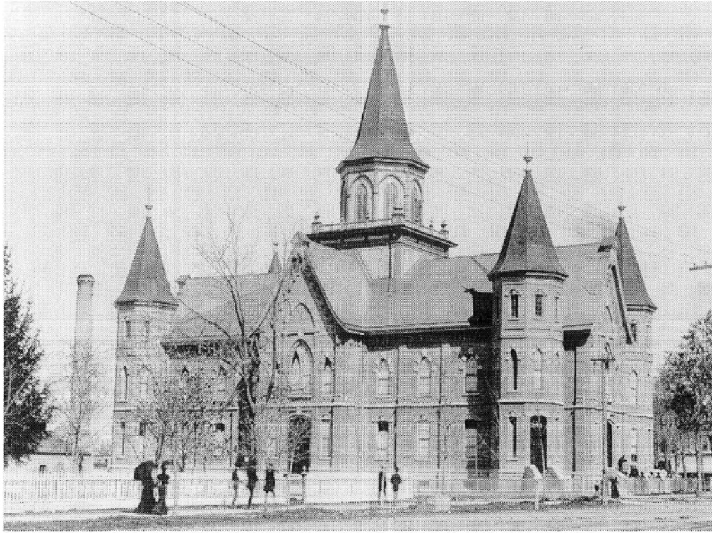
45. The New Provo Tabernacle (1883–98) before the removal of the crossing tower in 1917 for reasons of structural inadequacies. The view is from the southeast. ( Utah Historical Society )
