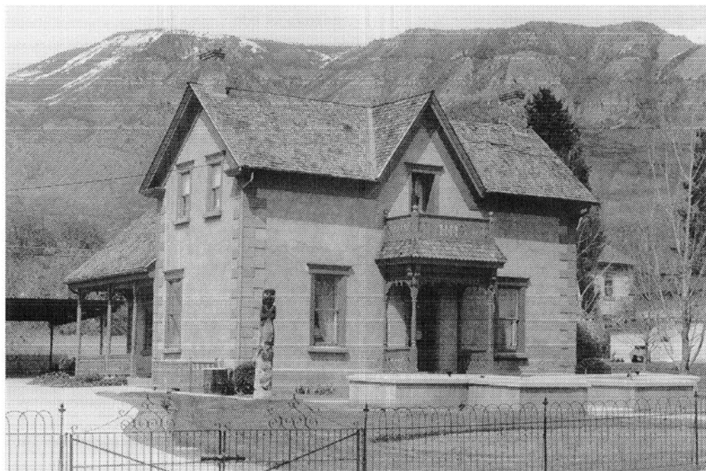
104. The Cyrus Benjamin Hawley house (c. 1869) in Pleasant Grove, Utah, seen from the southwest. The "soft rock" (tufa) rubble walls, typical of the area, were later stuccoed and scored to give the impression of ashlar construction. (Author)
