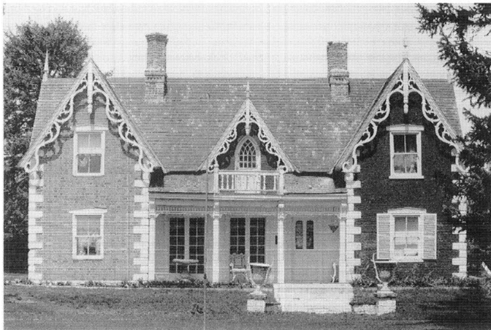
107. The John Watkins house (1869) in Midway, Utah, seen from the south. The paint has been partly removed from the brick in an effort to restore the house to its original appearance. ( Author )
