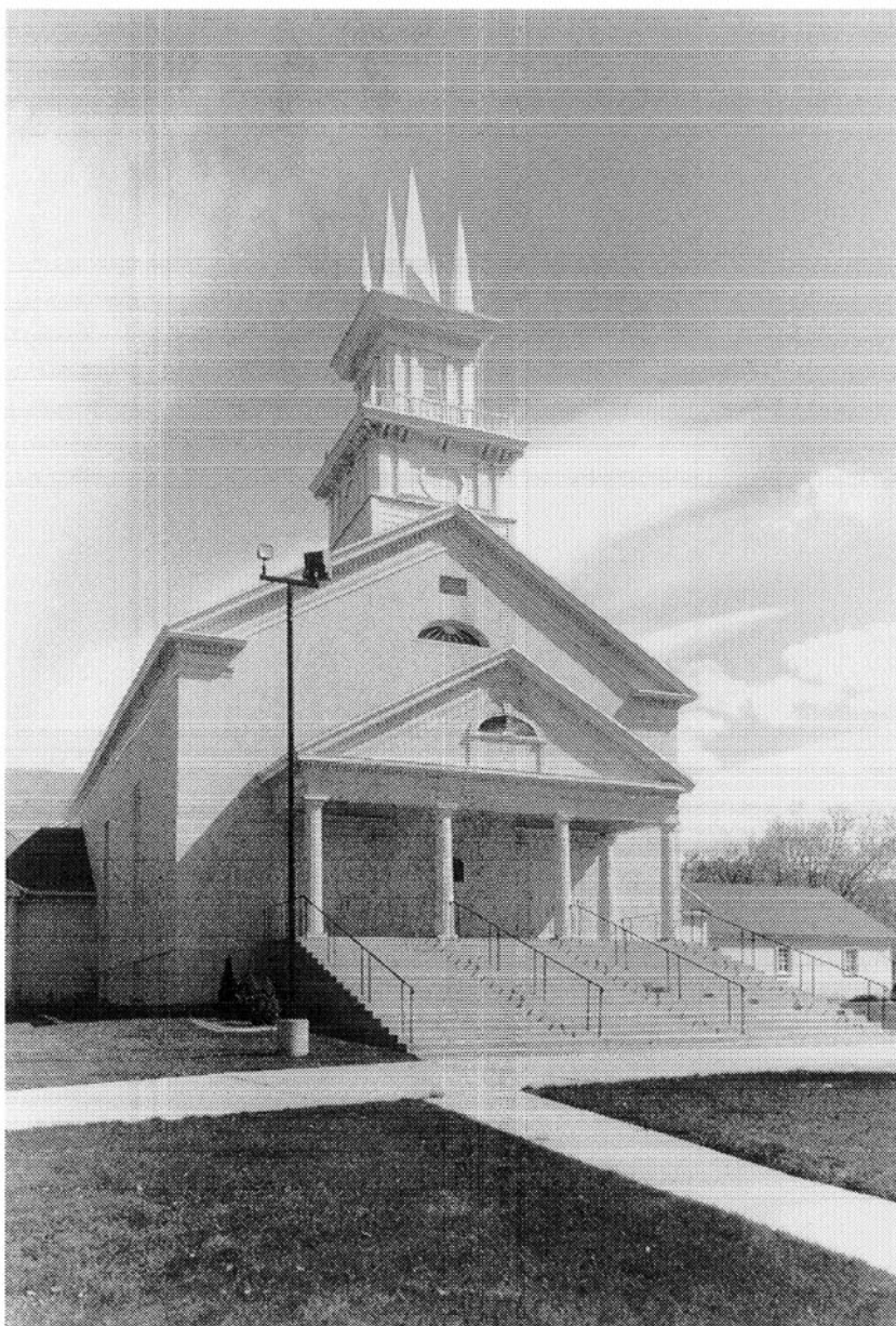
29. A contemporary view of the Bountiful Tabernacle (1857–63) from the northwest. The rostrum-choir area has undergone a number of changes, altering its original appearance. (Author)
