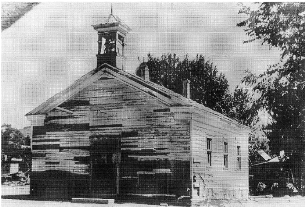
52. Adobe meetinghouse in Virgin City, Utah (1866–67) with its original clapboard siding. The clapboards were removed in the 1930s. ( LDS Historical Department )
