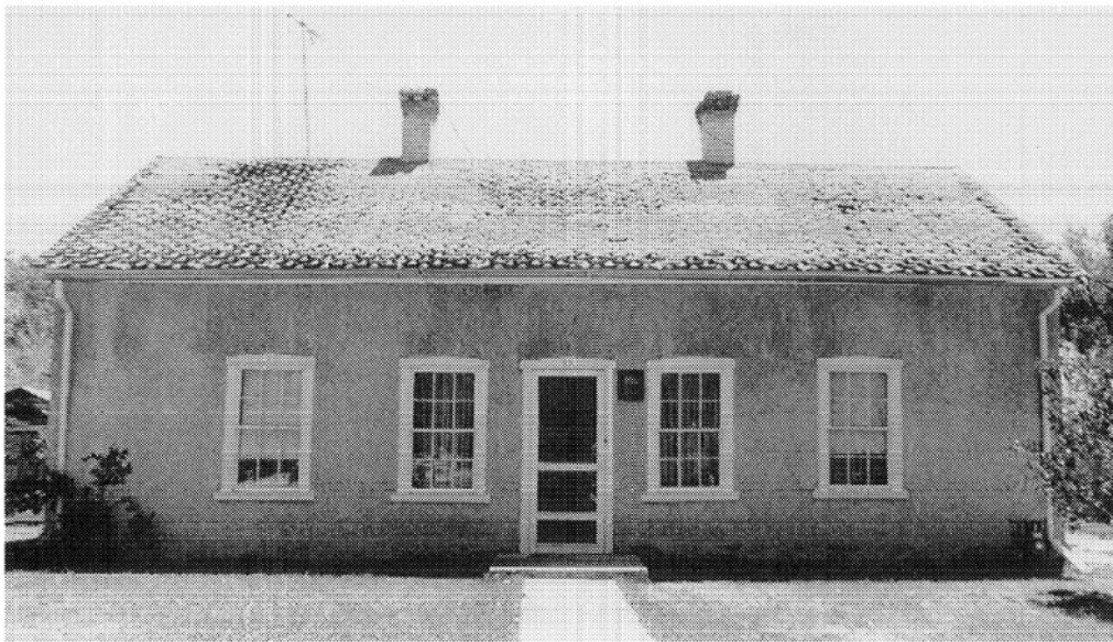
99. The Frederick Christian Sorensen house (c. 1850) in Ephraim, Utah, seen from the north. The distinctive position of the door and windows relative to disposition of the rooms is indicative of Scandinavian influence. ( Author )
