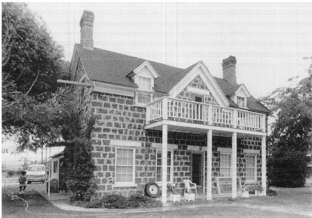
105. The Duckworth Grimshaw house (1877) in Beaver, Utah, seen from the southeast. The facade and north end are of coursed ashlar while the other walls are of rubble construction, a method common in Europe and America. (Author)
