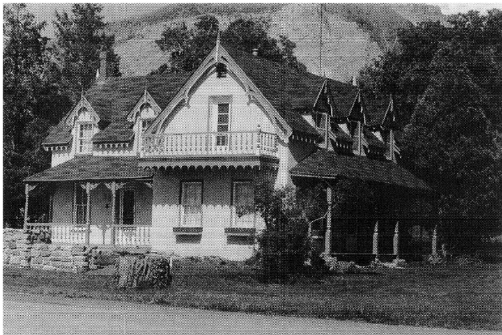
106. The John L. Edwards house (1860s) in Willard, Utah, seen from the southwest. Designs in this style and that of the Hawley House (fig. 104) became more common in the territory after 1870. ( Author )
