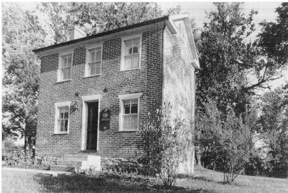
85. The George Laub house (1843) seen from the northwest. This is an extant example of a small single-room, two-story dwelling in Nauvoo. (Author)
