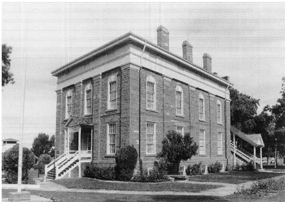
134. The completed wing of the Territorial Capitol Building (1855–56) at Fillmore, Utah. The view is from the southeast. ( Author )
