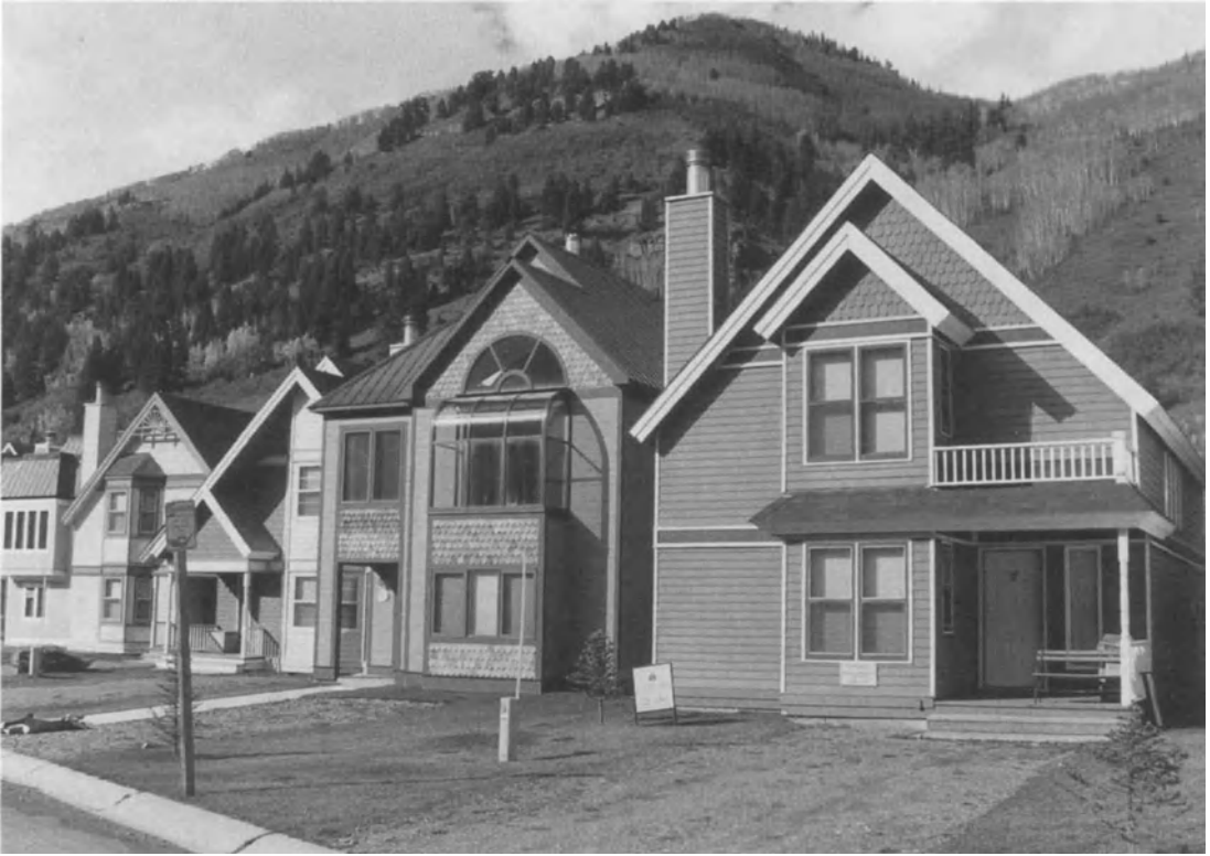
Figure 2-9. Telluride, Colo., new development outside historic area but subject to design review. (Photo: Ellen Beasley, 1986.)
