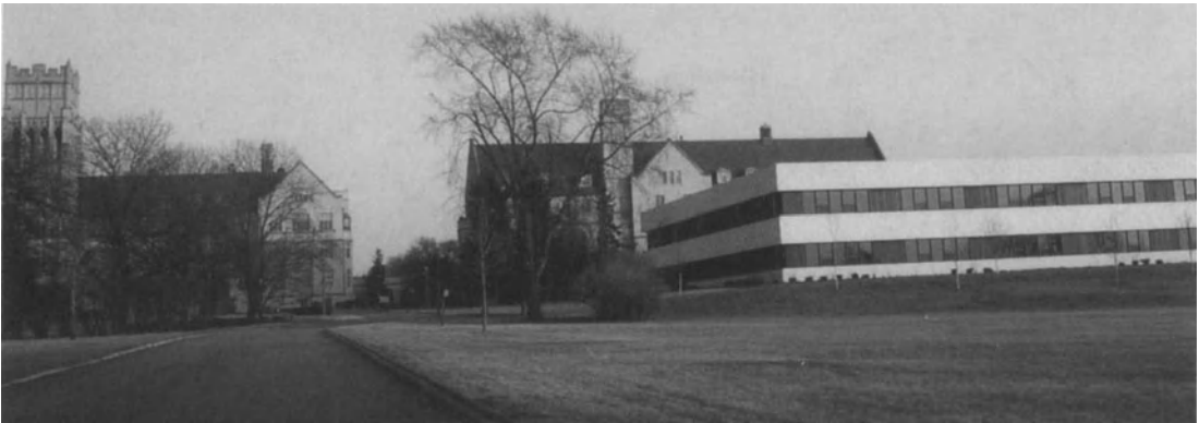
Figure 14-3. Library, Mt. Mary College, Wauwatosa, Wis.; Pfaller Herbst & Epstein, Inc. (Photo: Linda Groat.)
