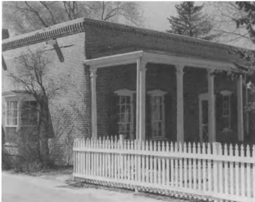
Figure 9-4. Tully House, restored Territorial style with painted brick pattern on adobe walls, 1851. (Photo: Courtesy Planning Division, City of Santa Fe.)
