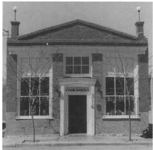
Figure 9-27. Stone warehouse, c. 1885. (Photo: Courtesy Planning Division, City of Santa Fe.)
