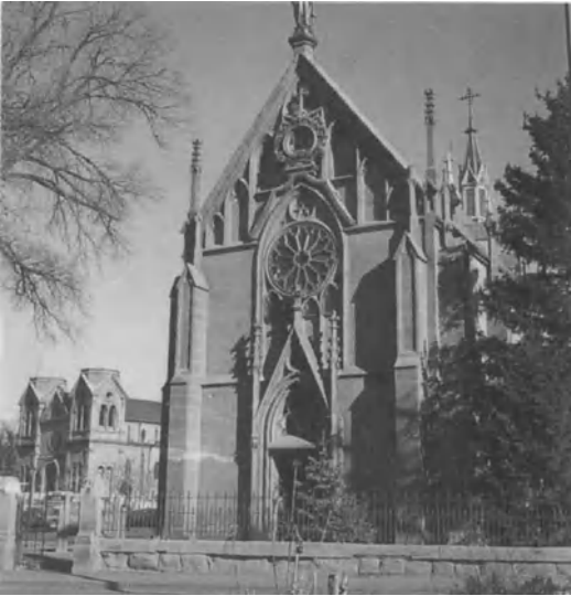
Figure 9-13. Loretto Chapel with wrought iron fence, 1878. (Photo: Conron & Lent, Architects.)
