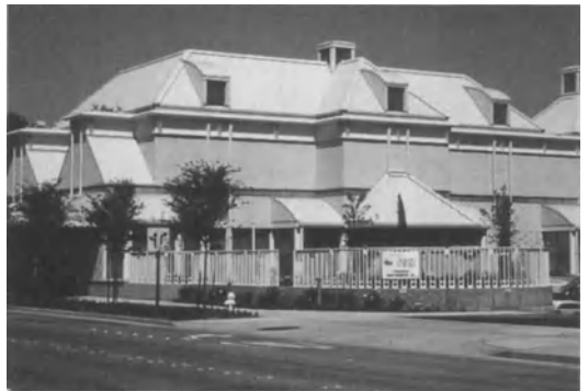
Figure 10-5. Bellevue's code offers incentives for museums, among other uses; a new, privately funded museum is being completed.
