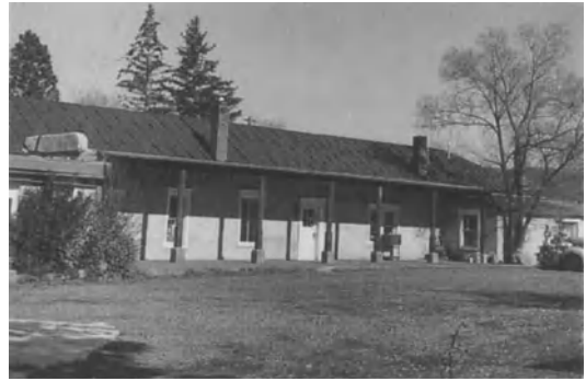
Figure 9-12. House with pitched roof on E. DeVargas Street. (Photo: Conron & Lent, Architects.)
