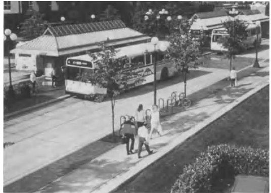
Figure 10-4. The downtown transit center contains a unisex public restroom that is monitored, with the result that it is clean and safe.
