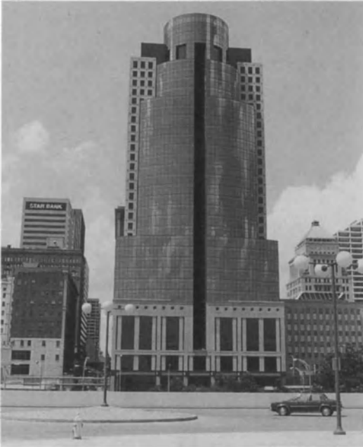
Figure 11-3. 312 Walnut Street: Third Street facade. (Photo: H. May.)
