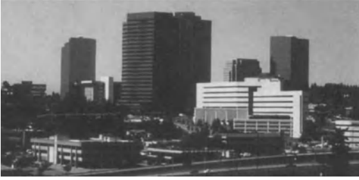
Figure 10-1. The “stair-stepped” zoning envelope has begun to fill in, with the core highly visible in the skyline.
