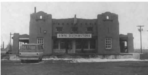
Figure 9-26. Gross, Kelly Warehouse, Rapp & Rapp, Architects, 1914. (Photo: Conron & Lent, Architects.)
