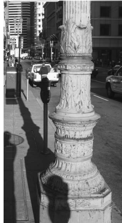
6.32 Ornamental bases for street light poles come in many styles. This one has acquired a distressed patina. Photo credit: Bill Main
