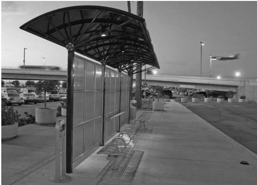
3.15 A remote parking area at Los Angeles International Airport provides light, airy shelters with benches and off-the-grid solar lighting for the comfort and safety of travelers waiting for shuttles to the terminal. Photo credit: copyright © Jim Powell
