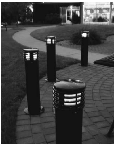
6.19 Bollards with solar LED lighting perform multiple functions. Photo credit: copyright Jim Powell
