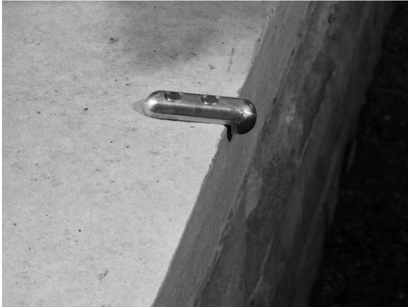
9.3 Skateboarding deterrence: Stainless steel elements added to a stone seat wall are small, simple, and discreet. Photo credit: Bill Main
