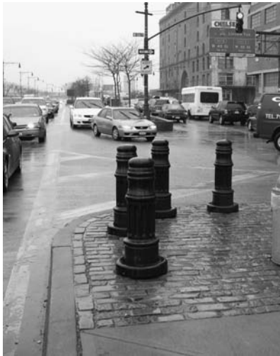
6.18 Bollards protect a pedestrian crossway at a median. Photo credit: Bill Main
