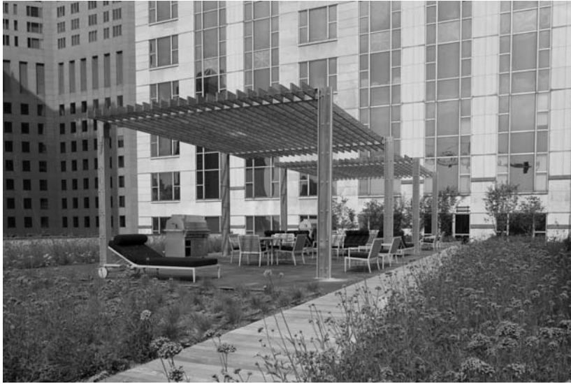
3.21 A roof garden designed by Hoerr Schaudt located on Michigan Avenue in Chicago,. Photo credit: copyright © Scott Shigley
