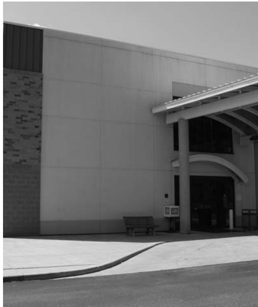
2.26 A lonely bench placed against a monumental wall is dwarfed in scale. Who would happily sit in this inhospitable space? Photo credit: Bill Main
