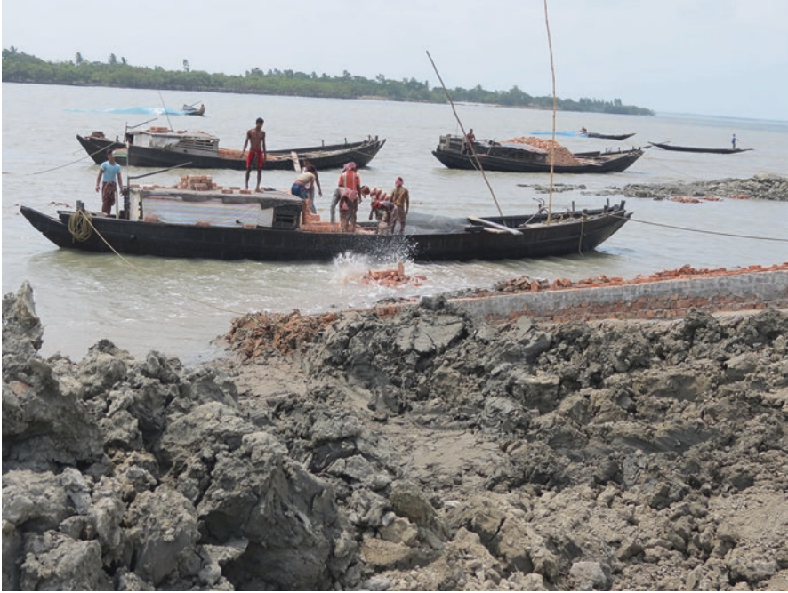
Photo 5.10 Bricks being unloaded for construction of embankments in Khulna, Sandeshkhali II, June 2015, © Aditya Ghosh
