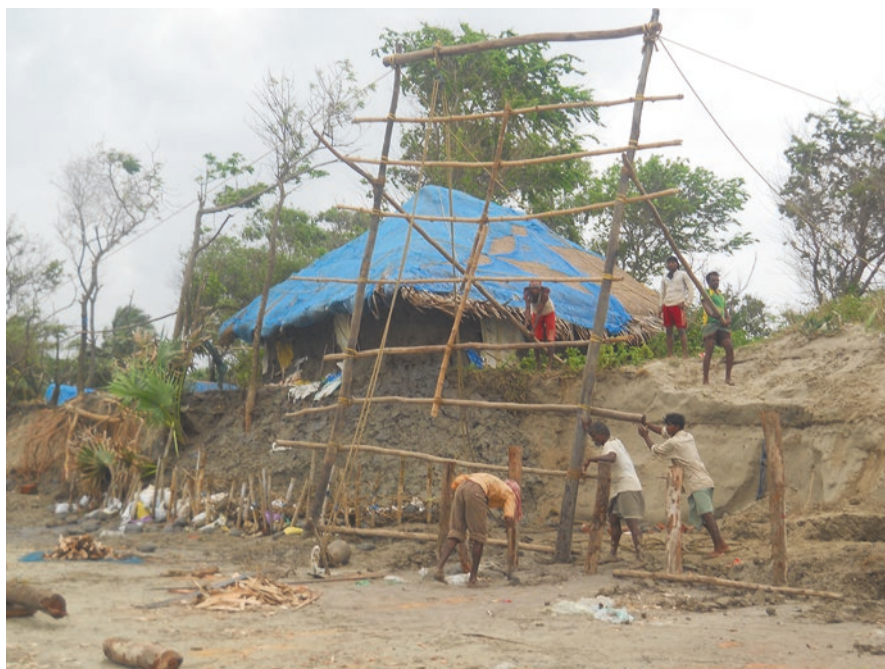
Photo 5.11 Futile defence? Temporary embankments being erected at Baliara, Mousuni, January 2012, © Aditya Ghosh
