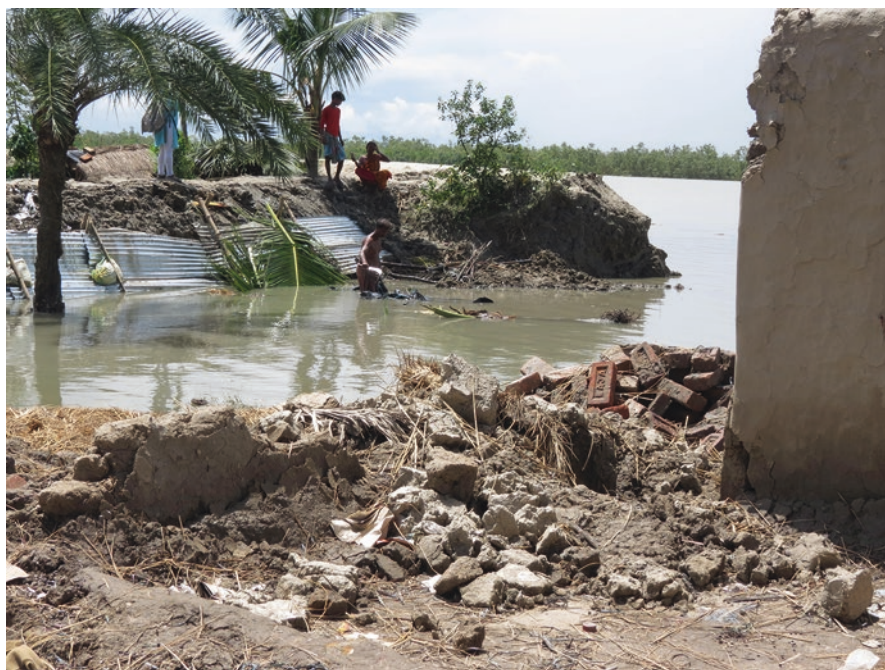
Photo 4.3 Tidal bore damages in Pakhirala, Gosaba. Scampering to rebuild their households and save whatever little is left of the house (on the right). September 2014 © Aditya Ghosh
