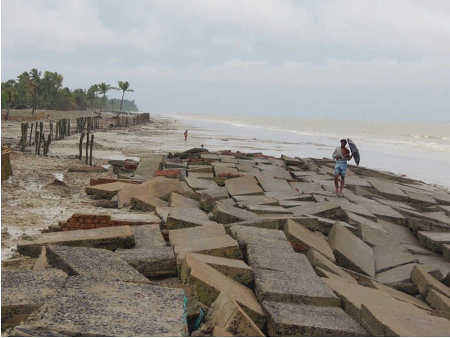
Photo 5.6 Destroyed concrete embankment in Baliara village, Mousuni Island. Locals however blame implementation rather than its ability to contain the tides. August 2014 © Aditya Ghosh
