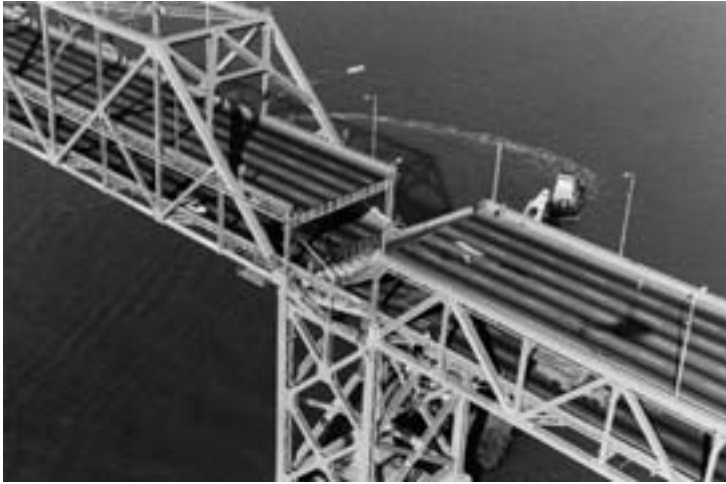
Figure 12.3 Collapse of Bay Bridge's east span, Loma Prieta Earthquake, 1989
