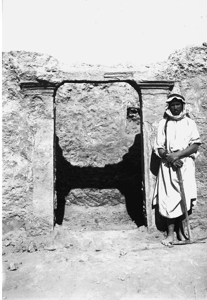
FIGURE 2.20 Image of doorway, B8-H3. YUAG c57.
