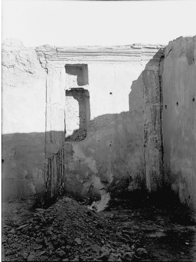
FIGURE 2.23 Niches in blocked door on east side of room C7-G3. Note also empty sockets in wall to right of door. YUAG H41a.
