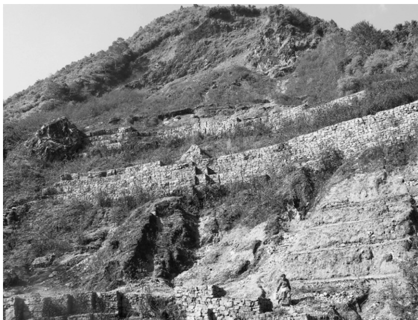
Figure 1. View of the research site at a landslide near Thankot in the Middle Mountains of Nepal at the beginning of construction works in December 2001.
