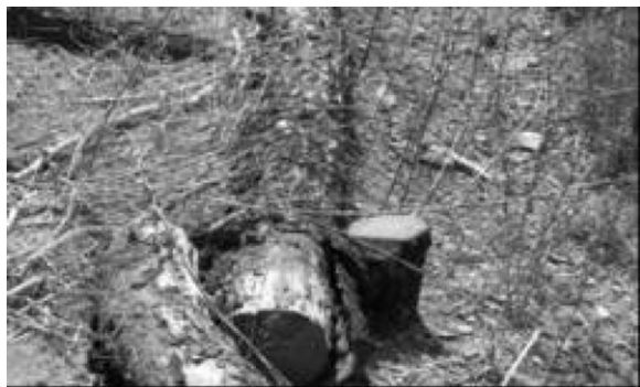
Figure 6. Log erosion barrier after 5–6 years of operation.
