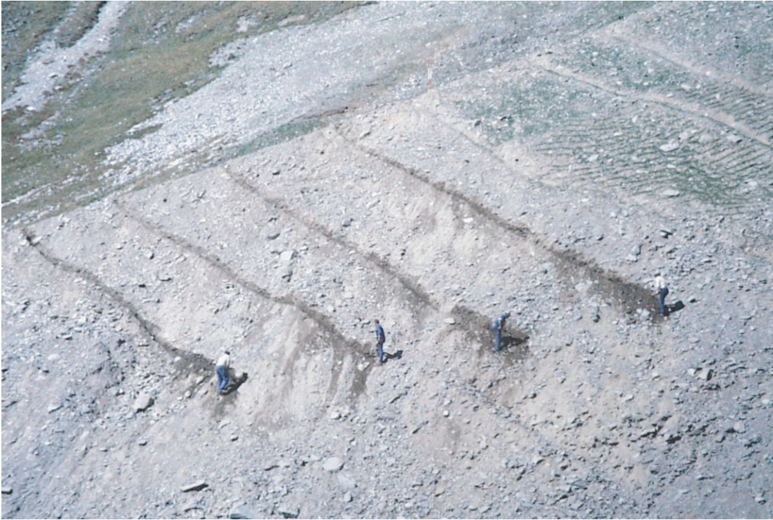
Figure 6. To prevent surface erosion, small ditches (furrows) are dug by hand, running diagonally across the slope.
