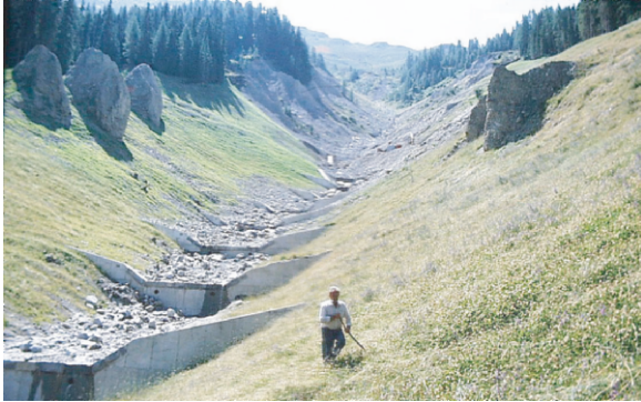
Figure 8. Middle reach of a torrent in 1993 after scarping, degrading and revegetating the slopes, using the method of Huter and Heumader (1981) (same site as in Figure 7).
