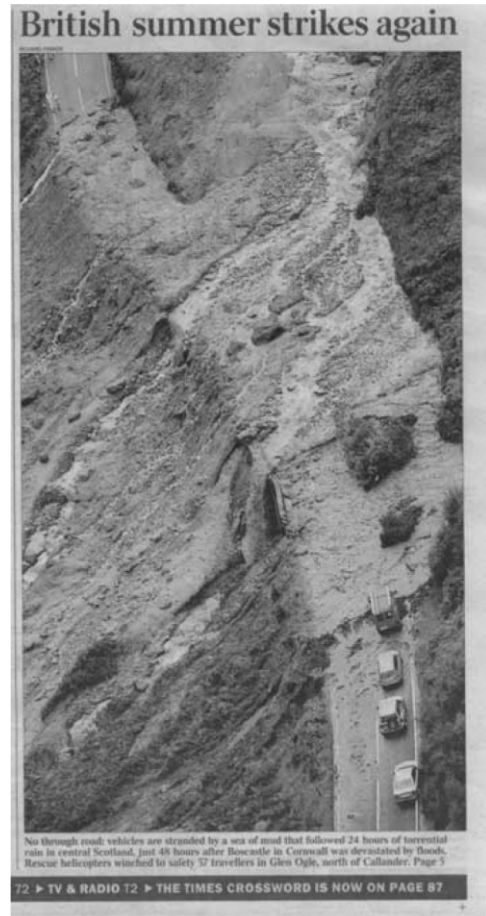
Figure 2. Shallow landslide problems blocking roads and trapping motorists in Scotland, after heavy rains in August 2004 (Times Newspapers).
