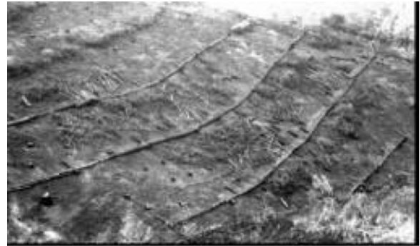
Figure 4. Log erosion barriers across the contours.
