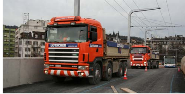
Fig. 12: The three test vehicles crossing the bridge in line in the right lane direction Tribtschen.
