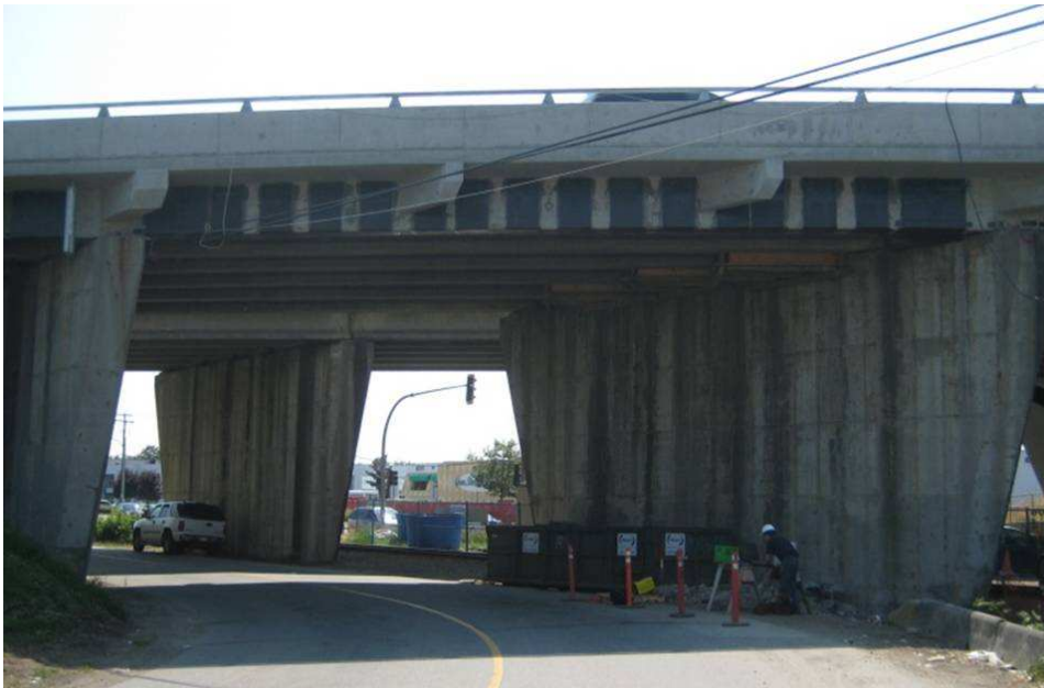
Figure 5: Installed CFRP strips and composite wrap
