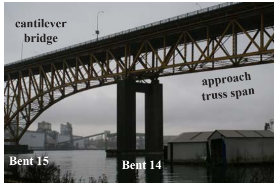
b) Bent 14: south end of the approach truss spans
