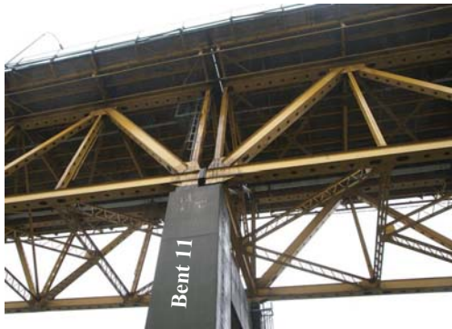
a) Deck floor and steel warren trusses
