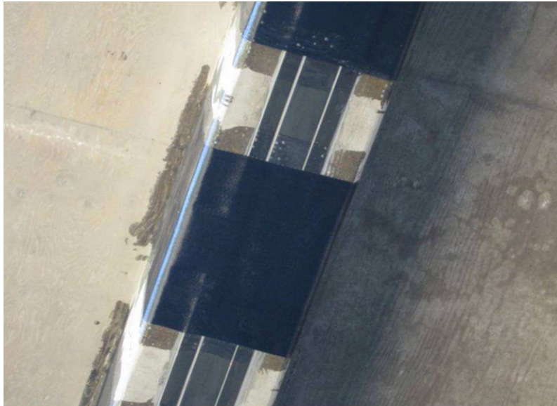
Figure 4: Seismic reinforcement project
