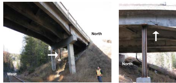
Figure 2 Temporary support at Goat Fell bridge
