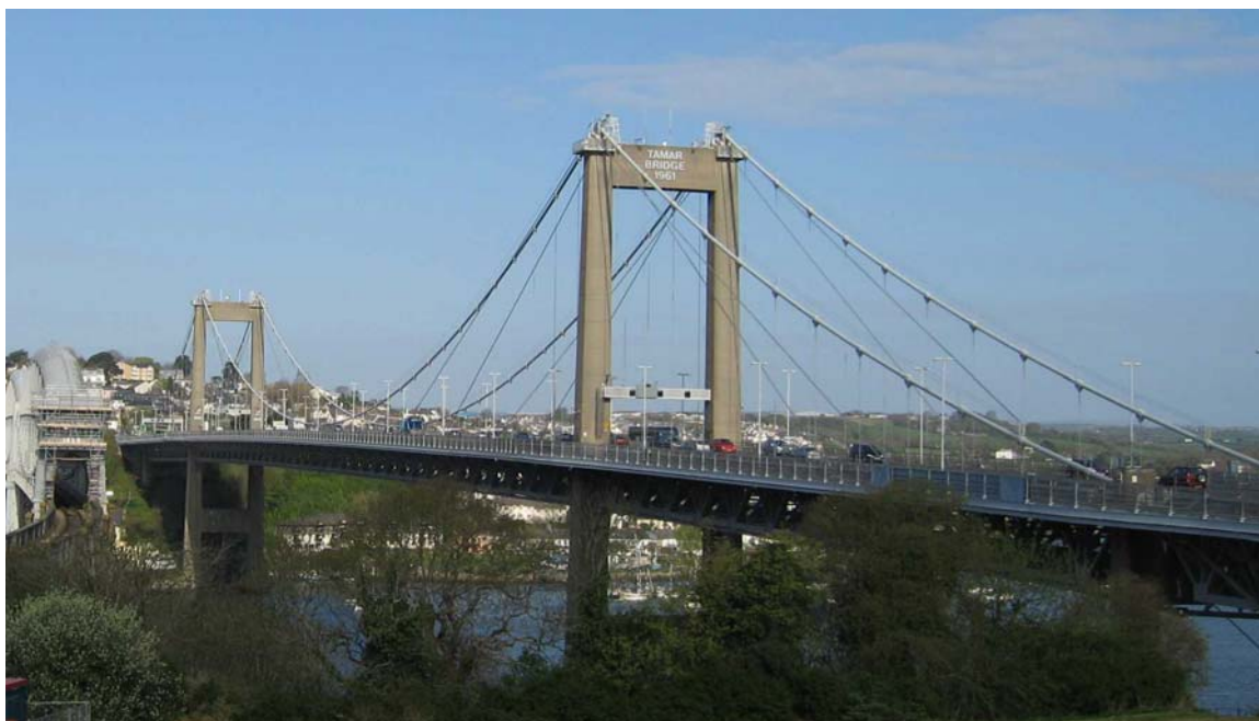
Figure 1. The Tamar Suspension Bridge, Plymouth, UK.
