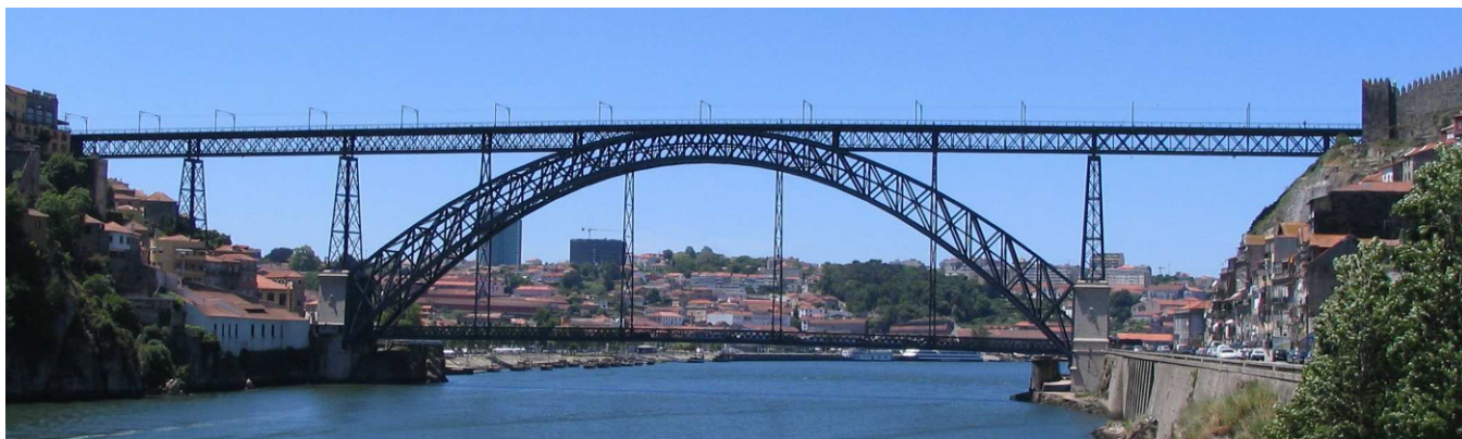
Figure 4: General view of the Luiz I Bridge.
