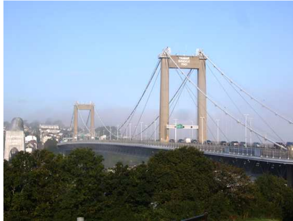
Figure 1: Photograph of the Tamar Suspension Bridge, Plymouth, UK
