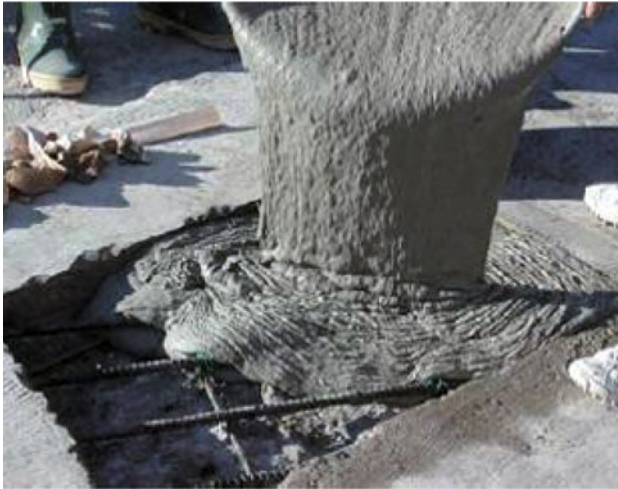
Fig. 7.4 Self-consolidating casting of SHCC patch (ECC Technology Network, 2009).
