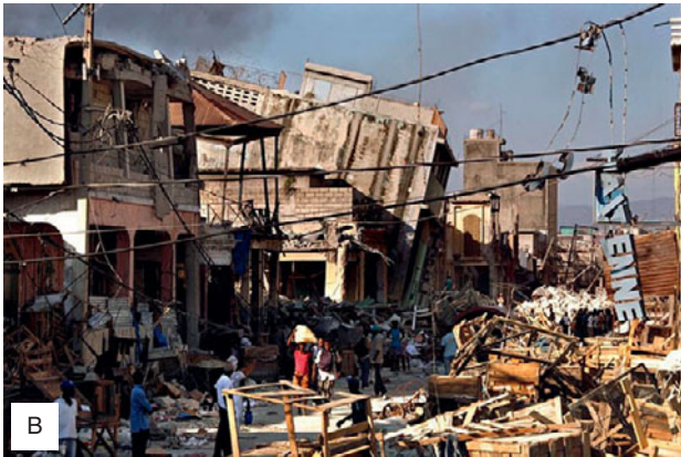
Figure 11.1 Haiti earthquake disaster in 2010.
