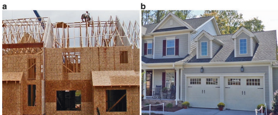
Fig. 6.11 (a) Web-like structural roof trusses effectively eliminate the use of dormers in the space within the roofline. (b) Rooms with dormer windows over the garage are a popular concept, as here roof rafters or specialty trusses are required only on one smaller section of the house and add to the appeal of the elevation
