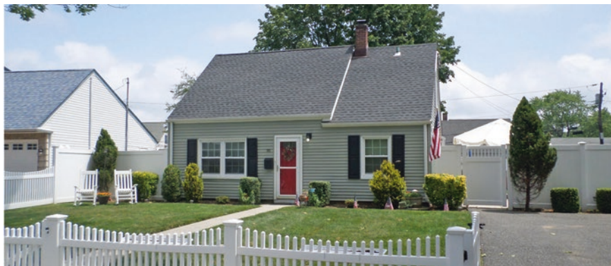
Fig. 1.18 This house in Levittown, NY was one of six basic models used for a community of 17,447 households. The selection of the Cape Cod style reinforces the style's enduring appeal and frugal qualities
