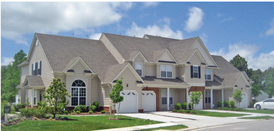
Fig. 8.11 Incorporating attached garages into multifamily buildings is a challenging design task. Garages should be recessed into the façade, as was done at Belmont in Suffolk, VA built by Chesapeake Homes
