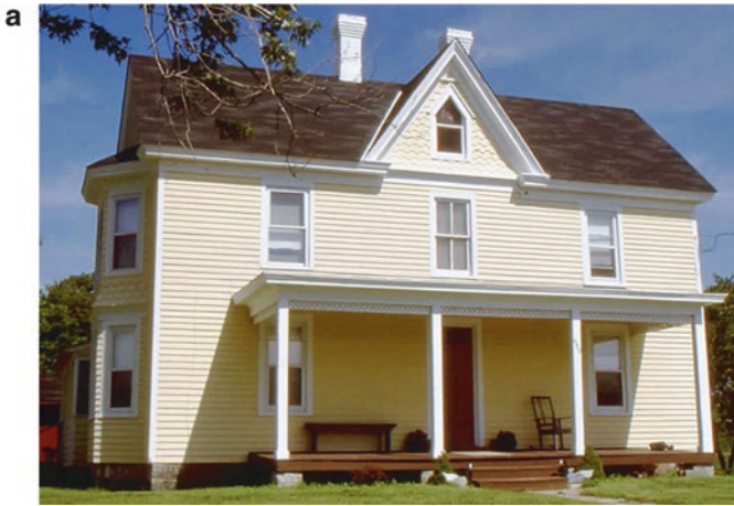
Fig. 5.17 (a) The narrow spans of the American Gothic farmhouse were an inspiration for this model house at Eirean Mohr in Salisbury, MD. (b) The floor plan had modules that were only 14’–16’ wide and had a two-story element facing the street with a one-story element in back. This is the very same practical-yet-livable floor plan of many historic farmhouses
