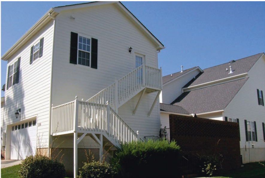
Fig. 4.17 The New Neighborhood in Old Davidson , in Davidson, NC, had accessory units above garages
