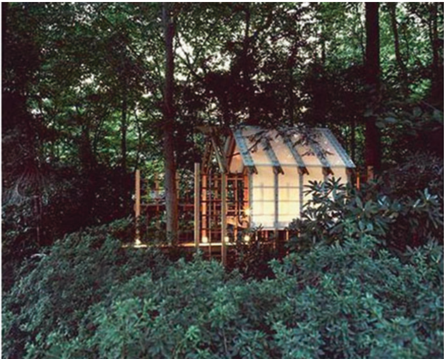
Fig. 4.37 This rear yard playhouse by Glen + Williams Architects won a national AIA Honor Award. (Courtesy J. Lee Glen and Roxanne Williams, formerly Glenn + Williams Architects)
