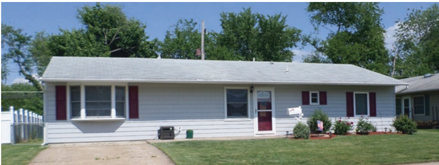
Fig. 9.2 Modular or manufactured housing is generally weak in design: low-pitched roofs, random window and door placements, box-like exteriors, and poor detailing are common problems in the industry
