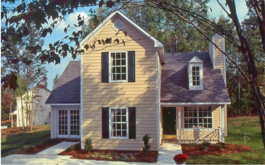
Fig. 7.6 This very affordable entry-level model house in Durham, NC incorporates a dormer on top of a vaulted truss roof. The narrow dormer here acts as a skylight into the living room below
