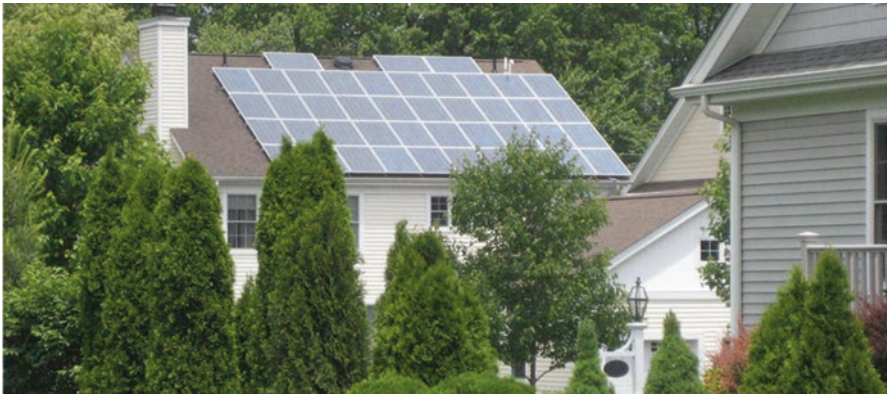
Fig. 10.1 Photovoltaic solar panels that provide electric power are more frequently seen on the roofs of newer homes and communities as housing consumers seek lower utility bills and clean energy
