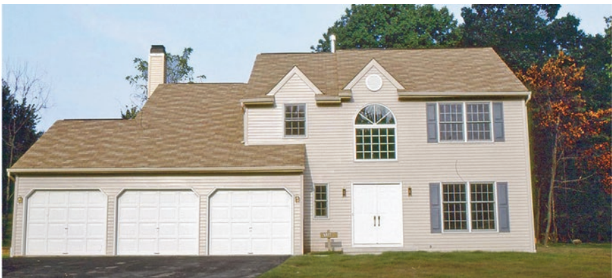
Fig. 7.1 The exterior design of production houses suffered tremendous deterioration in the post-war years
