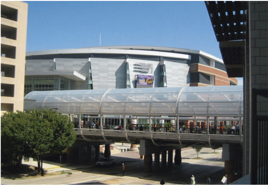
Fig. 10.15 This light rail station in Charlotte, NC connects the downtown to suburban communities, thereby relieving traffic congestion and reducing carbon emissions from automobile usage
