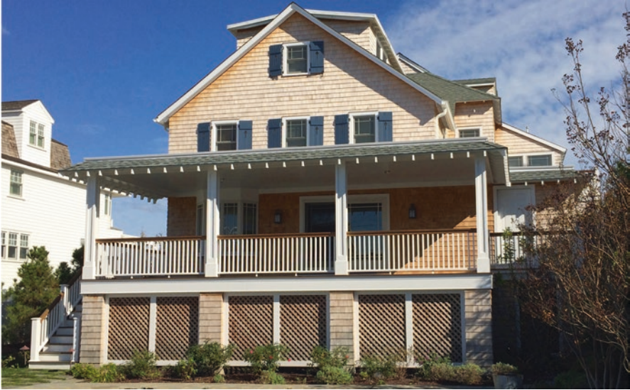
Fig. 10.9 Resilient design anticipates how periodic forces of nature can damage or destroy homes. For protection from flooding, homes are to be raised above government-mapped minimum floor elevations
