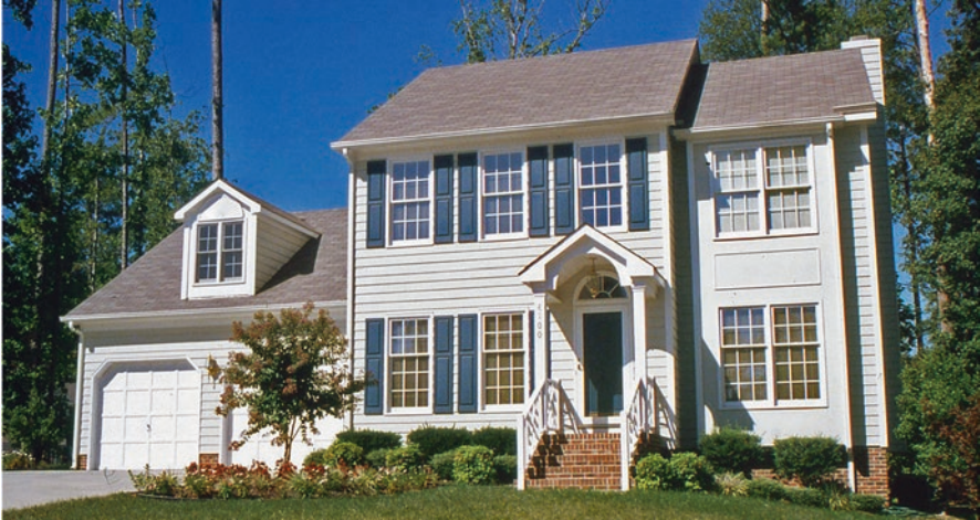
Fig. 5.8 This modest house in Durham, NC is organized as three modules, with each module's rooflines, window and door placements further reinforcing the façade's organization
