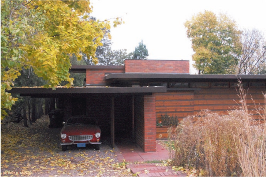
Fig. 1.15 The Usonian style developed by Frank Lloyd Wright is seen in his design for the Jacobs First House in Madison, WI, built in 1937. Elements of the Usonian style are found today in contemporary ranch houses nationwide. (Photography courtesy Rick McNeese)
