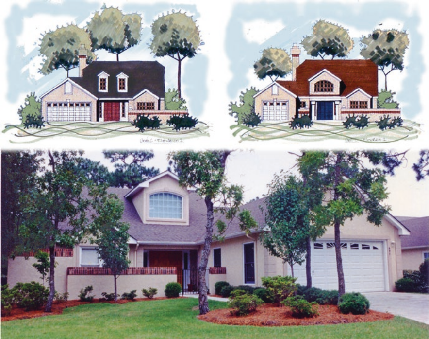
Fig. 4.34 Privacy walls at Providence Park in Myrtle Beach, SC were integrated directly into the exterior walls of houses, with consistent materials and colors. Wall in front yards could be no higher than 3 ft, while side walls were 6 ft high. A brick cap, stucco finish, and plantings helped to soften the wall's appearance
