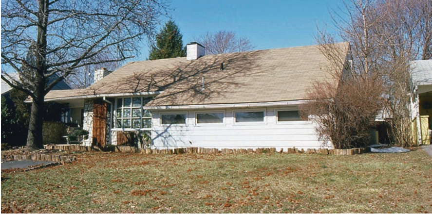
Fig. 2.3 In the postwar era, houses were stripped of frills such as covered porches, articulated floor plans, and other details. The goal was to build to the maximum square footage at minimum cost per square foot
