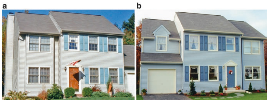
Fig. 7.16 (a) The inclusion of muntins in windows helps to develop human scale in the façade. (b) One problem with “snap-in” muntins is that some residents remove them, making some houses look unfinished when viewed from the street
