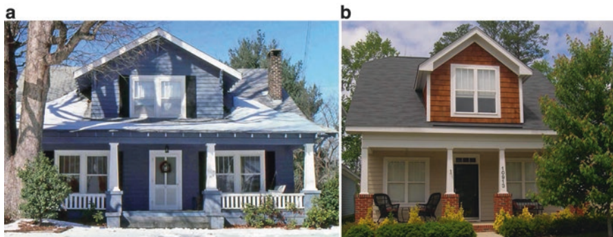
Fig. 1.13 (a) The Craftsman style, found in this 1920s house in Greensboro, NC, is still popular today. We see this style emulated in an entry-level design at Falls River in Raleigh, NC (b)
