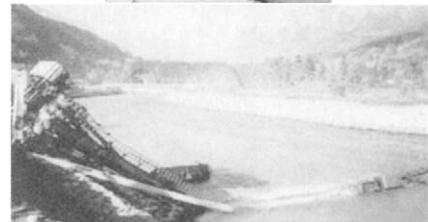
Figure 1.7 Collapsed pile driver: After Schaden Spiegel 2/96
