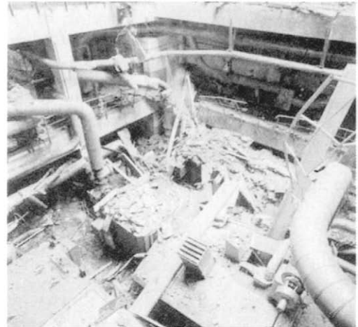
Figure 1.6 Burst high pressure preheater and devastated plant room: After Schaden Spiegel 1/82
