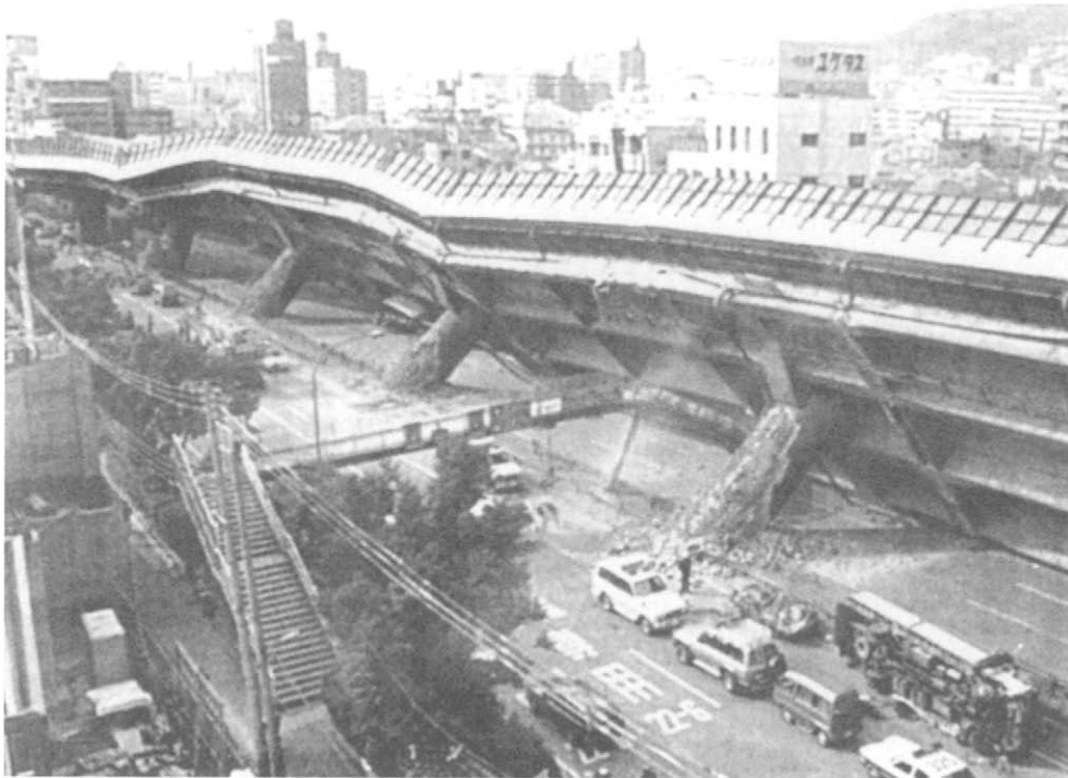
Figure 1.4 Collapsed Kobe-Osaka highway
