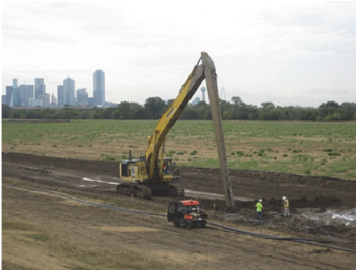
Photograph 1. East Levee SB cutoff wall construction, heading 1 PC 1250.
