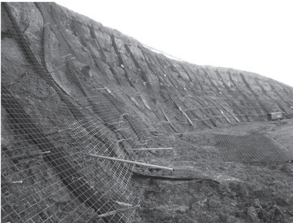
Photograph 3. Horizontal Drain Placement
