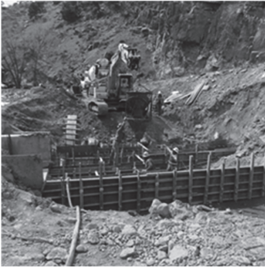
Photograph 3. Foundation Cutoff for the Dam
