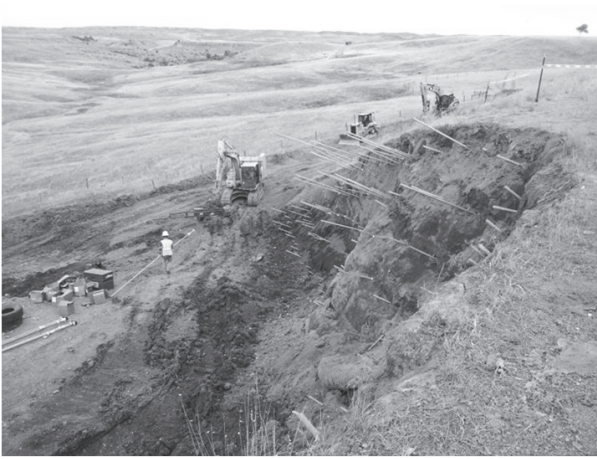
Photograph 2. Launched Nail Installation
