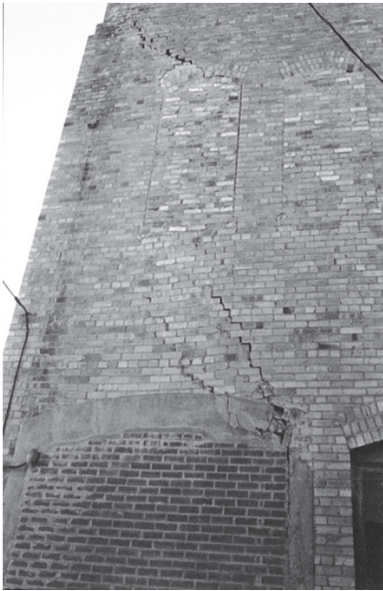
Photograph 2. Photographs of damaged structures resulting from collapsible soils (Image Source: White 2008)
