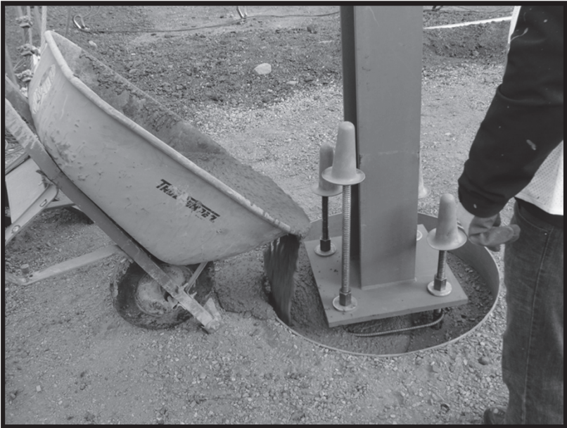
Photograph 12. Pouring the concrete foundation pad around the grouted bar elements.
