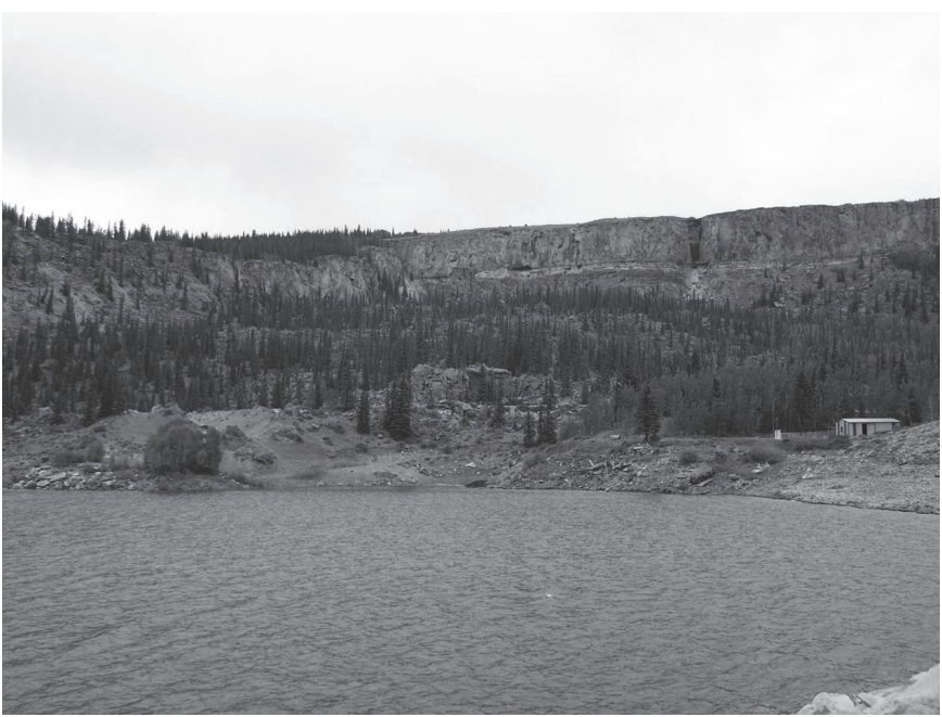
Photograph 5. Left Abutment Rock Slide Deposits (Note tuff cliffs that mark slide scarp)
