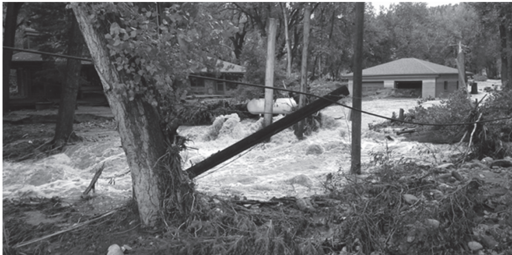
Photograph 2. Damage on Lower Left Hand Creek
