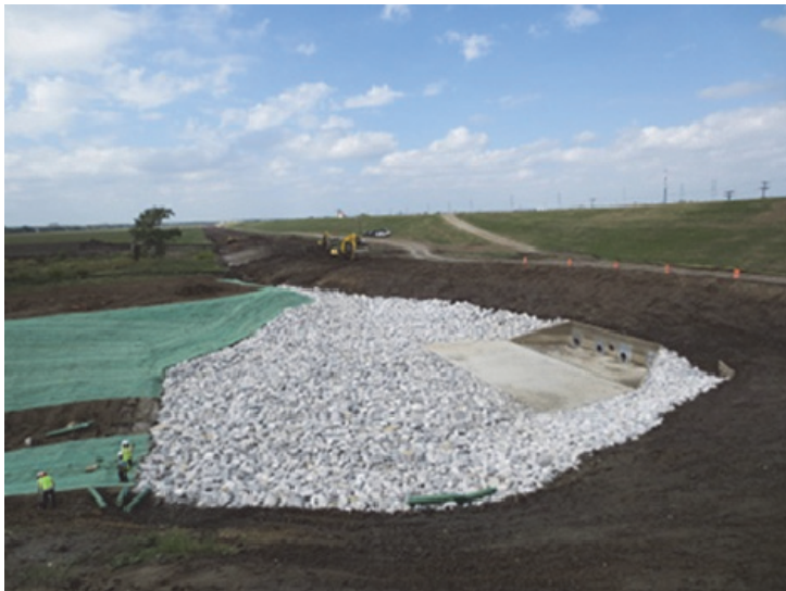
Photograph 3. East Levee Old Hampton Outfall.
