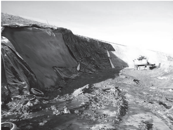
Photograph 5. Removing Shotcrete Blankets
