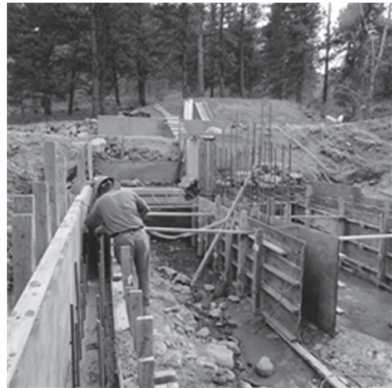
Photograph 4. Diversion Dam Reconstruction
