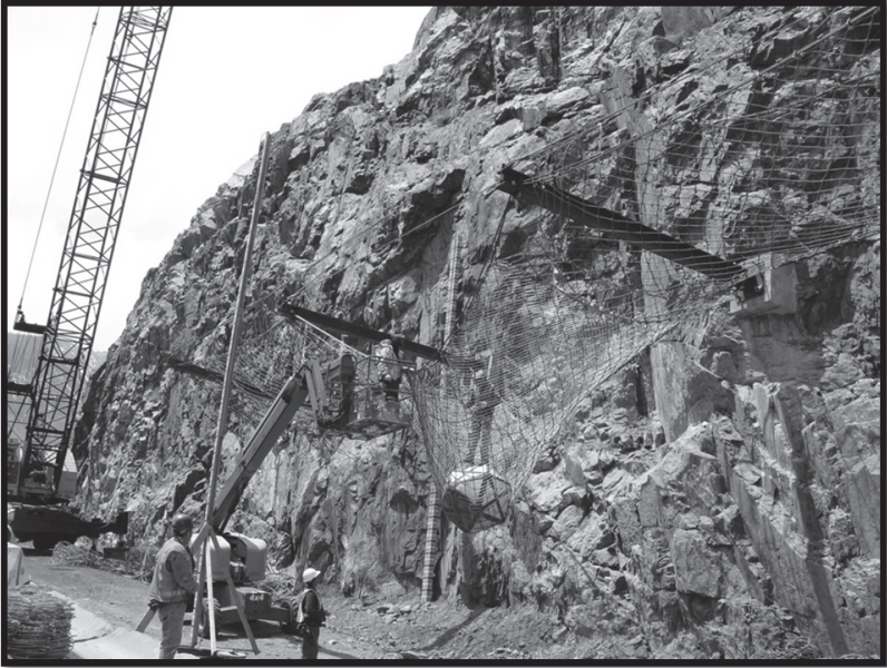
Photograph 6. Side View of Actual Post and Barrier Test System for Four Posts for Test L – 911 kJ test.
