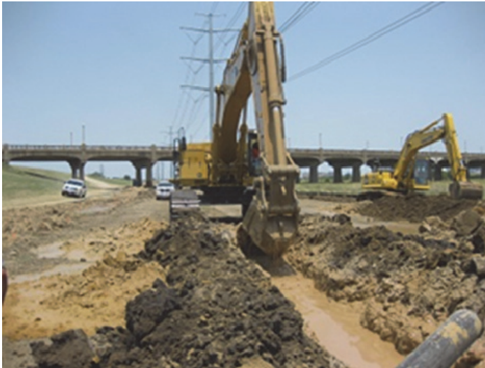
Photograph 4. West Levee SB cutoff wall construction.
