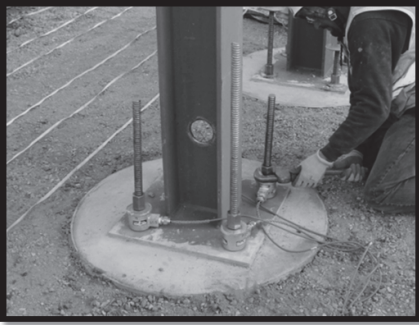
Photograph 10. Location and tightening of load cells prior to testing.
