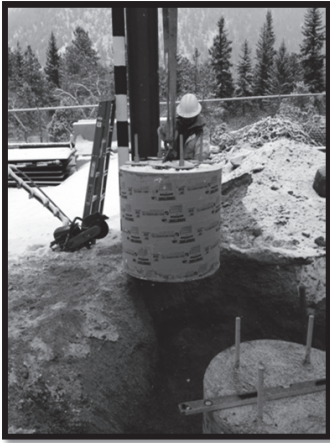
Photograph 13. Installation of circular concrete shaft post foundation systems with completed system compacted in place.
