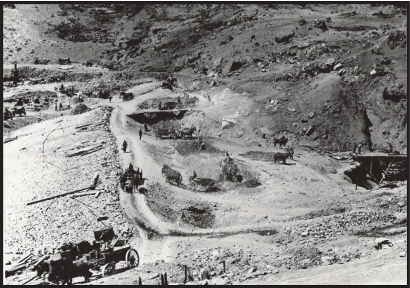
Photograph 2. Earthfill construction, June 2, 1912
