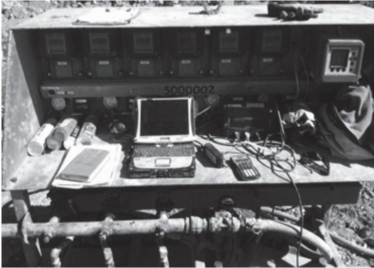
Photograph 7. Grout Field Setup
