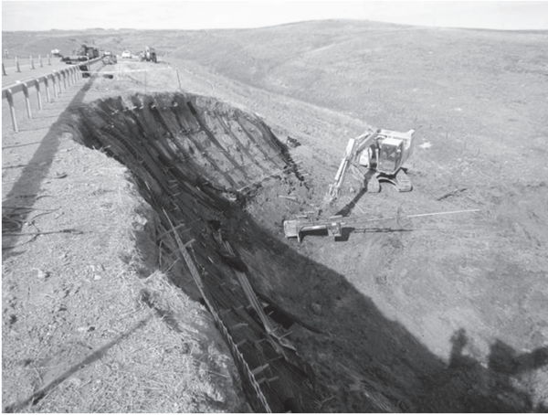
Photograph 4. Final row installation
