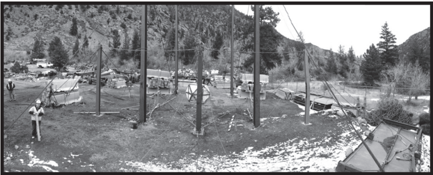
Photograph 9. Front view of the test site setup. Rock is directly behind test post prior to raising it.
