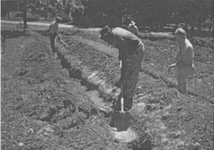
Figure 9-1. Excavation of the Peyton Randolph site in 1955, archaeologist James Knight shown (far right). Photograph courtesy of the Colonial Williamsburg Foundation.
