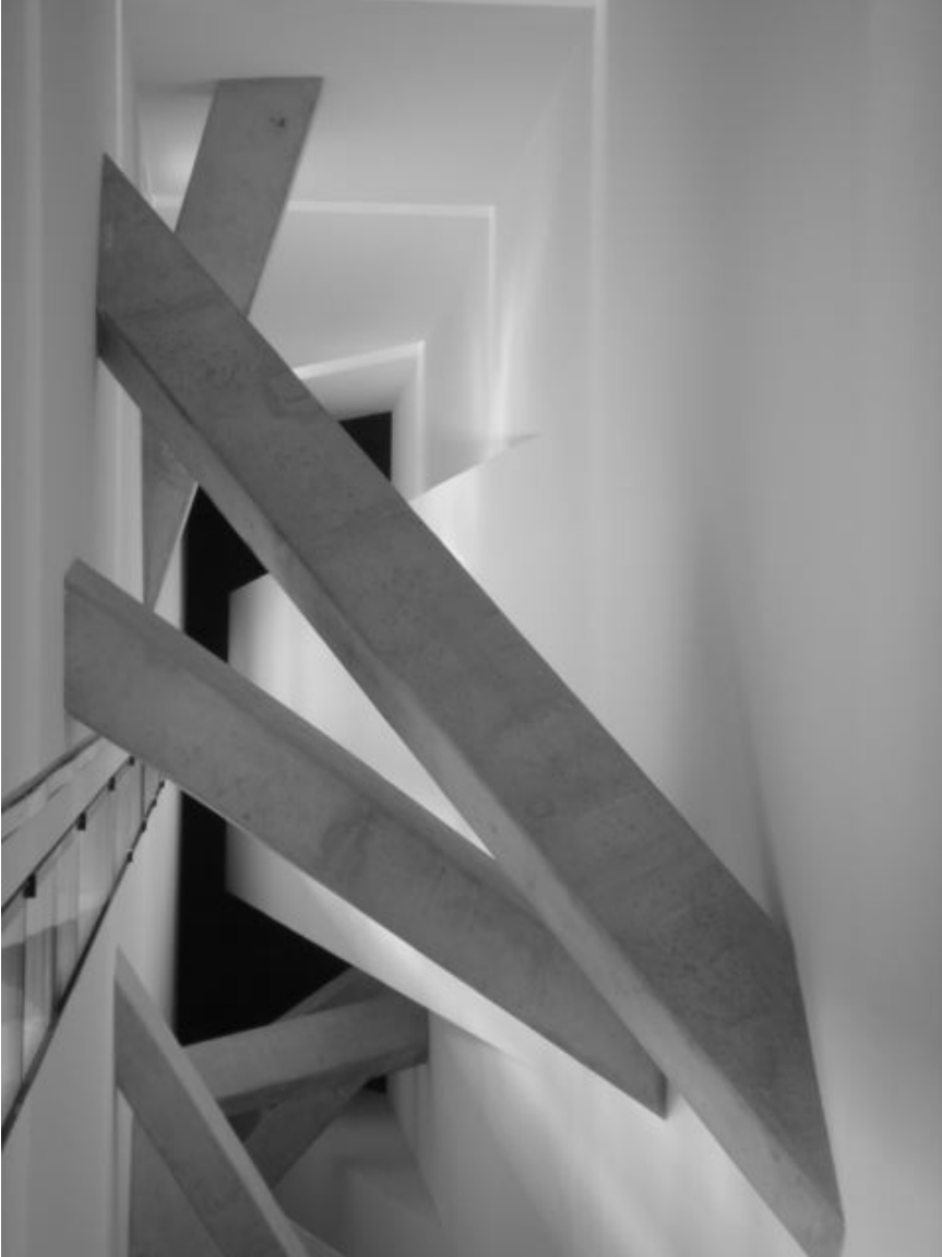
Figure 8-5. Interior, view of concrete beams above stair. Photographed by Frank H. Weiner.
