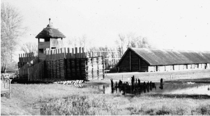
FIGURE 9. Bronze Age and Early Iron Age enclosed settlement on the lake at Biskupin in central Poland. Original remains of wooden construction and its reconstruction. Phot. Ł. Kobyliński.
