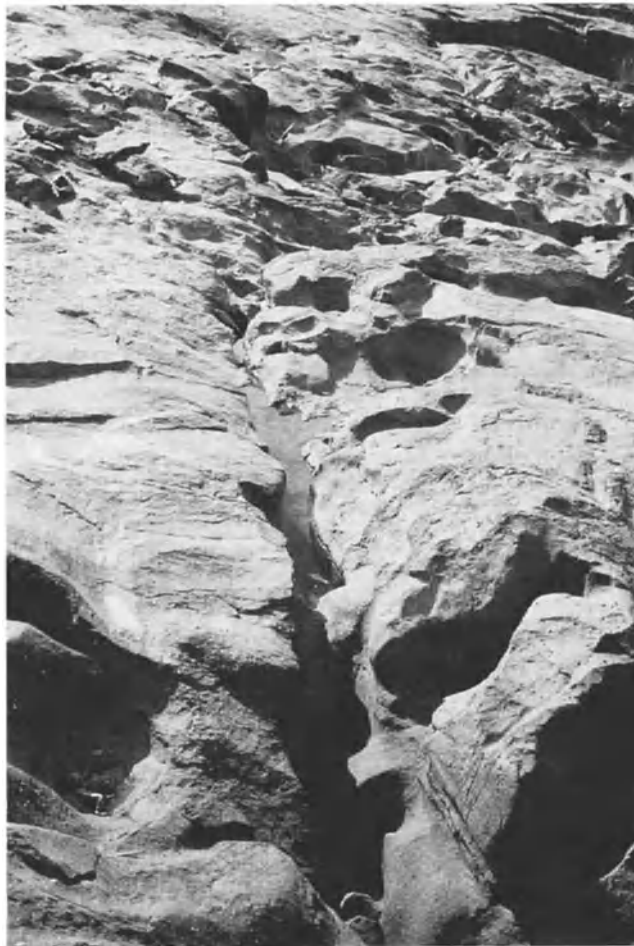
Figure 10. Control of potholes and grooves by a joint normal to flow direction, Tapi River, India.
