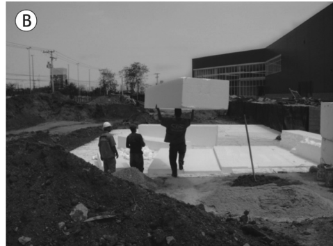
Figure 1.6 Use of EPS on embankments on soft soils: (A) cross section of an embankment built with EPS; (B) detail of the construction of an EPS embankment (Lima and Almeida, 2009).
