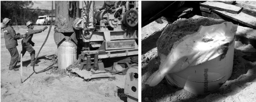
Figure 7.24 Execution details of encased columns.
