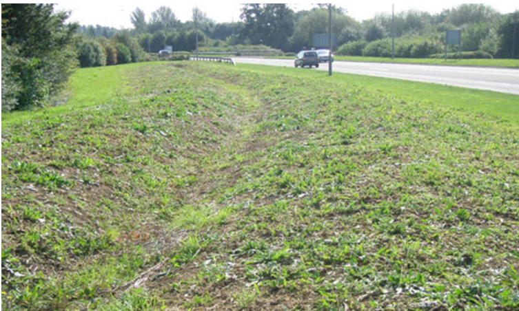
Fig. 7.5 A dry swale alongside a major road in Milton Keynes
