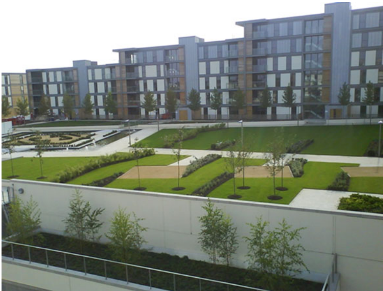
Fig. 7.2 An intensive green roof on top of a hypermarket in Milton Keynes
