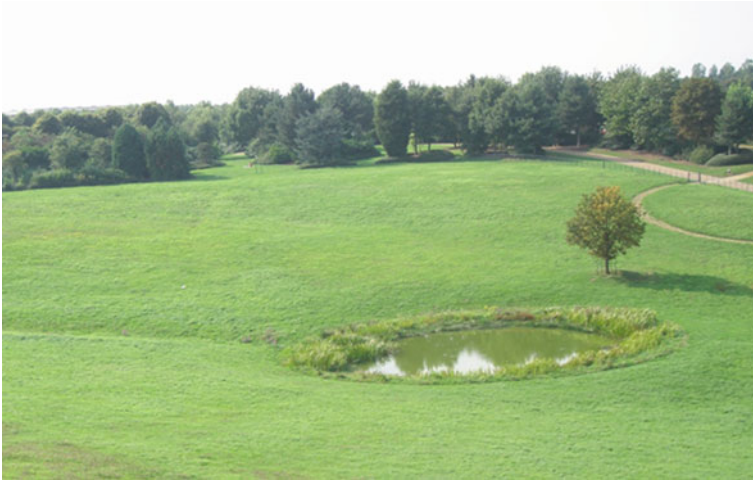
Fig. 7.4 Filter stripes, a swale and a retention pond at Campbell Park, Milton Keynes
