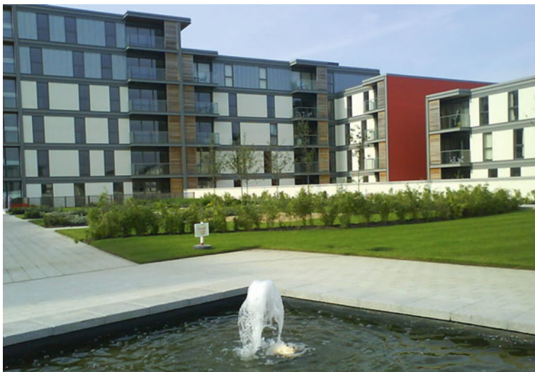
Fig. 7.3 Previous paving in a housing development in Milton Keynes
