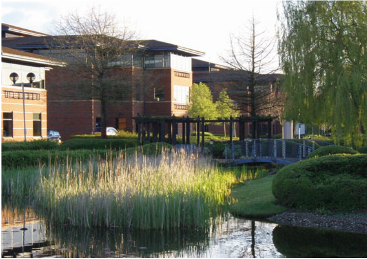
Fig. 7.11 SUDS and water features at Caldecotte Business Park
