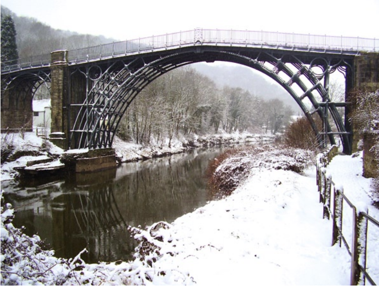
Fig. 3.5 The iron bridge (Shropshire). (Photo: Paul Belford)
