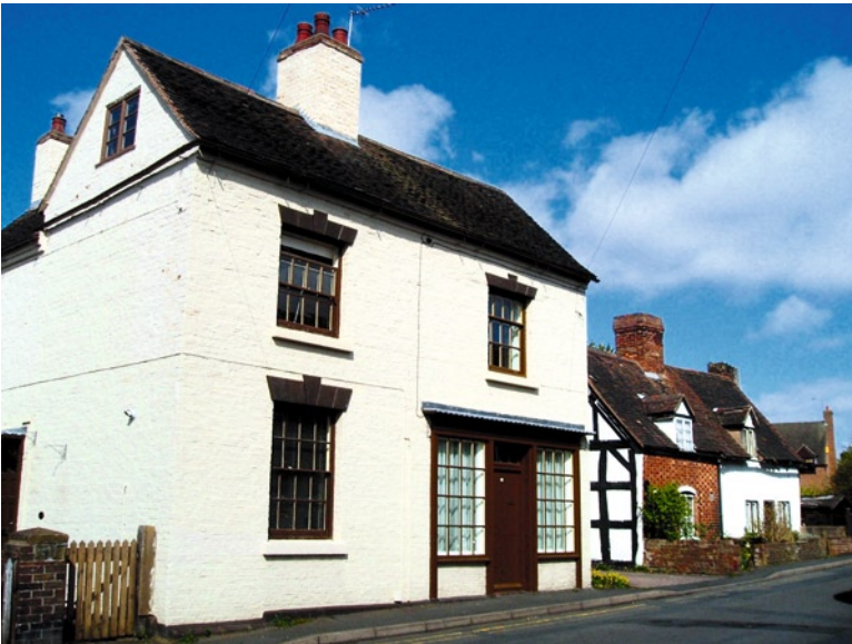
Fig. 4.2 Listed buildings range from large palaces and castles to smaller and more humble dwellings, such as these 17th to 19th century cottages and former pub. (Photo: Paul Belford)
