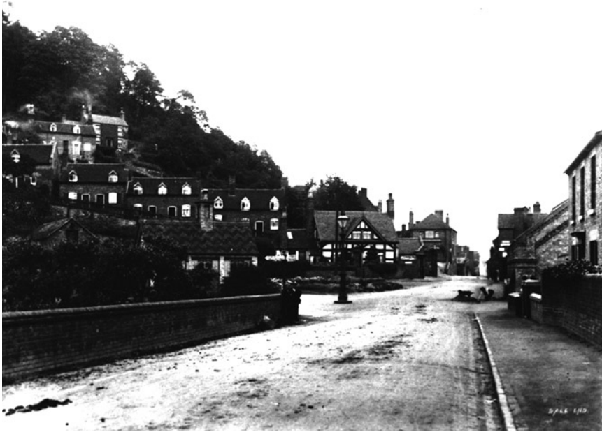
Fig 5.4 Old postcards can prove a useful source of historical, architectural, social and topographic information. (Photo: courtesy of Ironbridge Gorge Museum Trust)
