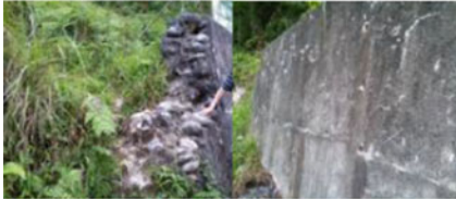
A roadside engineered structure, Mt. Apo, Kidapawan, Mindanao island, Philippines
