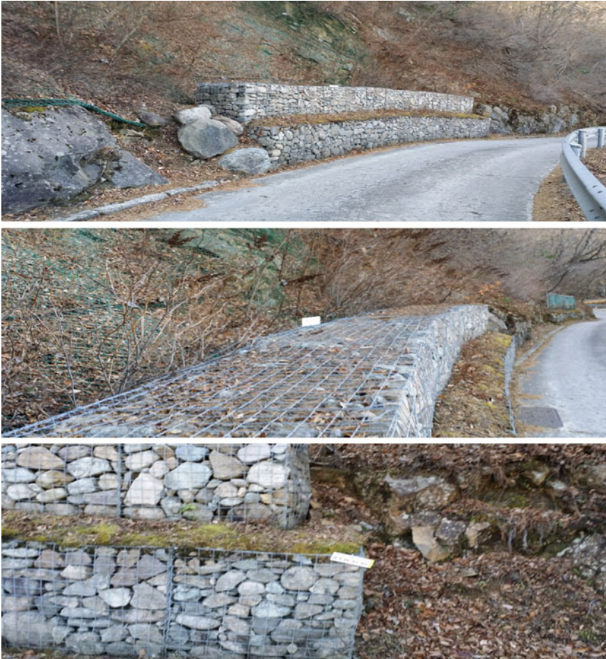
Fig. 4.33 Gabion walls to retain earth slopes on roadsides, Seoraksan National Park, Korea
