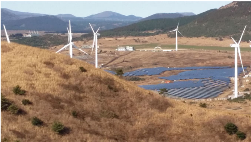
Fig. 3.51 Gasiri wind power generation complex, Jeju Island, Korea
