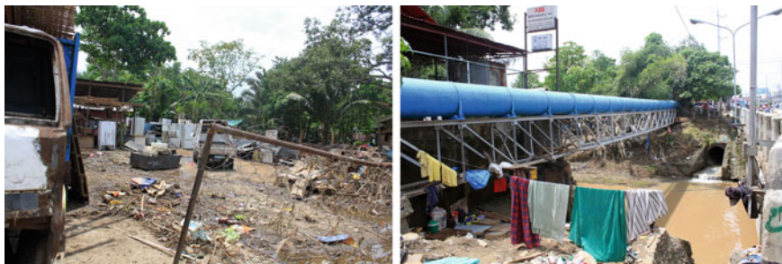
Fig. 4.6 Flood damage, Davao City, Mindanao, the Philippines
