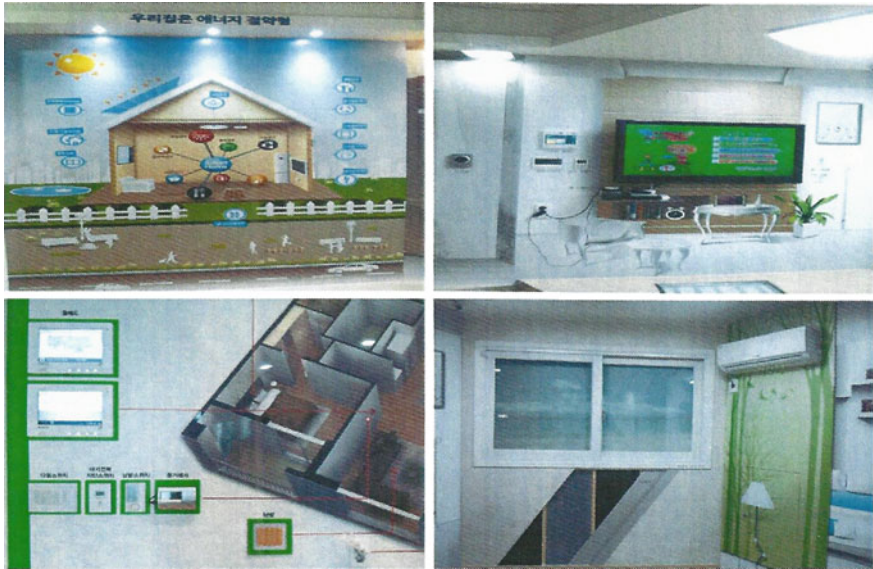
Fig. 3.48 Dispersal of room arrangements through overlay of new transfer technologies and new types of heat, electricity, and air-conditioning network, The Green, Korea Land and Housing Corporation
