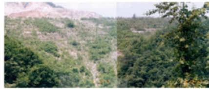
A restored area with the engineered structure and revegetation technique, Korea
