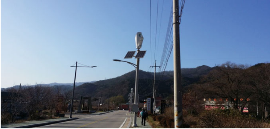
Fig. 6.2 Combined electricity generation of solar energy and wind power: hybrid system generated by natural energy, Seoraksan National Park, Korea
