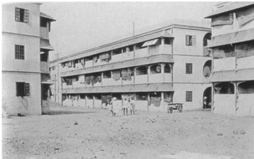
New-style chawls built by the Bombay Improvement Trust (about 1920). The plan was for one family to a room, with wide central corridors and through ventilation. (Source: Burnett-Hurst, 1925)
