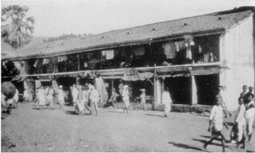
Two-storied chawl with shops on the ground floor. (Source: Burnett-Hurst, 1925)
