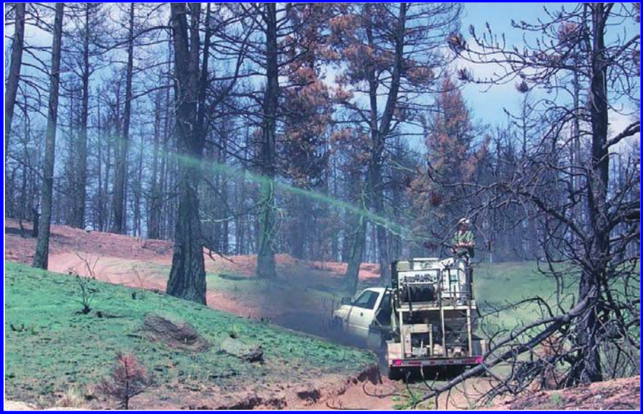
Fig. 5 Ground-based hydromulching on high soil burn severity area near a road after the 2002 Hayman Fire in Colorado, USA.
