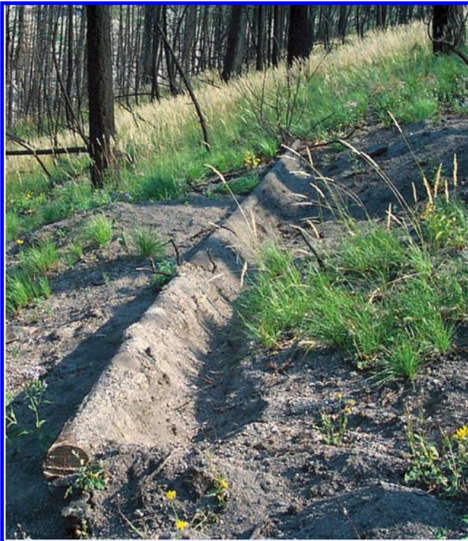
Fig. 1 A contour-felled log erosion barrier with soil end berms to increase storage capacity.
