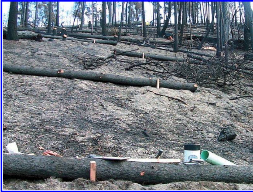
Fig. 7 Contour-felled logs installed in staggered tiers across a burned slope.
