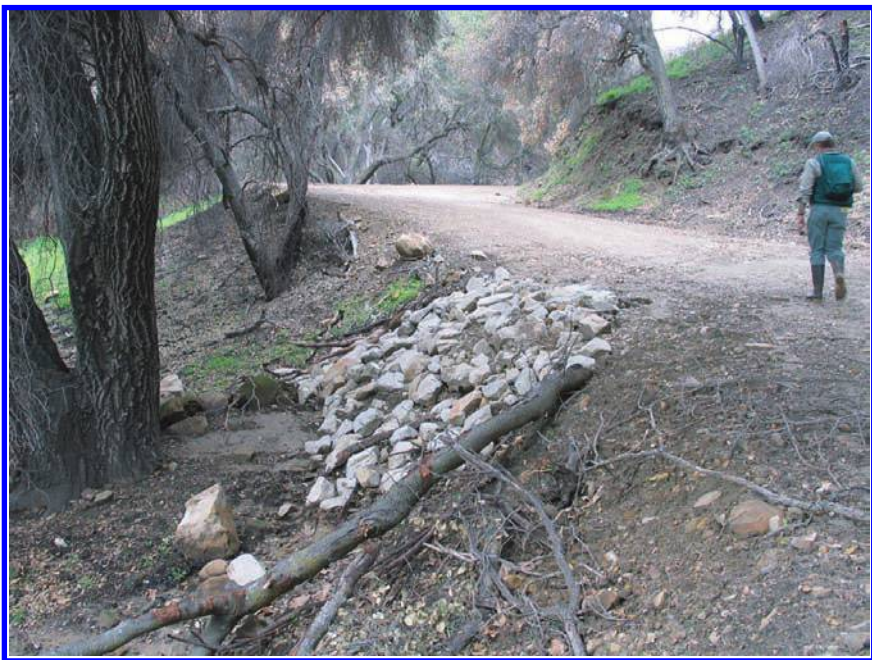
Fig. 2 Armoring of a fill slope on a forest road installed after the 2003 Piru Fire in southern California, USA.
