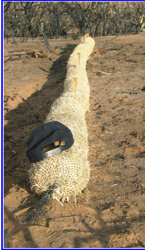
Fig. 2 A straw wattle erosion barrier.
