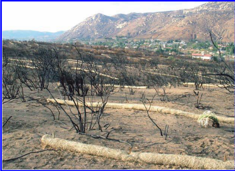
Fig. 8 Straw wattles installed in staggered tiers across a burned hillslope of chaparral.
