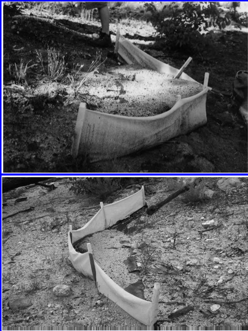
Fig. 2 Upper: Overflowing silt fence in the landscape north of Omeo, from Hobgen (2005). Lower: silt fence in the same area (photo taken September 2006), showing the absence of ground cover more than three years post-fire.
