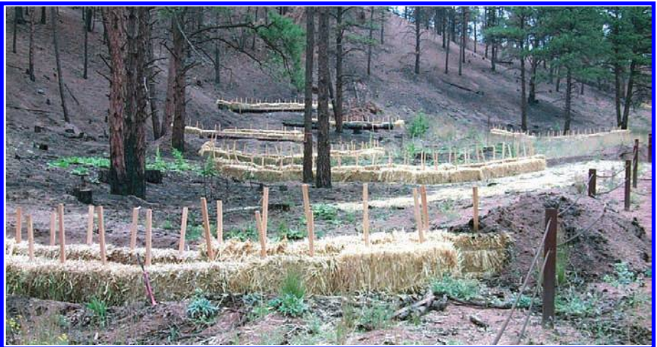
Fig. 3 Straw bale erosion barriers installed in a swale.
