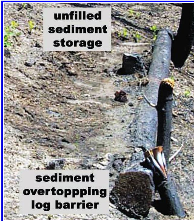
Fig. 10 Sediment over-topped this partially filled contour-felled log without filling the unused portions of the sediment storage basin.
