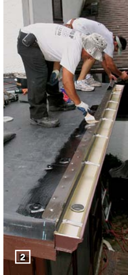
NAIL, THEN PRIME. Fasten the edge metal with 1½-in. galvanized roofing nails, wipe the edge metal and EPDM with membrane cleaner, and prime with EPDM primer.
