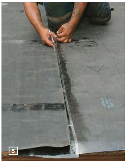
TRIM TO FIT. Heavy-duty scissors are the best tool for cutting EPDM membrane.
