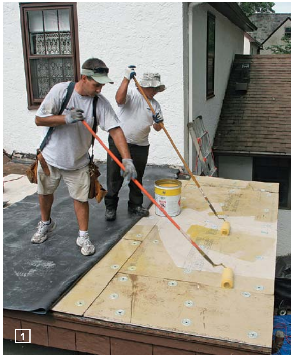
SPREAD THE ADHESIVE. Adhesive is rolled onto the gypsum board sheathing and the EPDM membrane.
