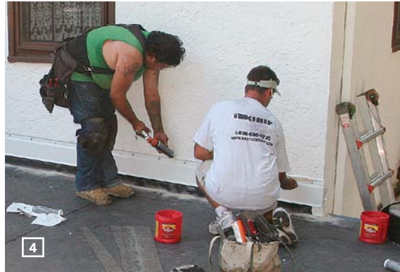
TERMINATION BAR IS FIRST. An extruded aluminum termination bar holds the kick and coats the top edge.
