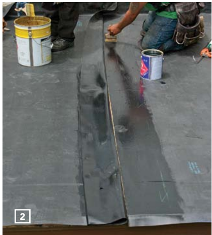
PREPARE SEAMS WITH PRIMER. Primer boosts the seam tape's adhesion.
