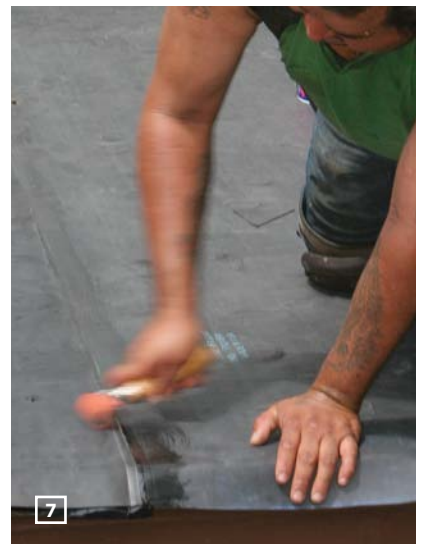
ROLL AGAIN. To activate the pressure-sensitive adhesive, it's important for every bit of seam tape to be rolled.
