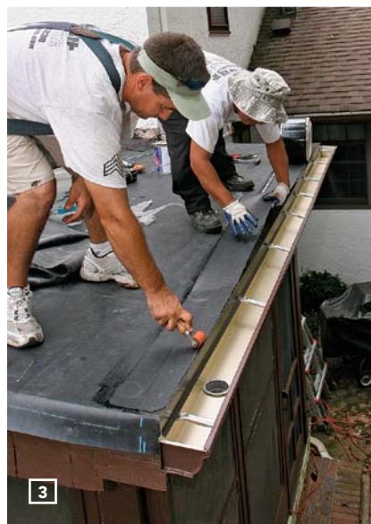
TAPE SEALS THE DEAL. To seal the metal edge, peel-and-stick cured flashing tape is applied and rolled in to activate.
