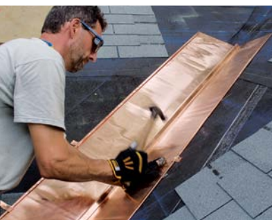
TWO WAYS OF HOLDING DOWN THE LINER. To allow the liner to expand lengthwise, fasteners cannot be driven through the liner. Instead, nails can be driven snug along the edge of the liner (right), or simple clips can engage a hem along the edge (left).
