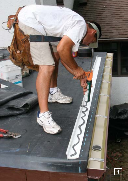
OVER, NOT UNDER. Drip edge goes over EPDM membrane.
