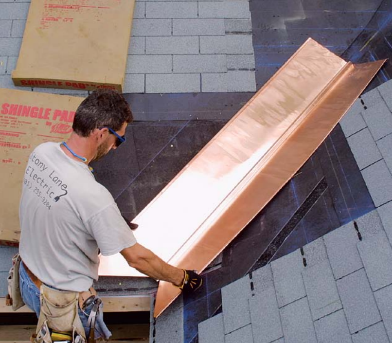
AN EXTRA CRIMP FOR EXTRA PROTECTION. An inverted V in the center of the valley liner helps to channel water down the valley while allowing for expansion and contraction widthwise.
