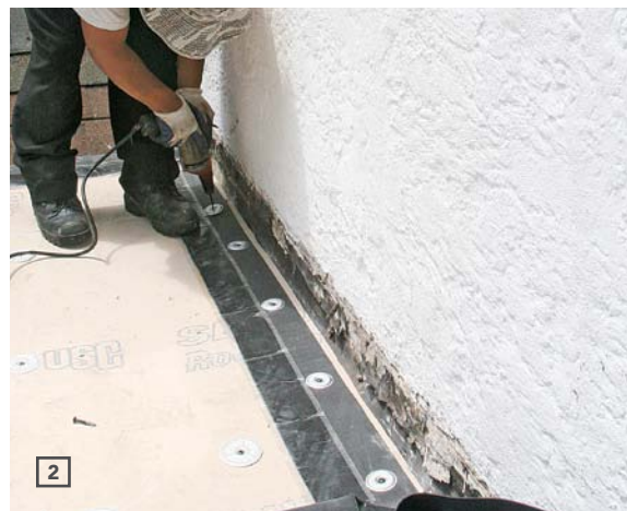
CONTROL EXPANSION AND CONTRACTION. To prevent the membrane from pulling away from the base of the walls, install a membrane-attachment strip.
