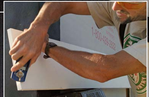
45° scarf joint on rake board
