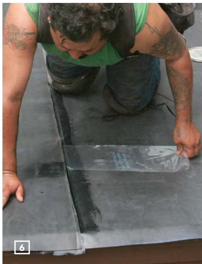
REMOVE THE RELEASE FILM by slowly pulling it away from the seam at a 45° to 90° angle.
