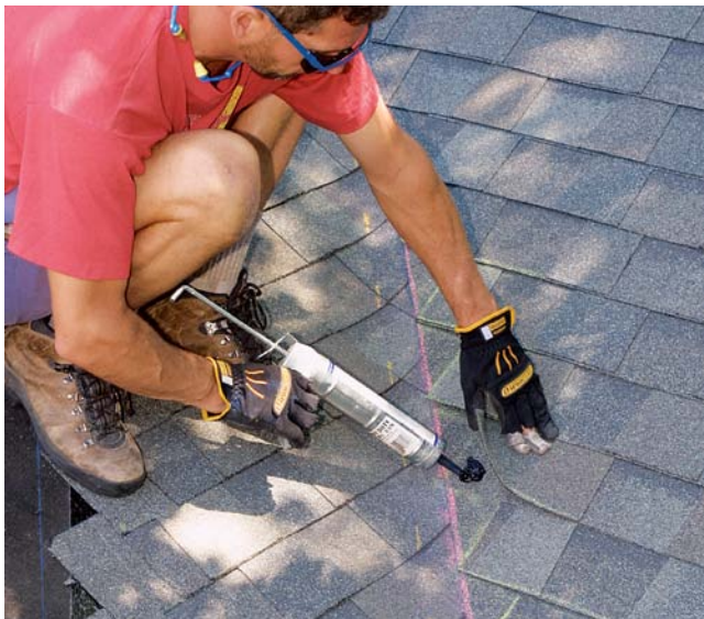
MINIMAL SEALING. A small dab of roof cement seals each shingle corner.
