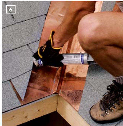
A CONTROLLED DOUBLE BEAD. For a quick and easy double bead of sealer, run the first bead with the nozzle of the gun inserted all the way under the shingles (left). A finger on the nozzle spaces the second bead (center), and the beads continue on the top lap of each shingle to complete the seal (right).
