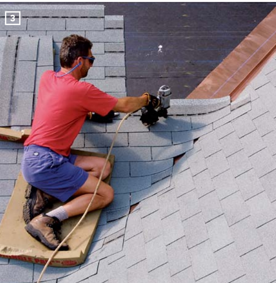
NAIL NOW, CUT LATER. A second way to install the shingles in an open valley is to run them long through the valley (left). Then, after snapping a cutline, trim the shingles with a hook blade in a utility knife, using sheet metal to protect the valley liner (right).
