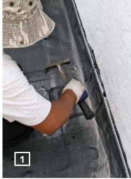
TERMINATION BAR IS FIRST. An extruded aluminum termination bar holds the kick and coats the top edge.
