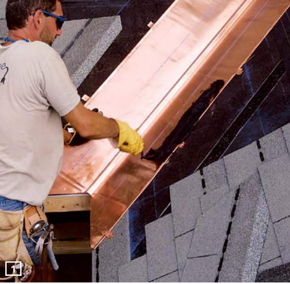
START SPREADIN' THE GOO. If you cut the shingles before nailing them in, spread a band of roof cement on the metal liner first (left). As each course goes on, the roof cement is spread on the top lap of each shingle as well (right).
