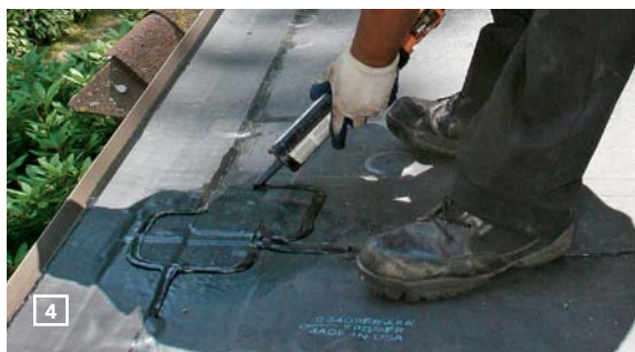
LAP CEMENT SEALS TAPE EDGES. Both sides of the flashing tape and any overlapping membrane should be sealed with EPDM lap caulk.
