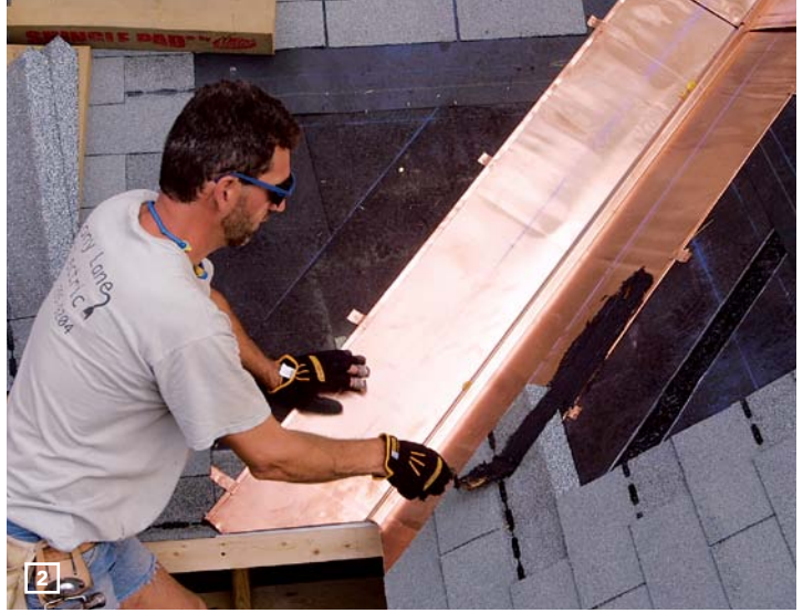
START SPREADIN' THE GOO. If you cut the shingles before nailing them in, spread a band of roof cement on the metal liner first (left). As each course goes on, the roof cement is spread on the top lap of each shingle as well (right).
