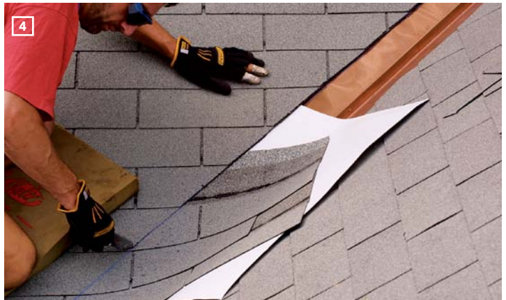
NAIL NOW, CUT LATER. A second way to install the shingles in an open valley is to run them long through the valley (left). Then, after snapping a cutline, trim the shingles with a hook blade in a utility knife, using sheet metal to protect the valley liner (right).
