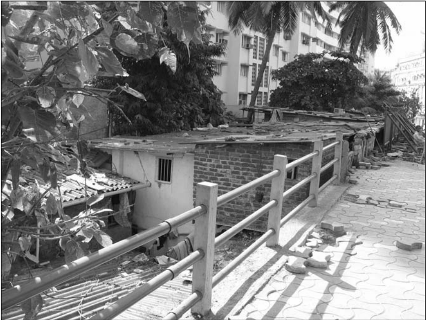
In Mumbai, slums attach, barnacle-like, to every high-rise building.
