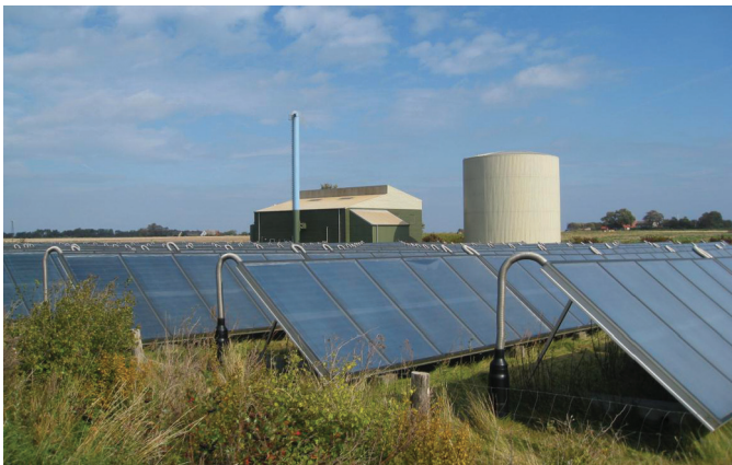
FIGURE 15.1 Solar panel used for heating. The district heating station is shown in the background.
