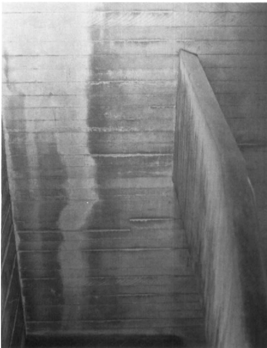
FIGURE 1.14 SOILING OF THE PARTIALLY SHIELDED EXTERNAL STAIRWAY OF THE NATIONAL THEATRE, LONDON
