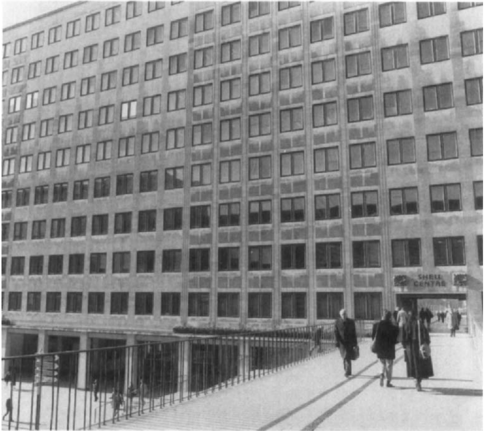
FIGURE 1.15 THE FACADE OF THE SHELL CENTRE IN LONDON, LAST CLEANED IN THE MID 1970s AND NOW SHOWING RENEWED SOILING
