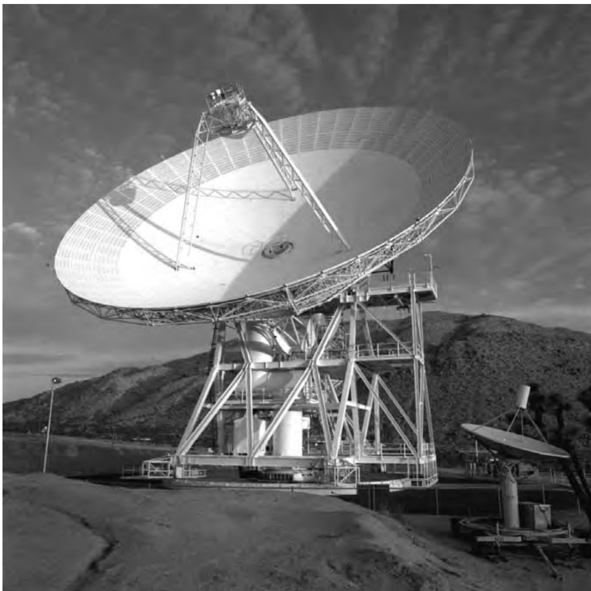
Figure 1.5. The Deep Space Network antenna at Goldstone, California (courtesy of NASA/JPL/Caltech, Pasadena, California). It can rotate with respect to azimuth (vertical) axis, and the dish with respect to elevation (horizontal axis).
